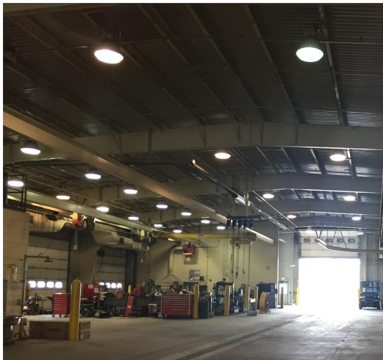
Figure 11 – Williams Garage Maintenance Area
