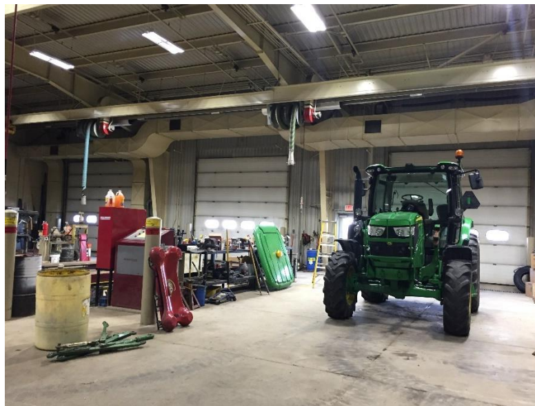
Figure 7 – Seneca Garage Maintenance Area
