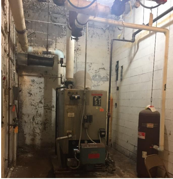
Figure 3 – 1987 Bryan Hot Water Boiler in Garage
