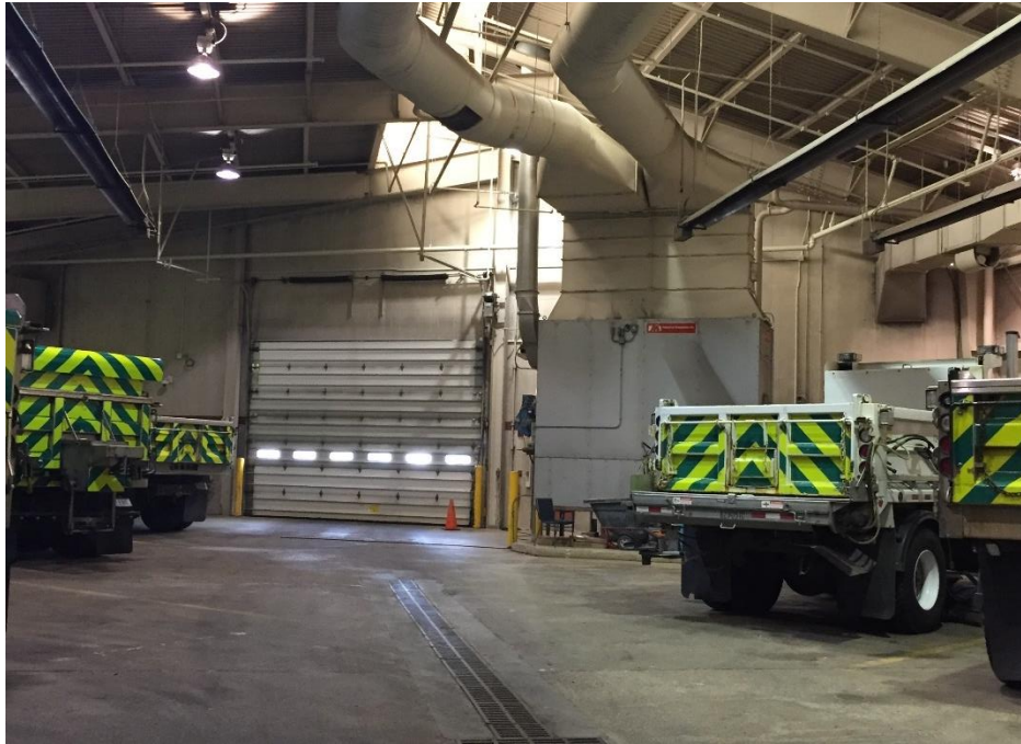
Figure 12 – Ottawa Garage Storage Area
