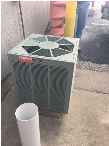
Figure 4 – 1999 Dayton Condensing Unit for Garage Offices
