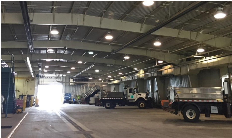
Figure 10 – Williams Garage Storage Area
