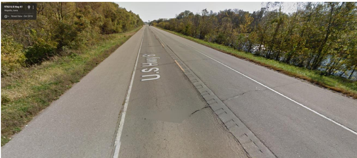
Figure 7. Centerline-only installation example
