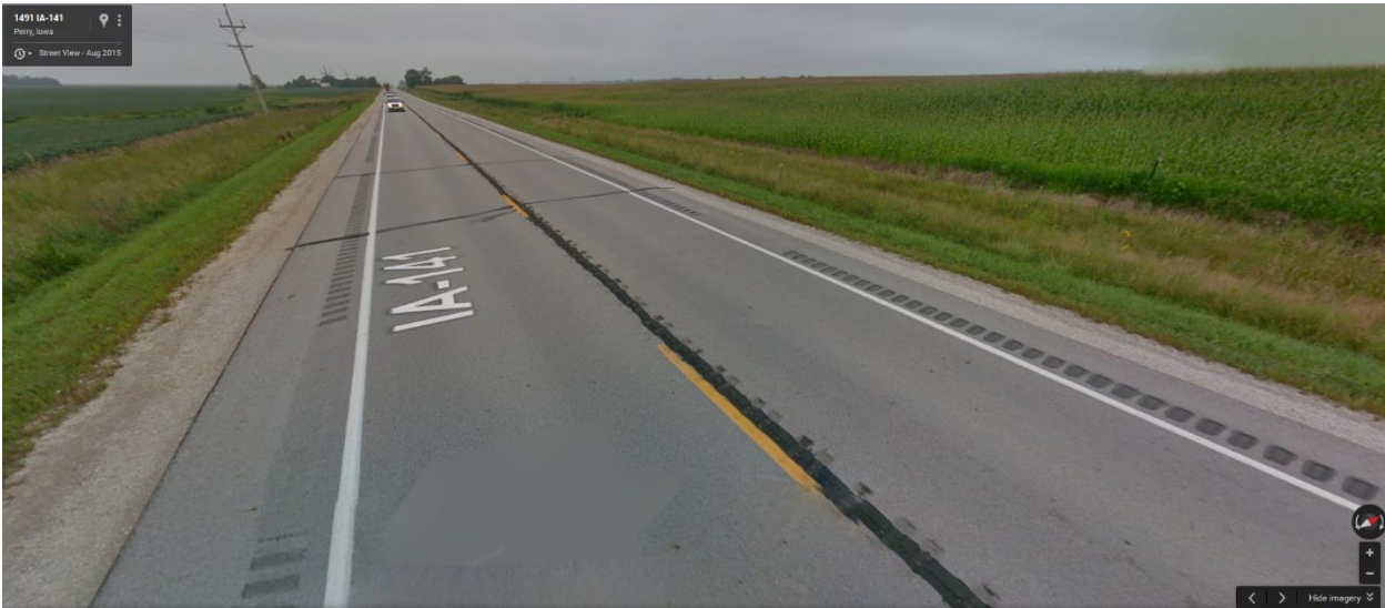
Figure 4. Continuous rumble strip installation with bicycle gaps
