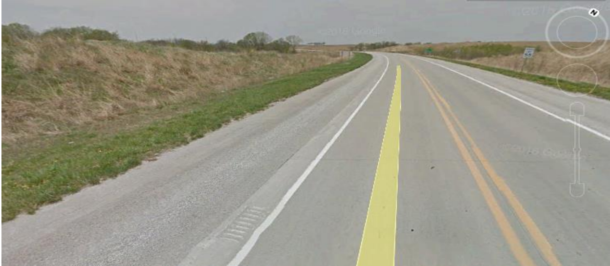
Figure 3. Intermittent rumble strip installation example
