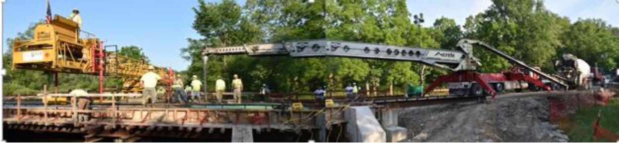
Figure H.13 Placement of Concrete into the Bridge Deck Formwork
