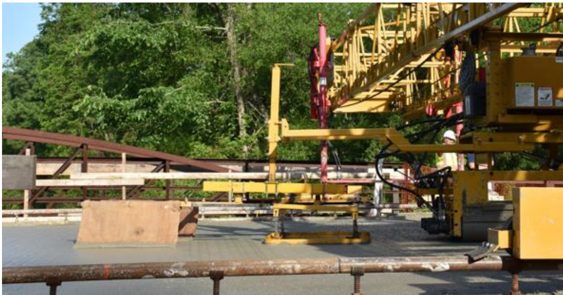
Figure H.14 Three-way Surface Finish Process Adopted for the Bridge Deck
