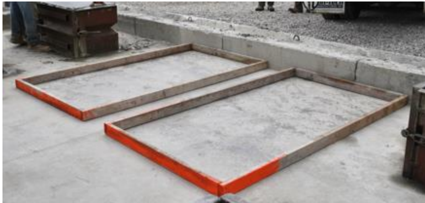
Figure H.3 Formwork for Trial Slabs
