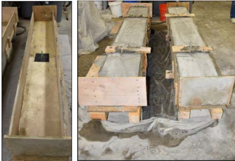
Figure G.17 Formwork and Casting of Slabs
