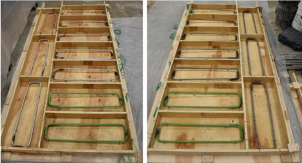
Figure D.3 Formwork for Test Slabs with Various Types of Rebar
