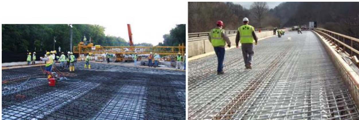
Figure A.62 Bridge with ASTM A1035 (left) and ASTM A955 Steel (right)
