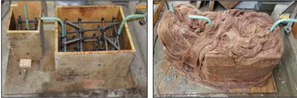
Figure G.16 Formwork for Column Showing Connection Type and Curing
