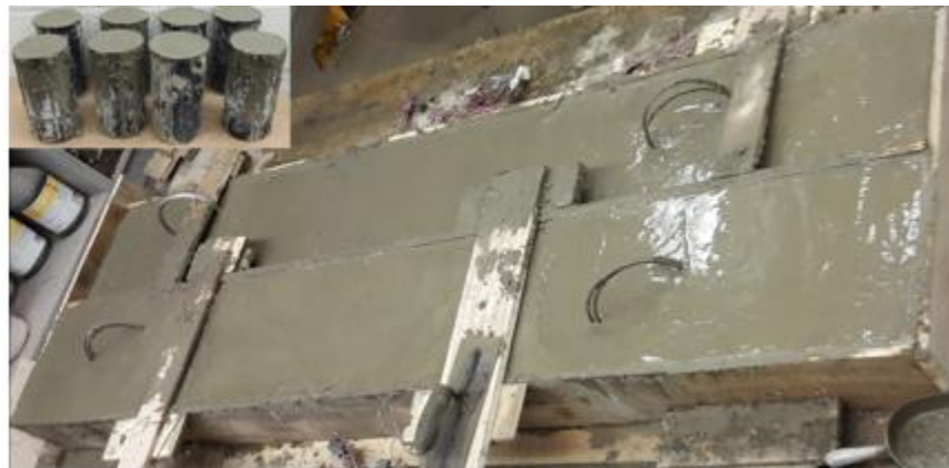
Figure F.47 Casting for Reduced-Scale Trial Slab Specimens
