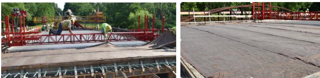
Figure H.16 Placement of Wet Burlap over the Bridge Deck
