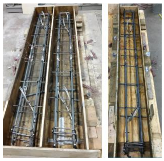
Figure F.46 Formwork and Reinforcement for Reduced-Scale Slab Specimens
