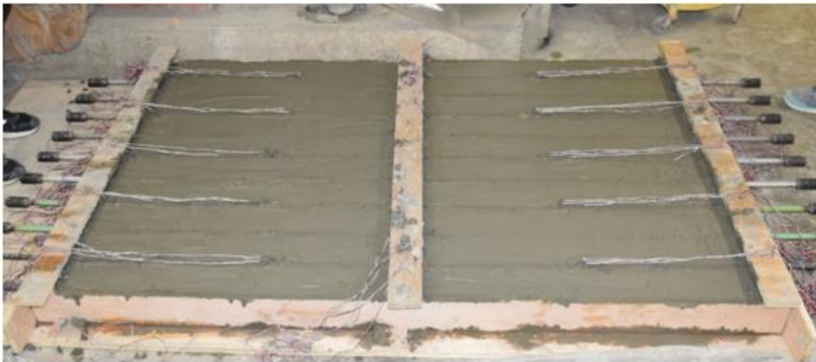
Figure F.20 Typical Casting of Long Specimens
