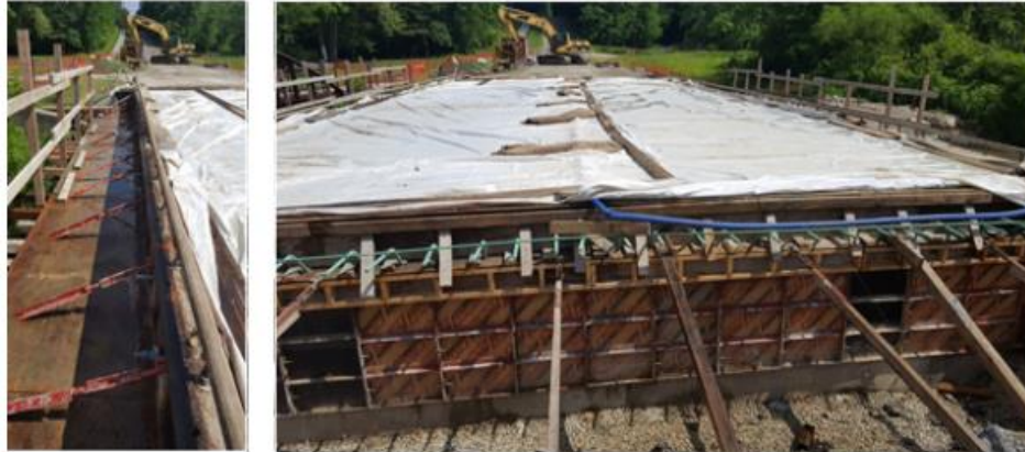
Figure H.17 Curing of the Bridge Deck
