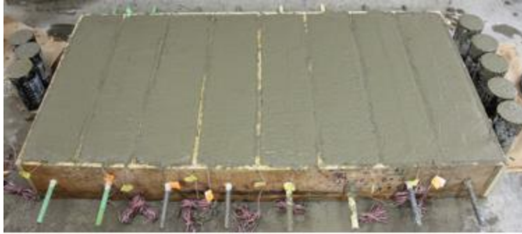
Figure F.8 Casting of 7'' × 7'' Specimens
