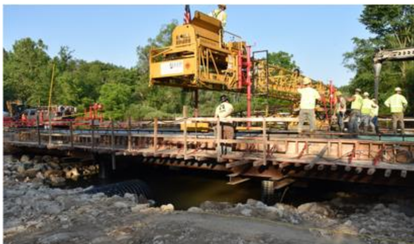
Figure H.9 The Selected Three-Span Bridge in Hinckley, Ohio
