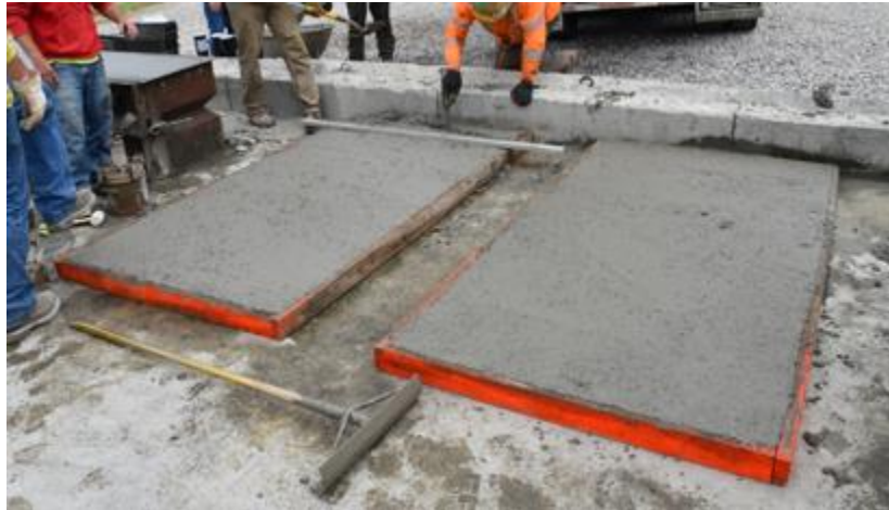
Figure H.8 Surface Finish of Slab 1 and Slab 2
