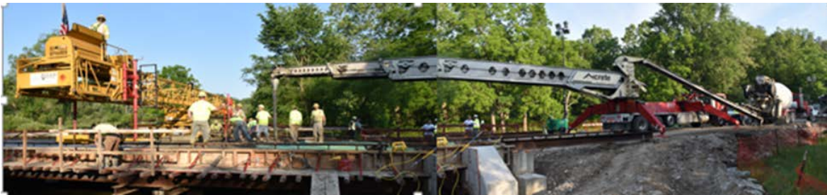
Fig. 16 General View of the Placement of Concrete
