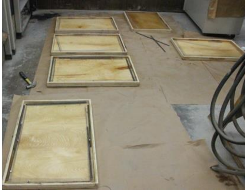
Figure E.10 Formwork for Test Panels
