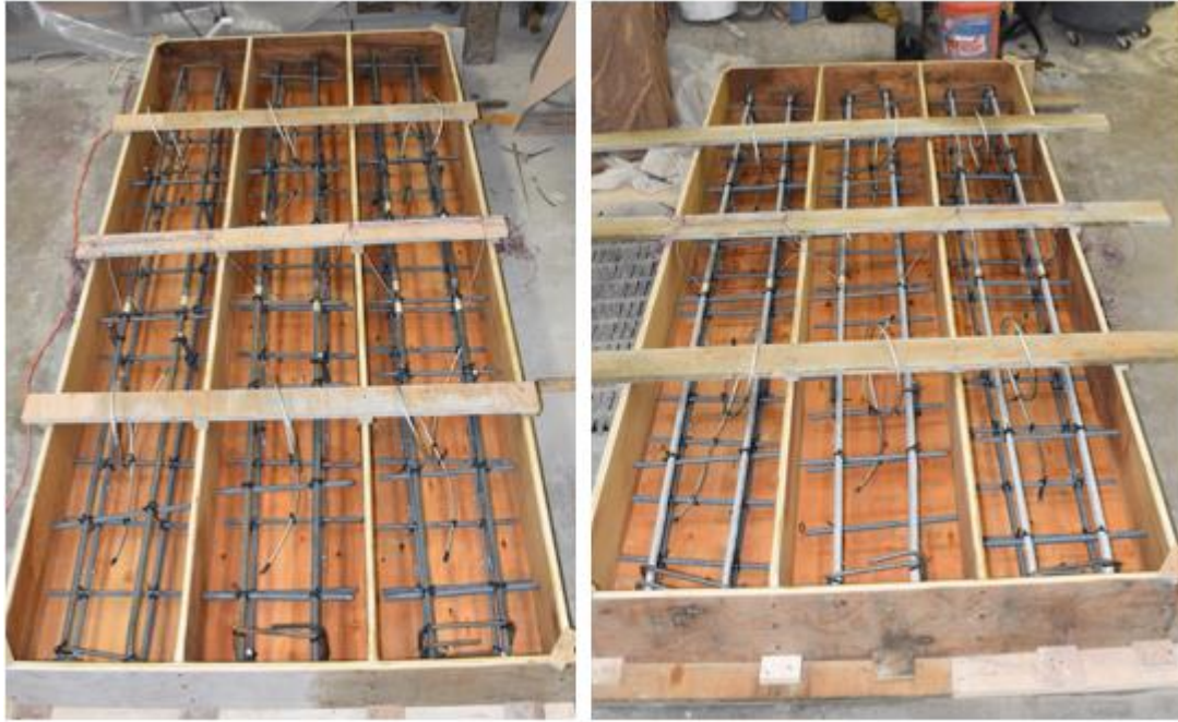
Figure F.55 Formwork Showing Black Bars ( Left ) and Stainless-Steel Bars ( Right )
