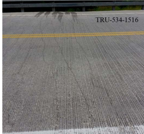
Fig. 2 Typical Structural Cracks over Pier Caps
