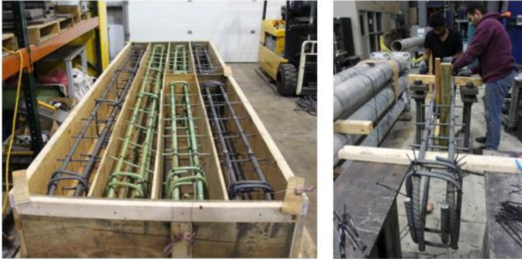
Figure F.34 Formwork and Reinforcing Cage for Slab Specimens
