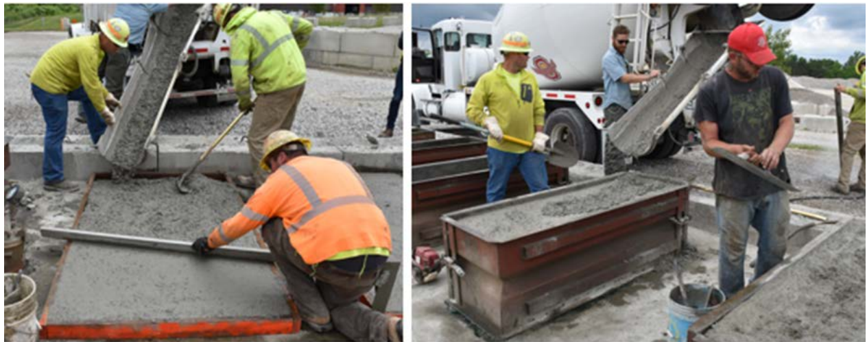
Fig. 15 Test Slab Placement at Osborne Test Site
