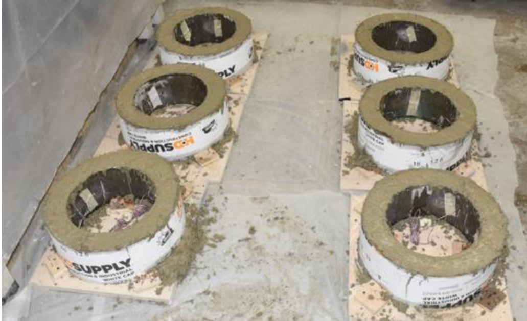
Figure E.23 Casting of Concrete Rings
