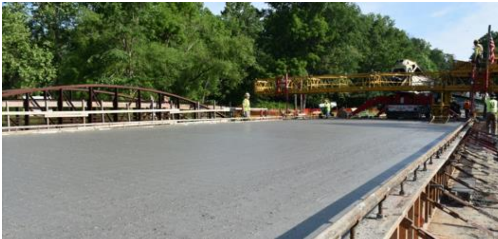
Figure H.15 Finished Surface of the Bridge Deck
