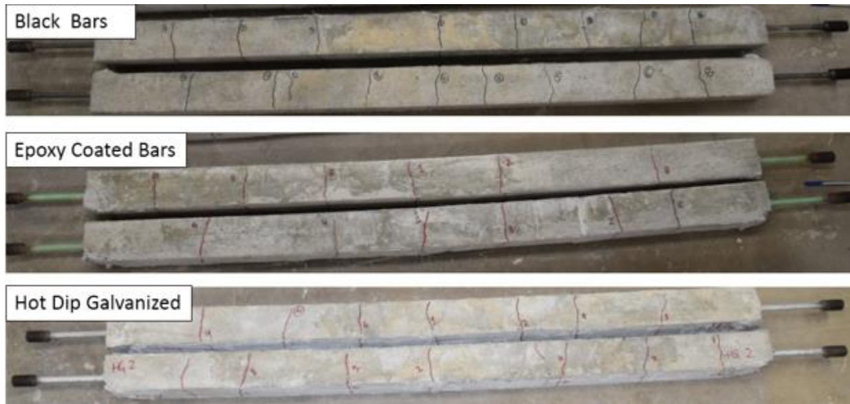
Figure F.27 Cracks on Prism Specimens without Fibers with Black, Epoxy-Coated and Hot-Dipped Galvanized Bars
