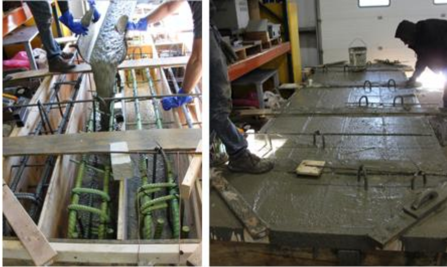
Figure F.35 Placing of Concrete into the Formwork
