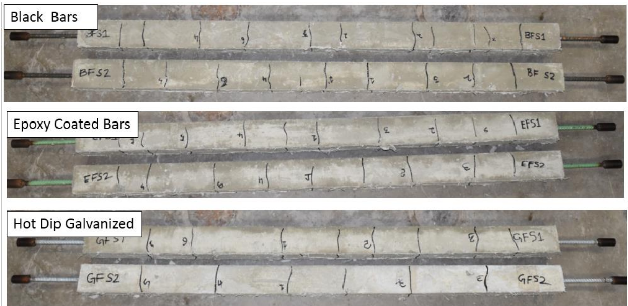
Figure F.29 Cracks on Prism Specimens with Fibers with Black, Epoxy-Coated and Hot-Dipped Galvanized Bars
