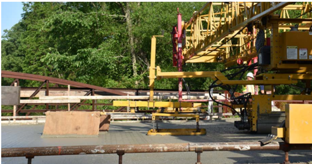
Fig. 17 Finishing of Concrete
