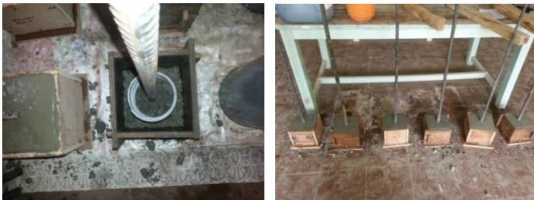
Figure A.36 Casting of Pullout Specimens (Deepthi and Sabeena, 2016)
