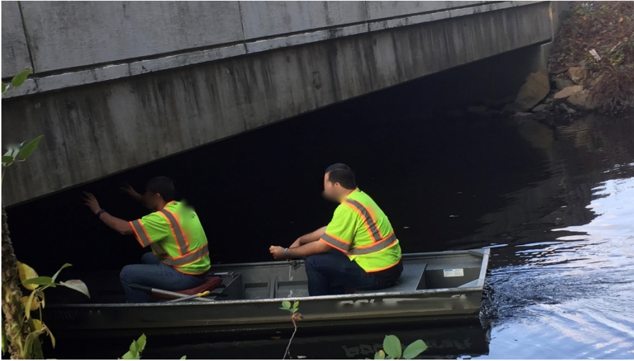
Figure D-1: Inspection of substructure elements of the bridge
