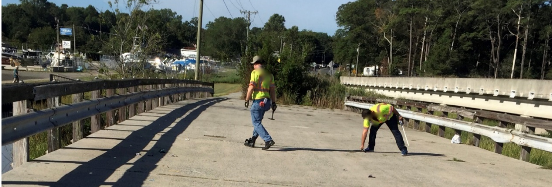
Figure C-3: Inspection of Bridge Elements
