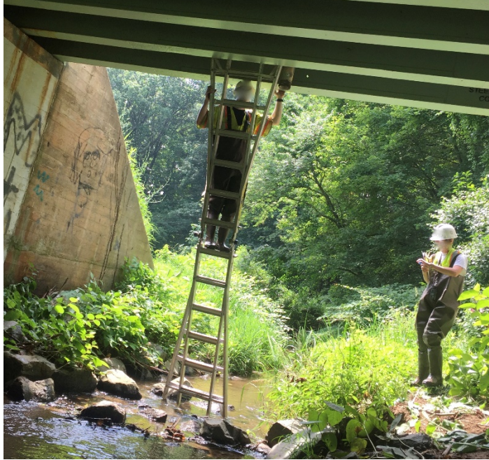
Figure D-3: Hands-on inspection of steel girders of the bridge
