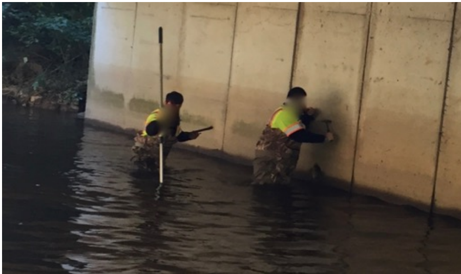
Figure D-2: Collecting scouring detail of creek
