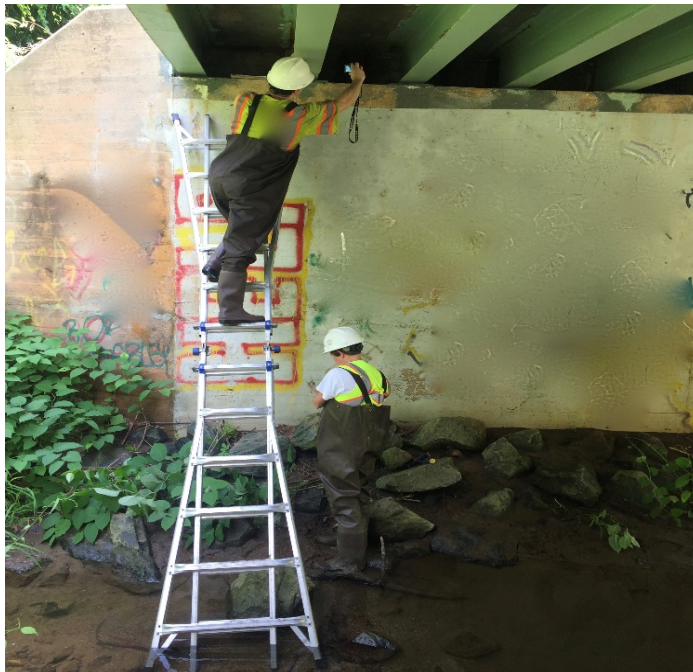
Figure D-4: Taking photos of fixed bearings of the bridge
