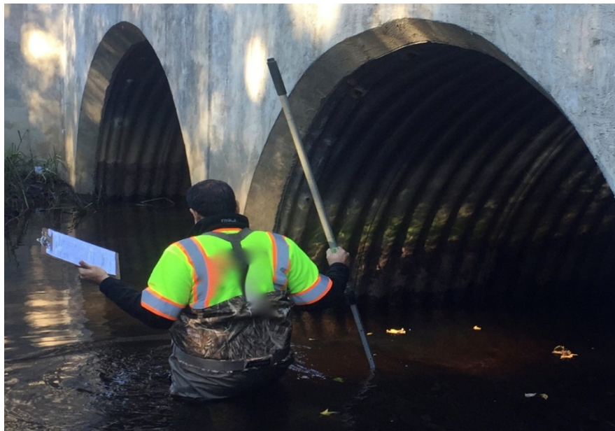
Figure 3.7: Inspector measuring scour detail of a channel
