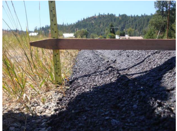
Figure 49. Close-up of edge treatment slope.
