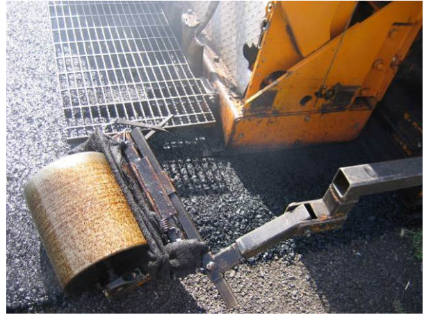
Figure 19. Close-up of roller hardware.
