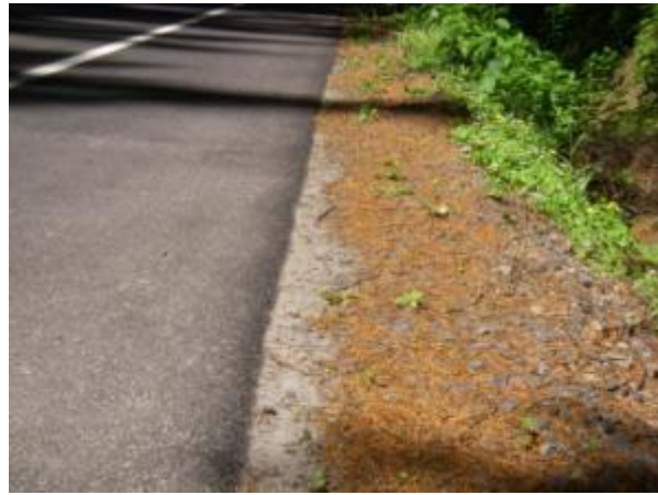
Figure 38. Pavement edge treatment on SR 410 one year after construction.
