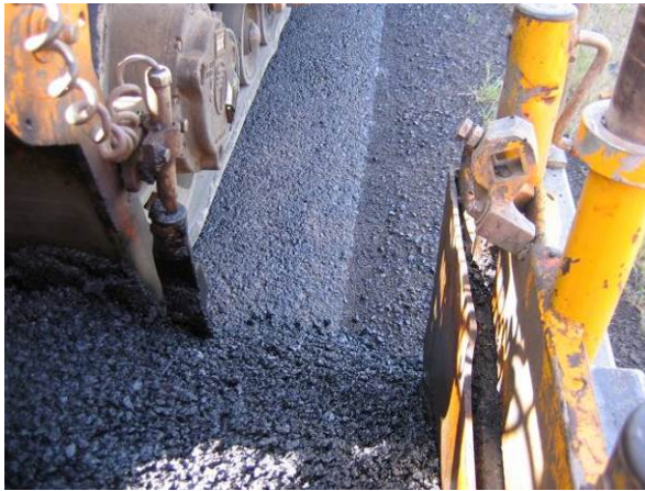
Figure 20. Close-up of sloped pavement edge showing top of slope at existing pavement edge.
