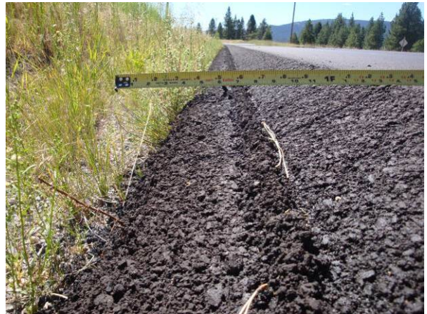
Figure 45. Close-up of edge treatment slope.
