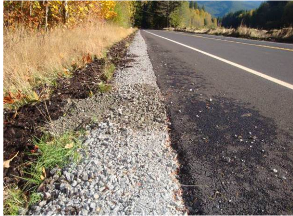
Figure 36. Shoulder material put back in place.
