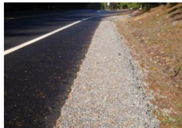
Figure 34. Finished pavement with dressed shoulders.
