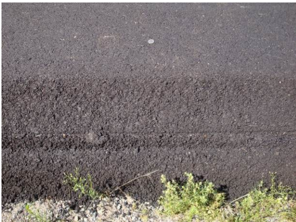
Figure 46. Side view of edge treatment.
