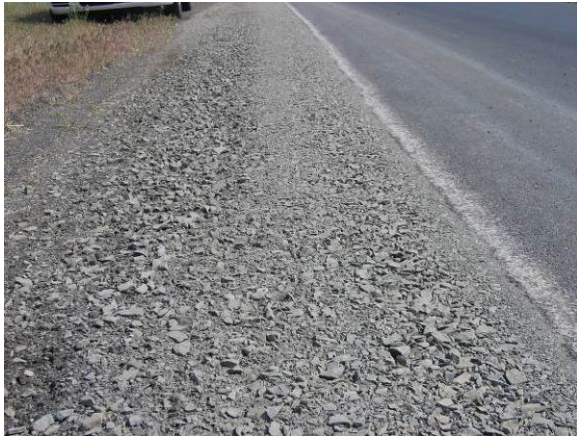
Figure 24. Finished pavement with shoulder material in place.
