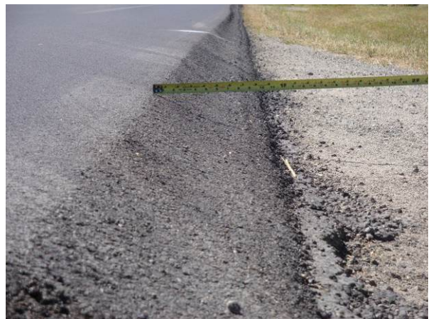
Figure 51. Closer view of slope of edge treatment.
