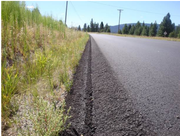
Figure 44. Pavement edge treatment on SR 21.
