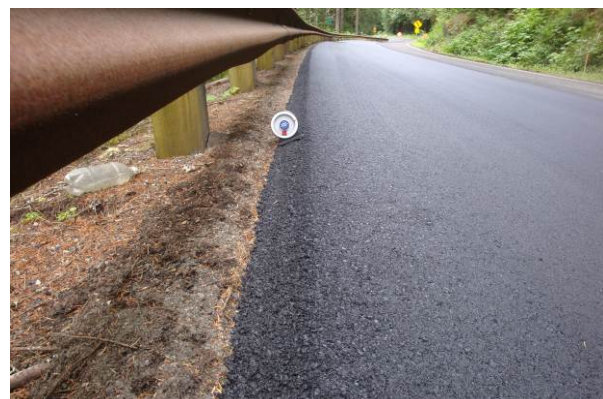
Figure 60. Pavement edge treatment next to guardrail.
