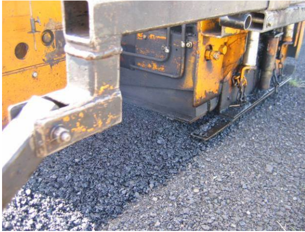
Figure 18. Close-up of paver screed.
