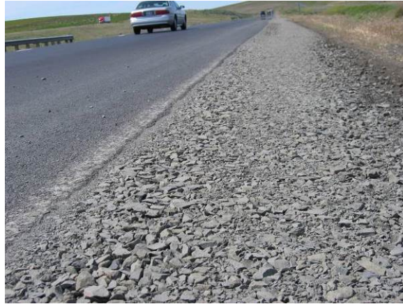
Figure 25. Finished pavement with shoulder material in place.
