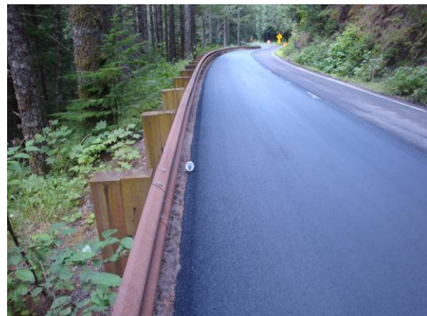
Figure 58. View showing uniform appearance of edge treatment.
