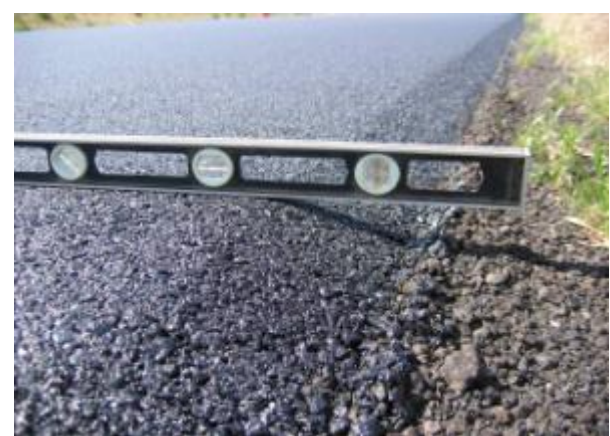
Figure 23. Angle of sloped pavement edge. Note the uniform compaction.
