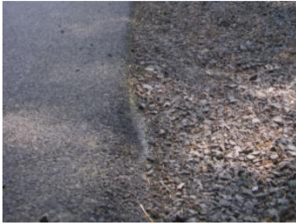
Figure 37. Pavement edge treatment close-up one year after construction.
