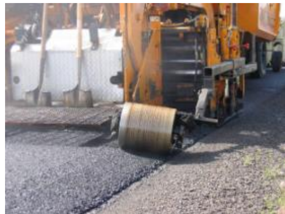
Figure 17. Paver forming and compacting pavement edge treatment.
