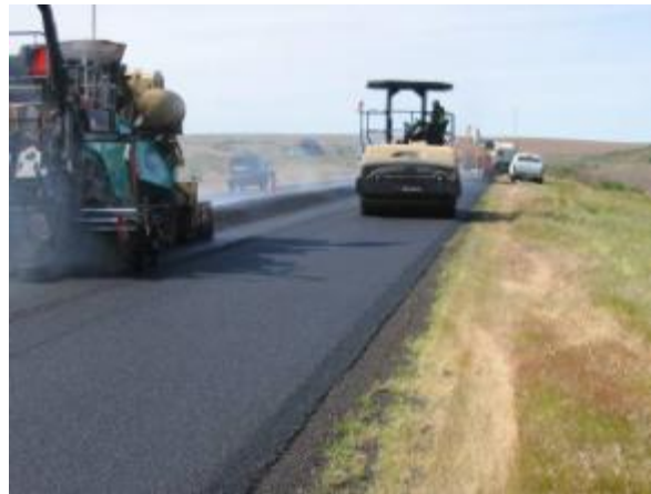
Figure 22. Distant view of paver with edge rolling hardware.
