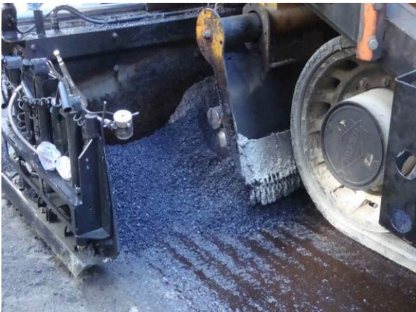
Figure 54. Mix passing through the end gate.
