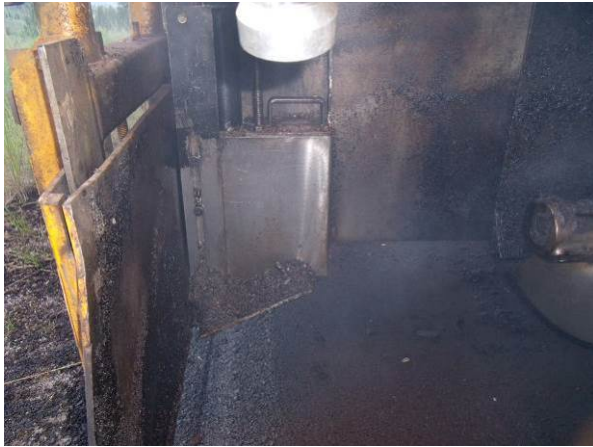
Figure 42. Advant-Edger™ used to produce the pavement edge treatment.
