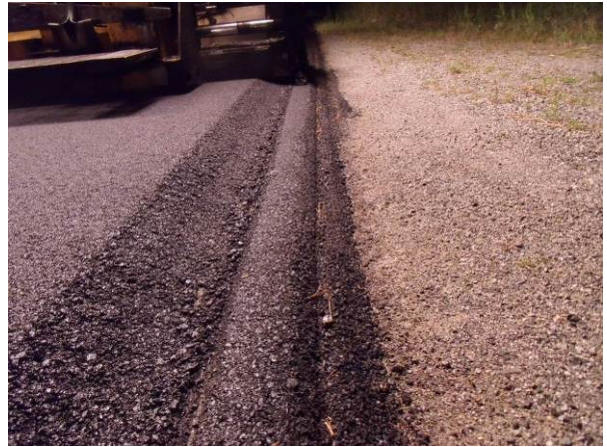
Figure 43. Pavement edge treatment produced by the Advant-Edger™.
