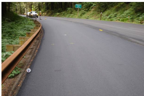
Figure 59. Pavement edge treatment next to guardrail.
