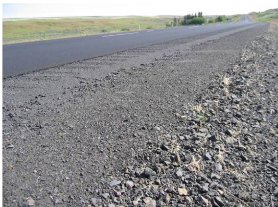
Figure 16. SR 395 before overlay. Note wide stable shoulder.
