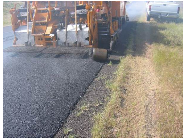
Figure 21. View of rolled pavement edge treatment.
