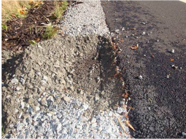
Figure 35. Dig out showing slope of pavement edge.
