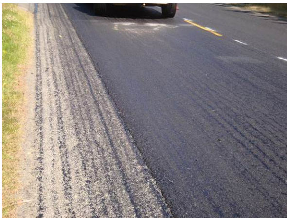
Figure 27. SR 410 prior to construction.
