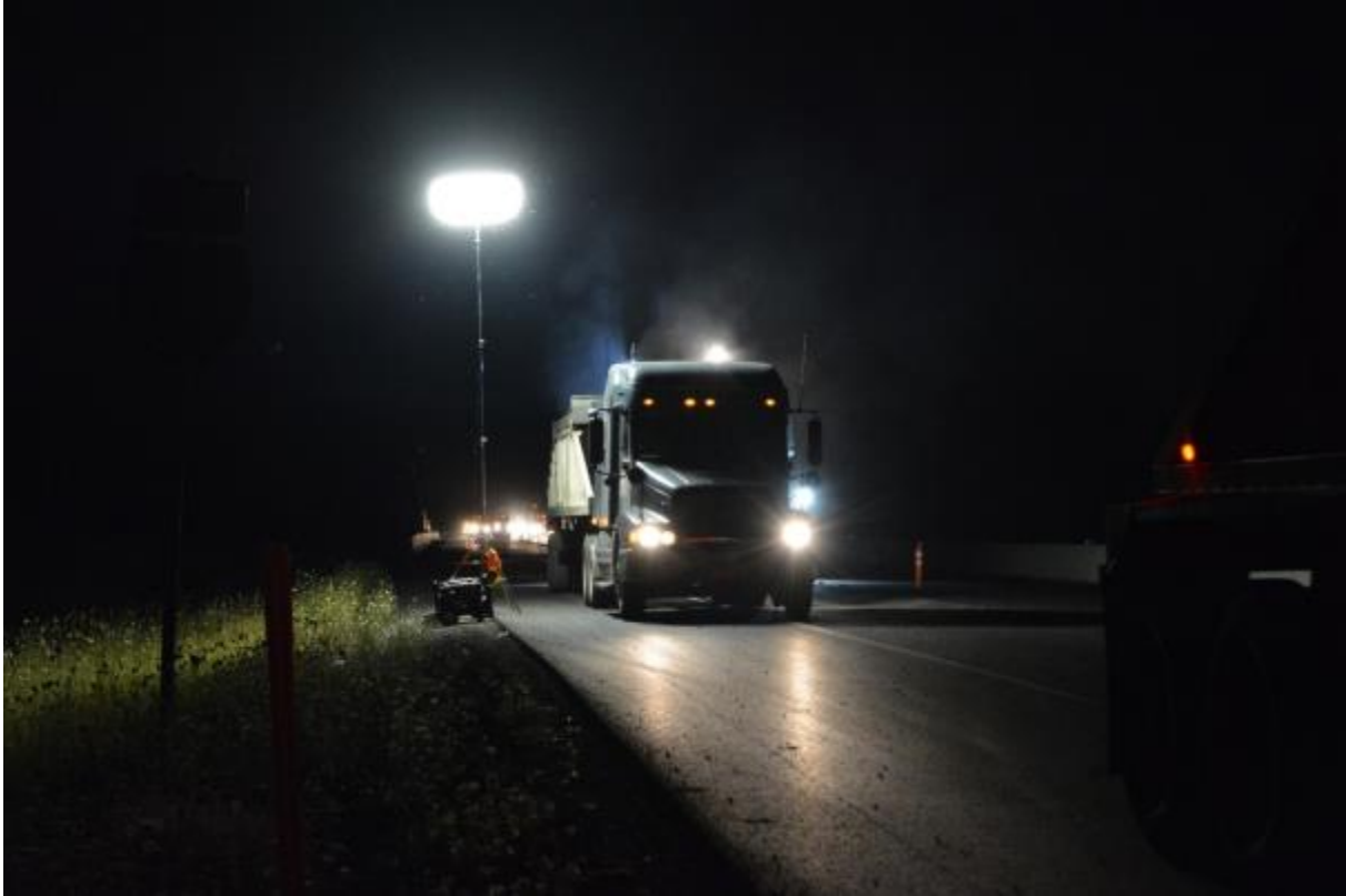
Figure 8.2: Balloon Light used on I-84 Jordan Road to Multnomah Falls (Case Study #1)
