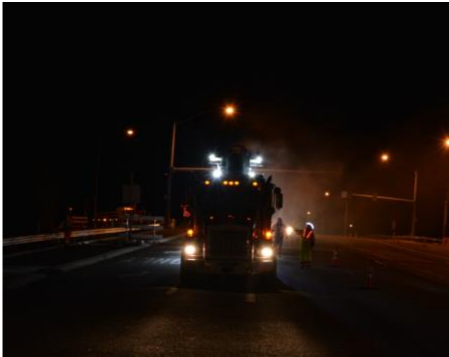
Figure 5.2: Spotter Working around Grinder and Dump Truck with Halo Light on Hard Hat and Flashing LED Vest
