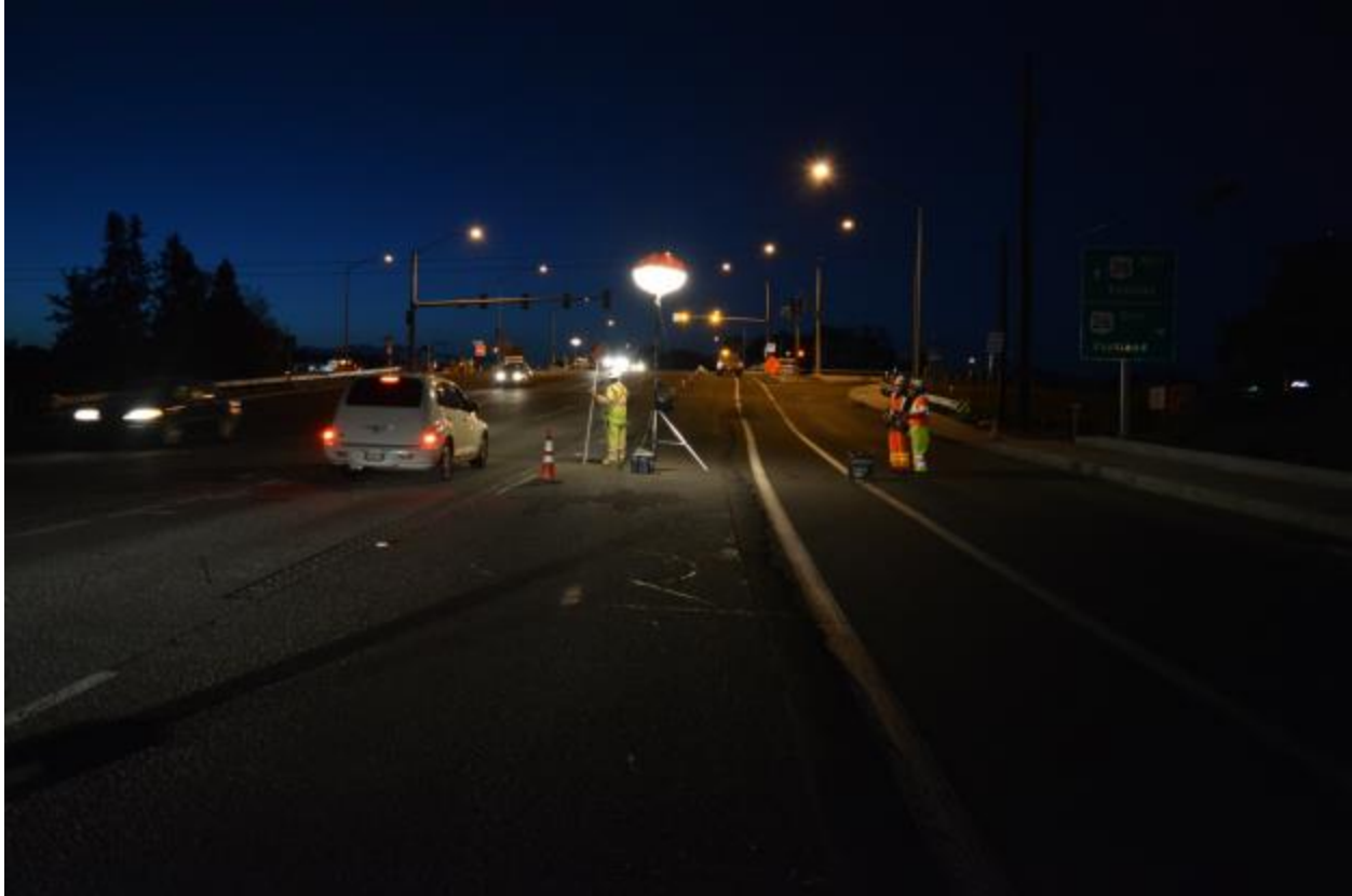
Figure 5.4: Flagger under Portable Balloon Light and Researchers within approximately 15 feet Distance from the Light
