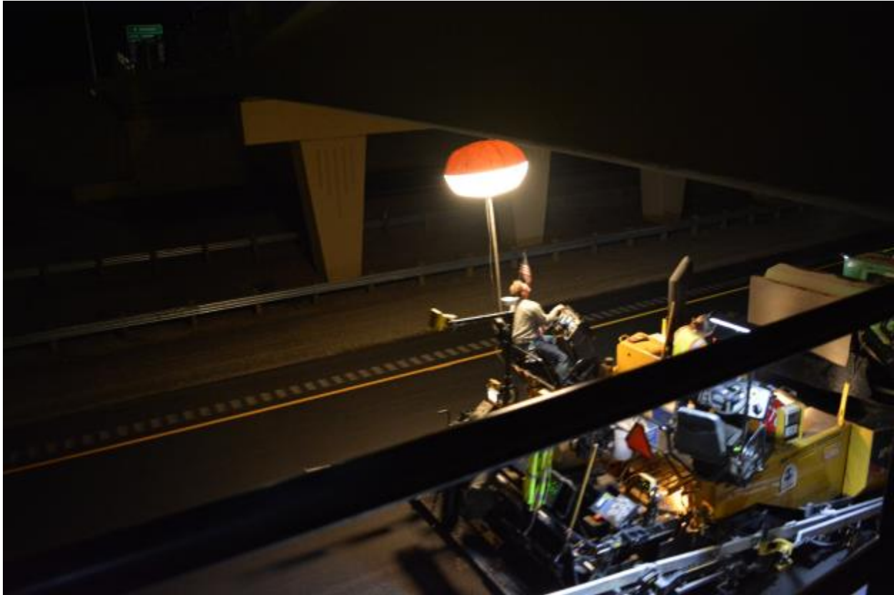
Figure 9.40: Paver Progress being Obstructed by Overpass due to Height of Balloon Light
