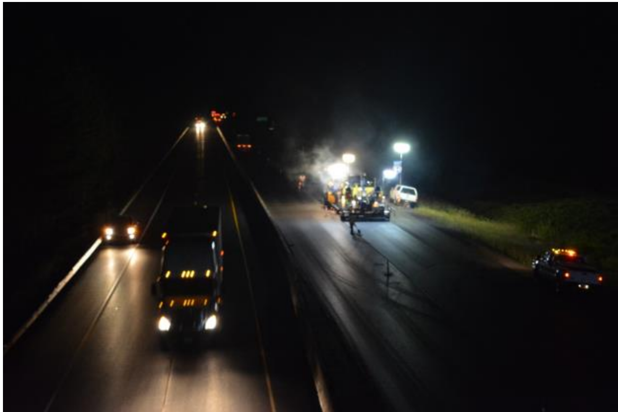
Figure 9.33: Visibility of Workers Upstream and Downstream of Light
