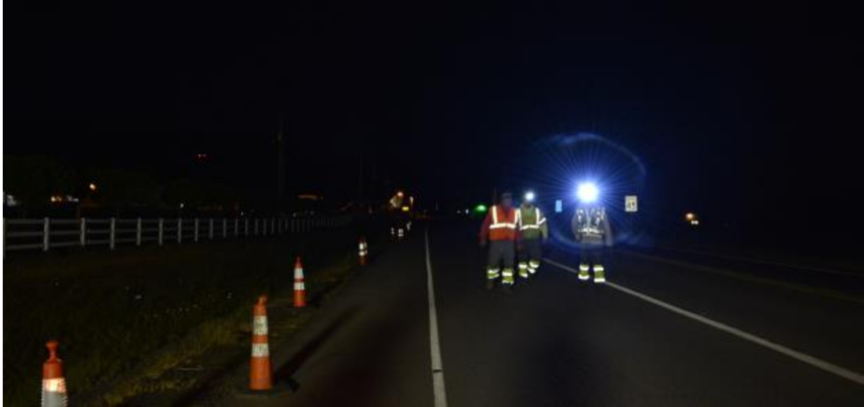
Figure 5.8: Workers Wearing High Visibility Apparel and Head Light
