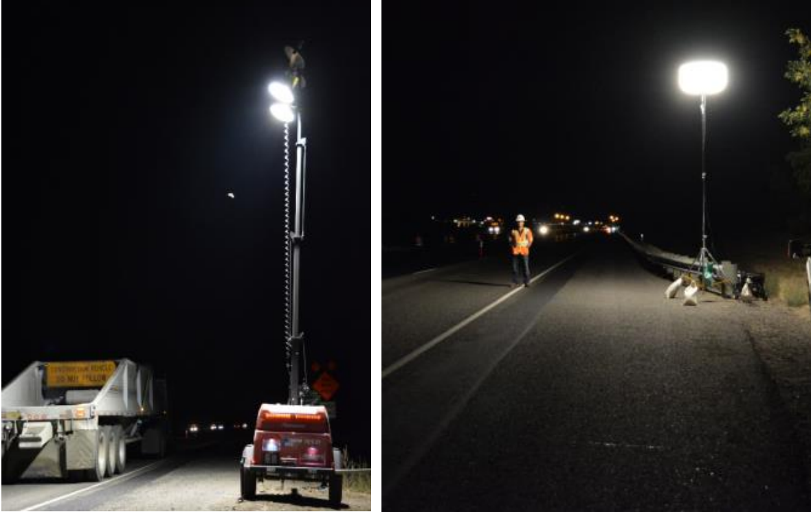
Figure 8.14: Lighting Equipment used for I-5 Medford to Ashland-(Case Study #2)
