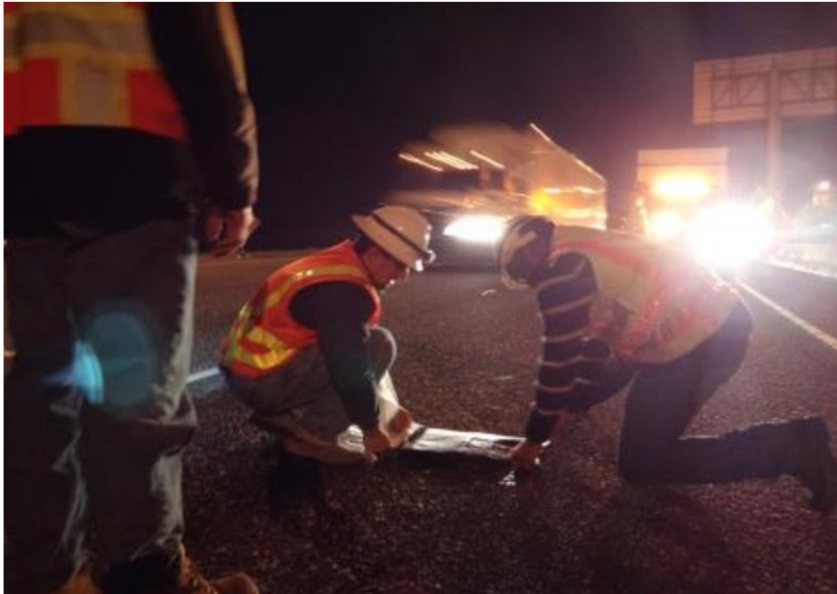
Figure 8.5: Placement of Portable Traffic Analyzer using Adhesive Tape (Gambatese and Jafarnejad, 2015)
