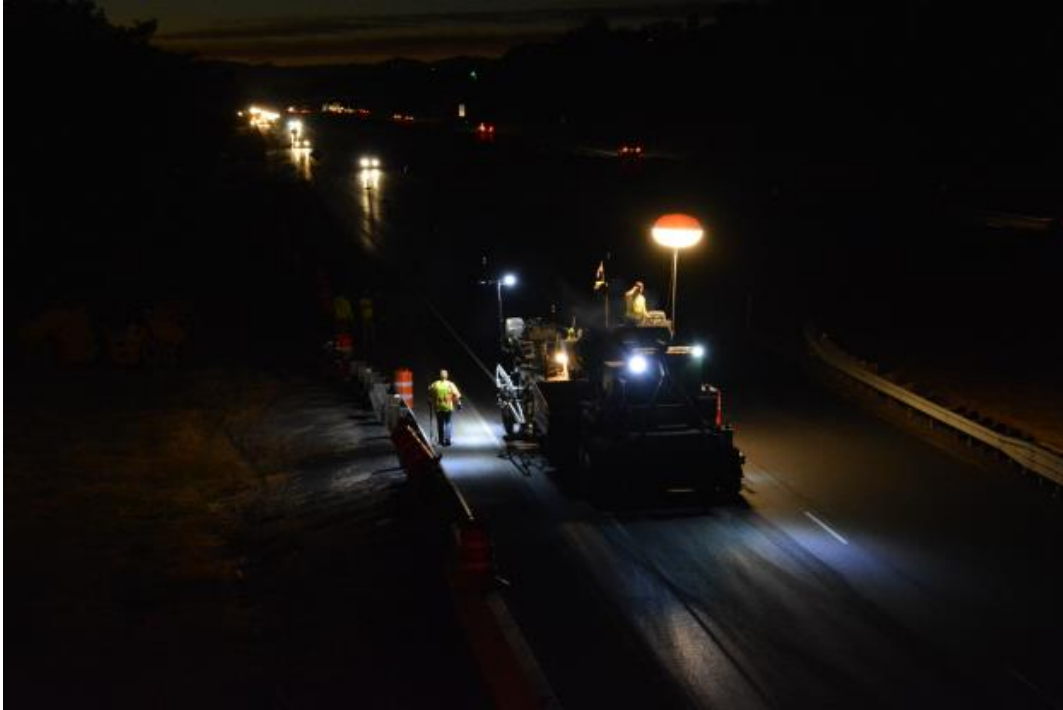
Figure 8.15: Paver Lighting, I-5 Medford to Ashland (Case Study #2)
