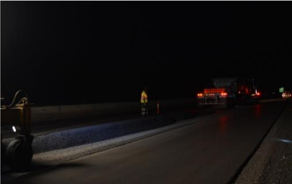
Figure 9.39: Visibility of Worker Wearing Clean Reflective Garments without Halo Light
