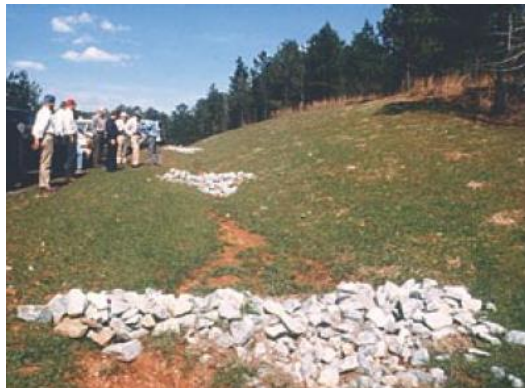
Figure 28. Picture of rock check dam placed inside roadside ditch (Tonning, 2007)
