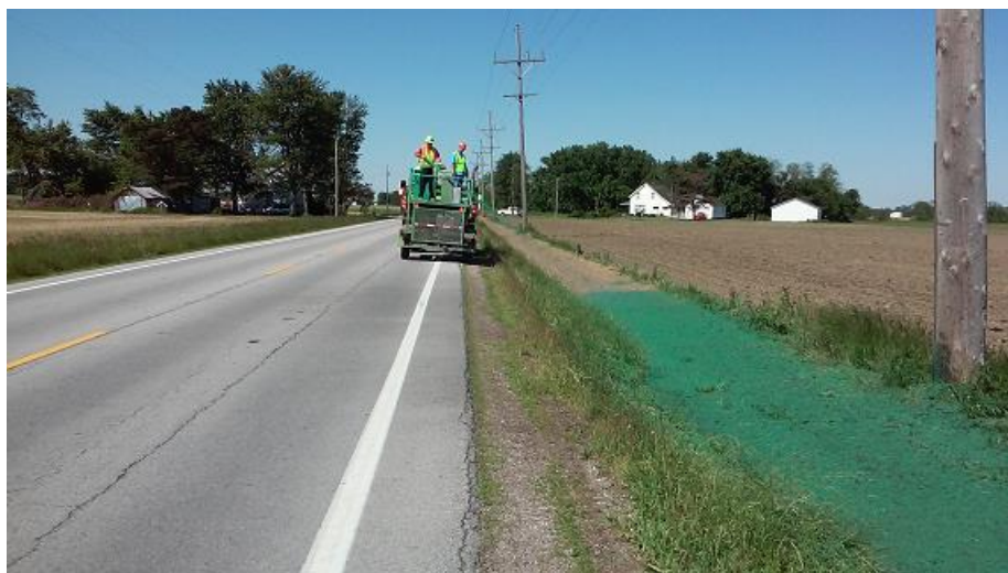
Figure 13- ODOT Crew applying hydraulic mulch to a ditch in Putnam County
