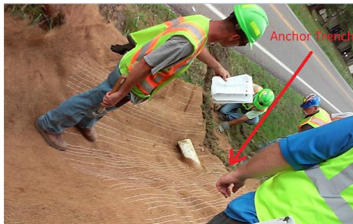
Figure 23. ODOT backfilling anchor trench with dirt
