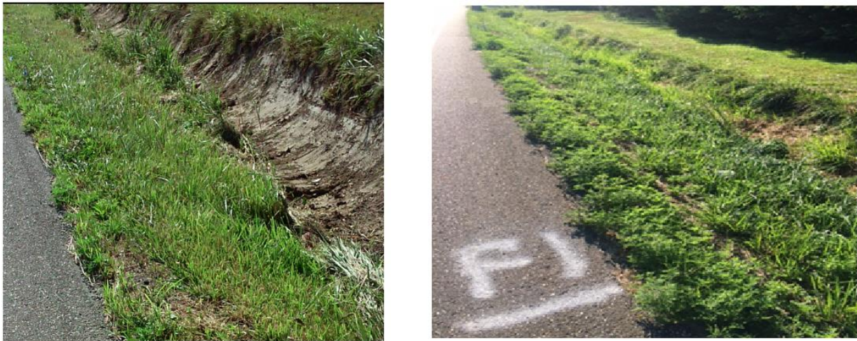
Figure 10-Roadside Ditch before and after permanent seeding
