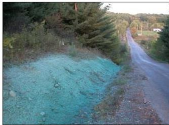
Figure 15. Ditch with a steep slope (Schneider 2014)
