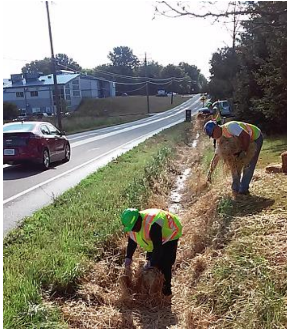
Figure 12- ODOT crew applying straw mulch to ditch after seeding it.
