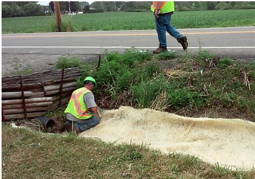
Figure 20. ODOT Crew installing a TECB in a ditch in Mahoning County
