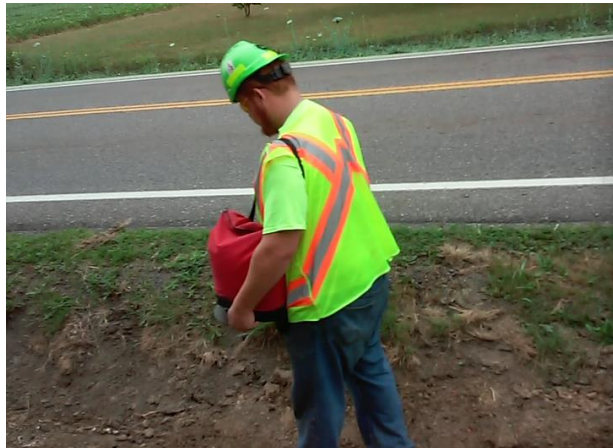
Figure 11. Manual Seeding using a Cyclone Seeder
