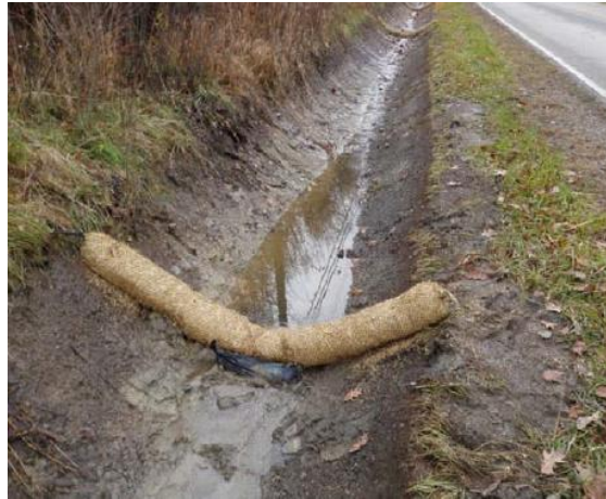
Figure 19. Picture of straw wattle placed inside a roadside ditch (Kitsap 2012)
