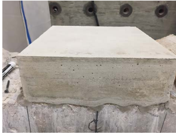
(b) Casting of grout block
