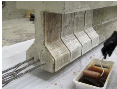
(e) Applying shear GFRP
