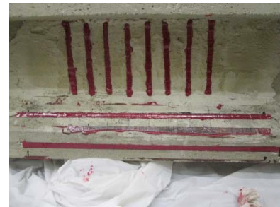
(f) Final repair after troweling and removing tape
