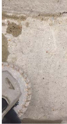
(a) Surface grinding
