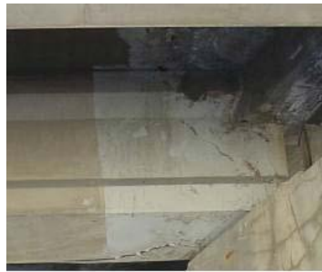
(b) Typical mortar repair of girder end
