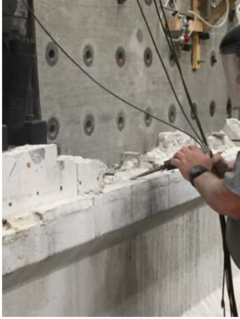
(a) Removal of uneven concrete
