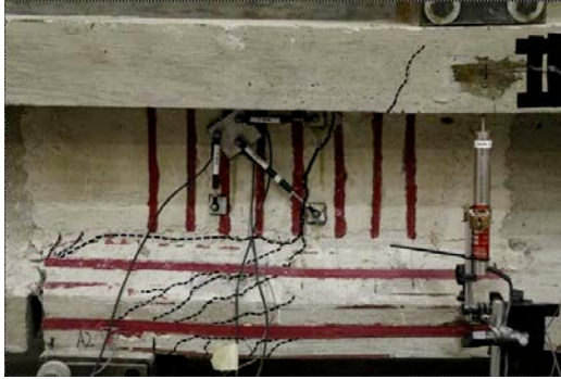
(a) Cracking pattern
