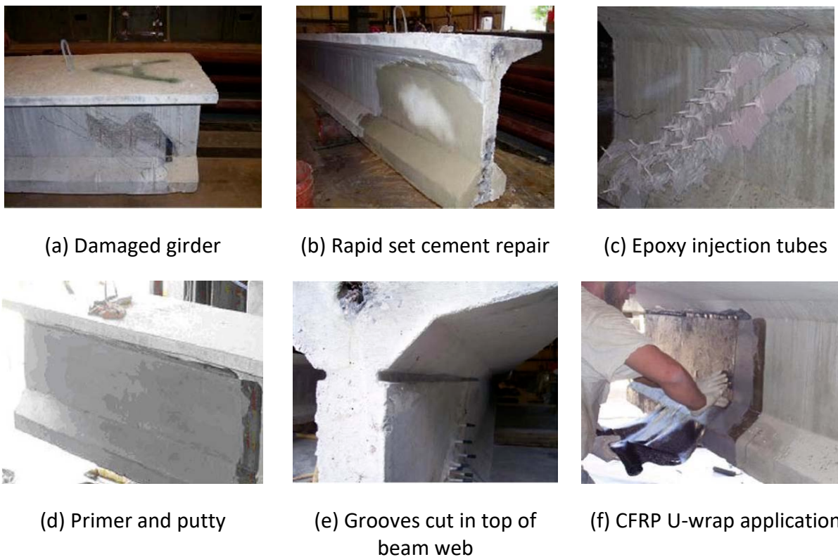
Figure 2.3. Post-Damage repair of PC girders (Ramseyer and Kang 2012).
