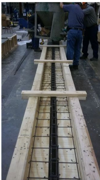
(c) Concrete pouring
