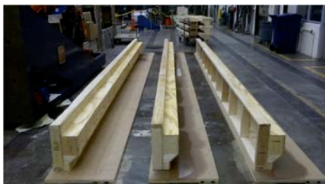
(a) Formwork construction
