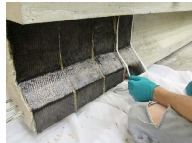
(c) Applying shear CFRP
