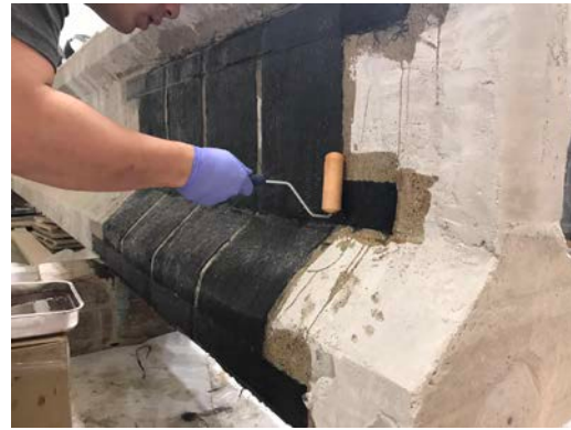
(e) Applying longitudinal strips
