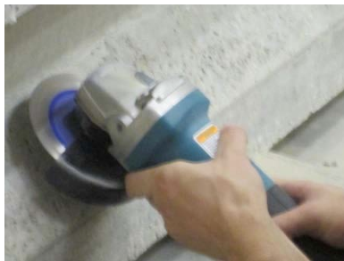
(a) Surface grinding
