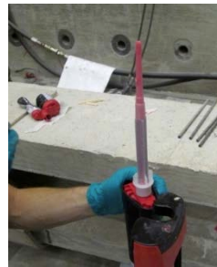
(e) Applying Hilti HIT-RE 500 epoxy
