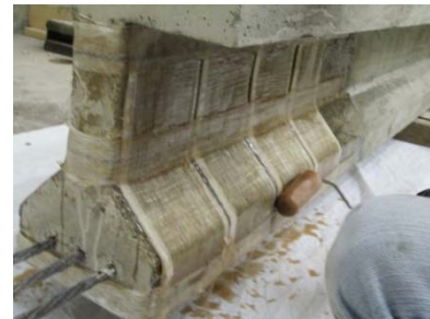
(f) Saturating GFRP anchors
