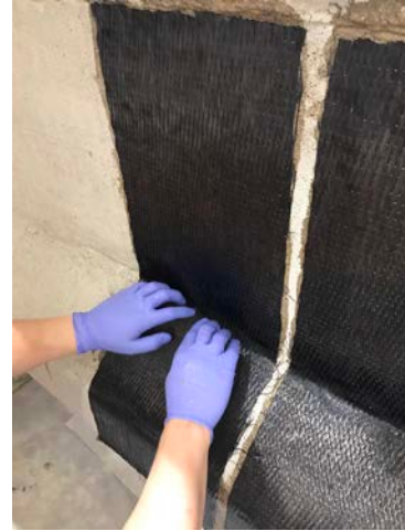
(c) FRP laminates application
