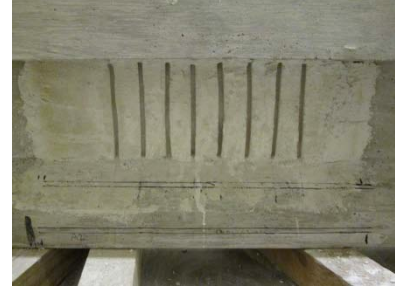
(c) Foam removed and longitudinal notches marked
