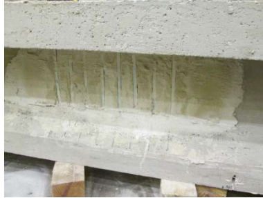
(b) Mortar repair with foam notch placed
