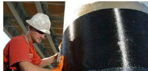
(b) Wet layup of CFRP on column
