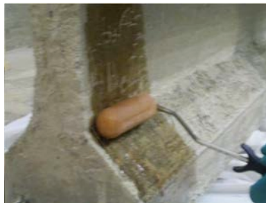
(b) Epoxy saturation of concrete
