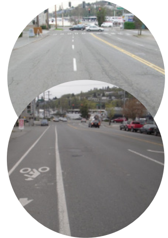
Stone Way Rechannelization: Before and After Study
