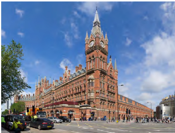
Figure 3-1. St. Pancras Station head house (Wikipedia).
