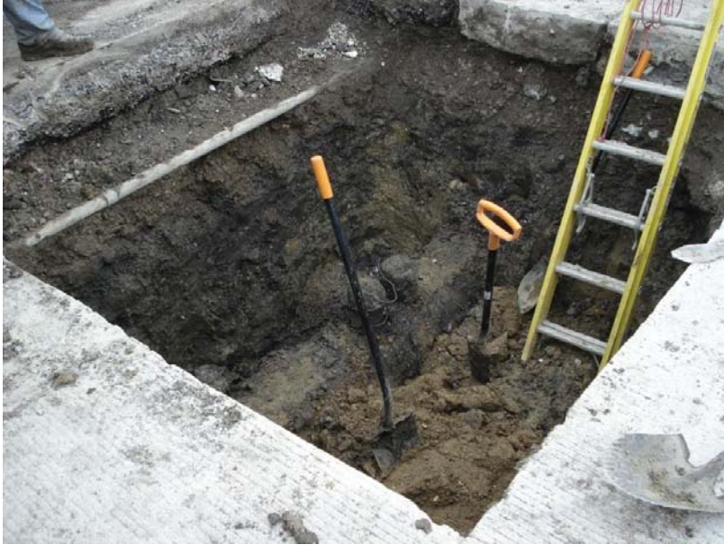
Figure 60 - ECDA excavation at the Utility E Site-1
