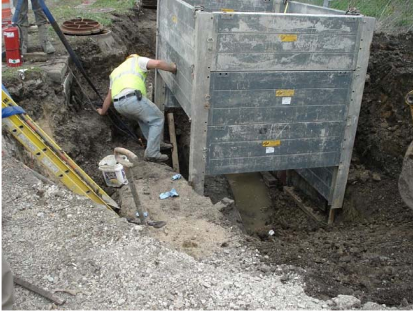
Figure 62 - ECDA excavation at the Utility-E Site-2
