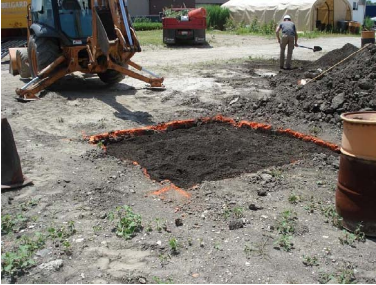
Figure 39 - View of the backfill in Section-1
