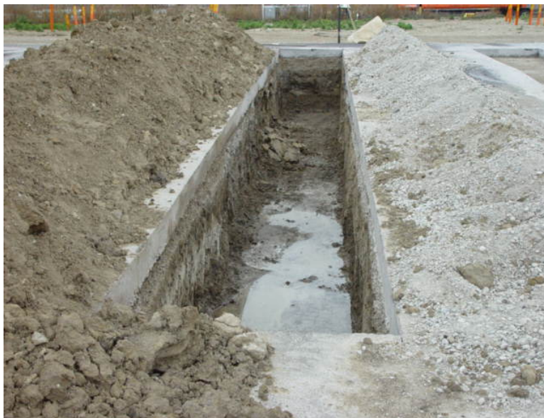
Figure 24 - Trench-A at GTI facility for corrosion monitoring
