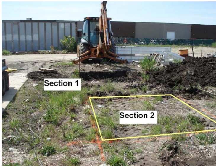
Figure 37 - Excavation of the test section at GTI testing facility
