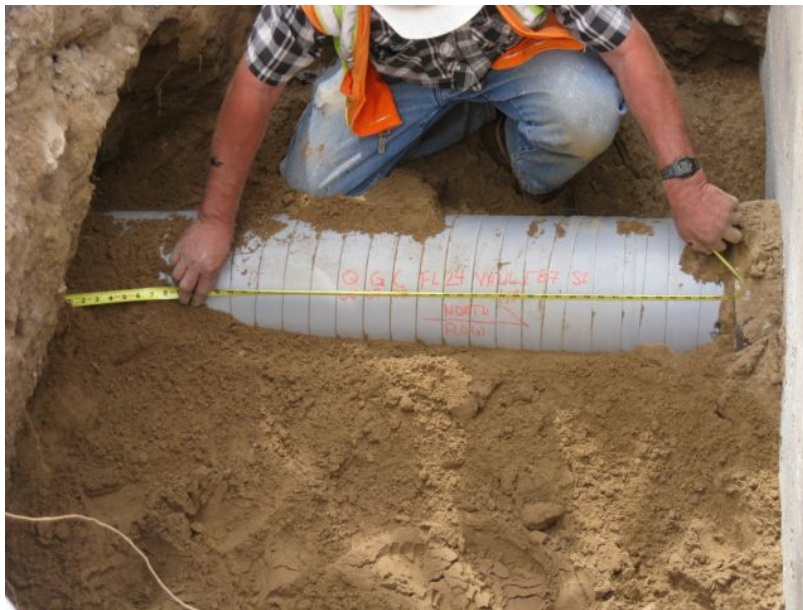
Figure 51 - View of the test section at Site-1
