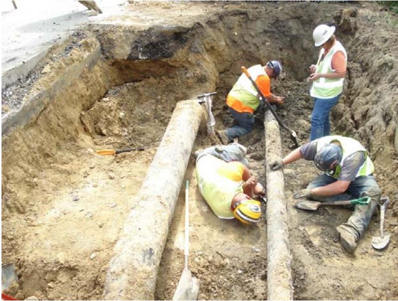
Figure 64 - Site preparation at the Utility-E Site-3
