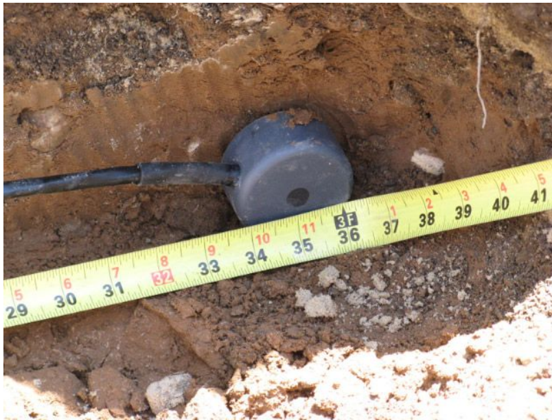
Figure 53 - View of the ER probe installation in the backfill
