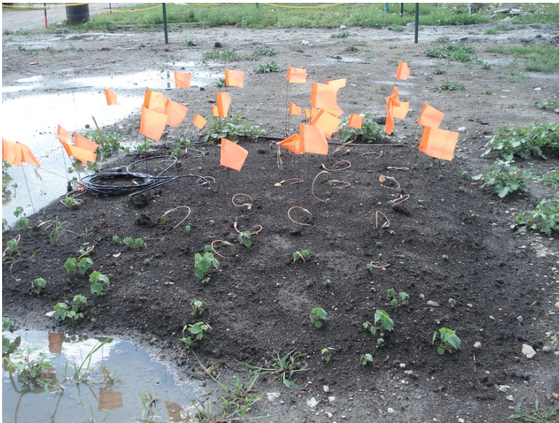
Figure 41 - View of the backfill in Section-3
