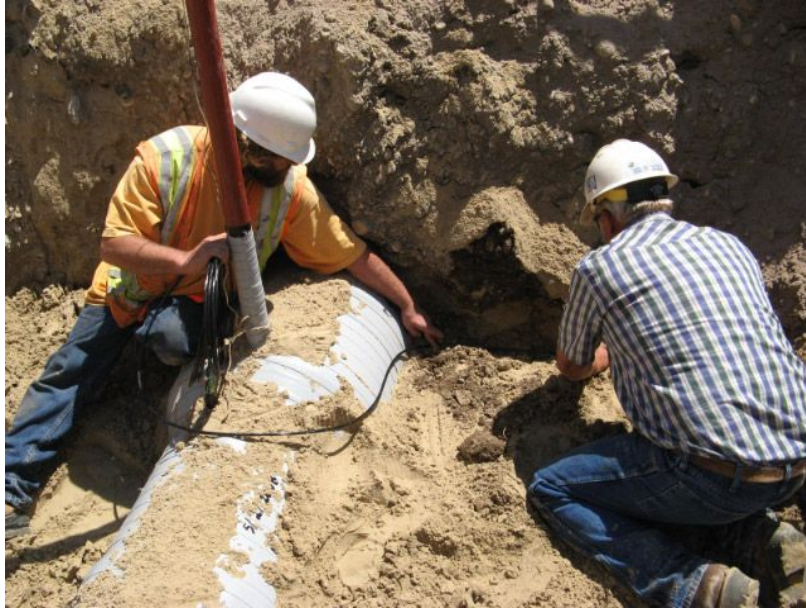
Figure 52 - Installation of the ER probe in Site-4
