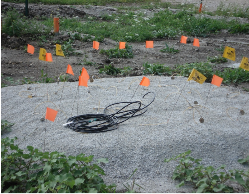
Figure 42 - View of the backfill in Section-4
