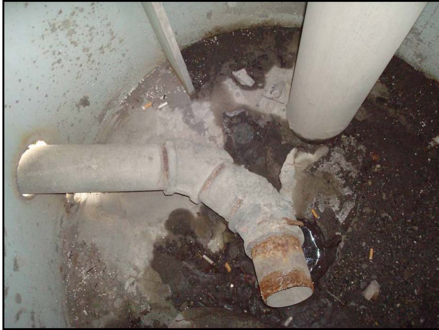
Photograph No. 56 – Looking up through the interior of the west column of pier 4C. Note: surface corrosion on the stiffening rings due to dysfunctional drainage system.
