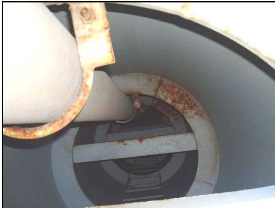
Photograph No. 56 – Looking up through the interior of the west column of pier 4C. Note: surface corrosion on the stiffening rings due to dysfunctional drainage system.
