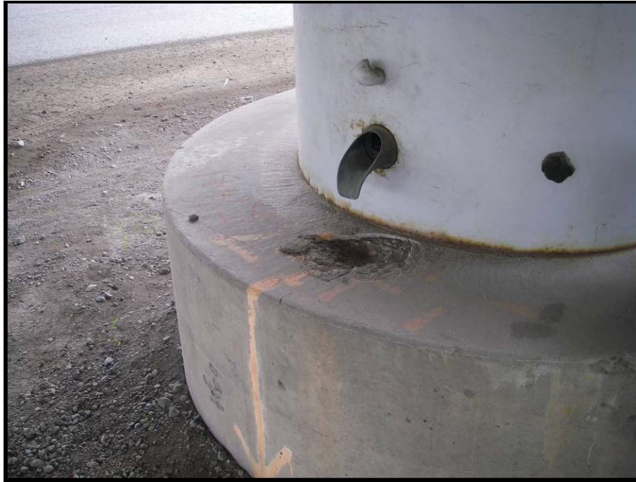
Photograph No. 86 – Looking south at the concrete collar of
