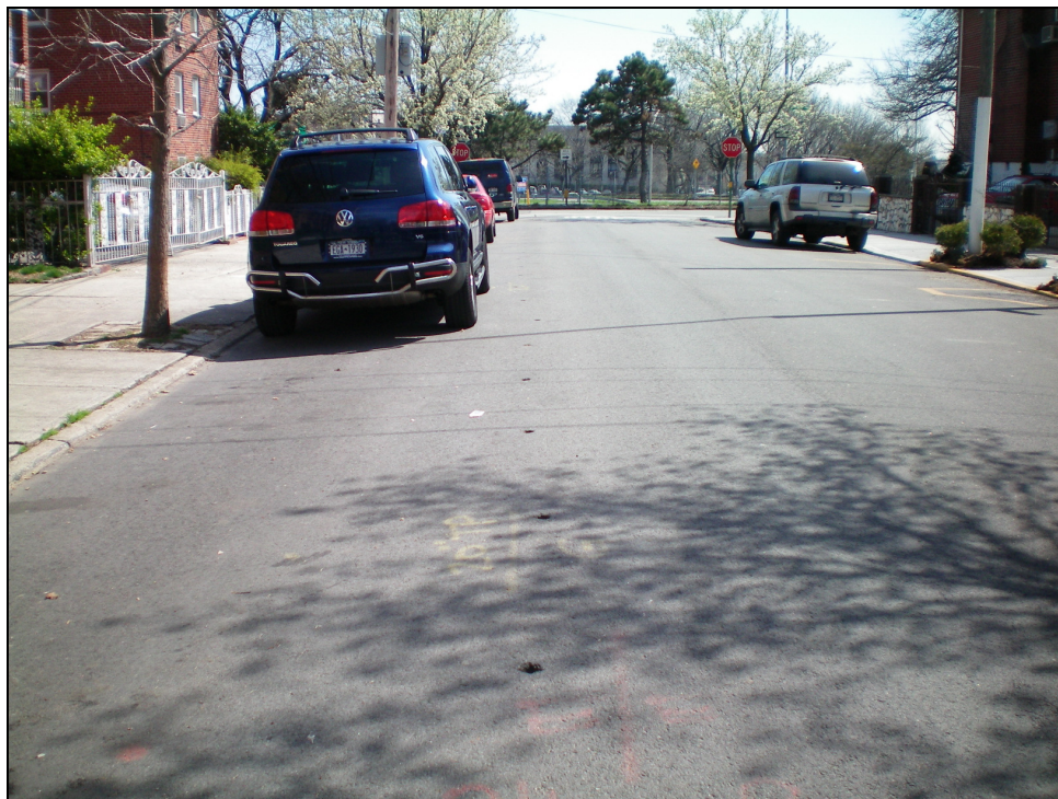
Condition 8: Asphalt Unacceptable for Potential Measurements Drilled Holes Required
