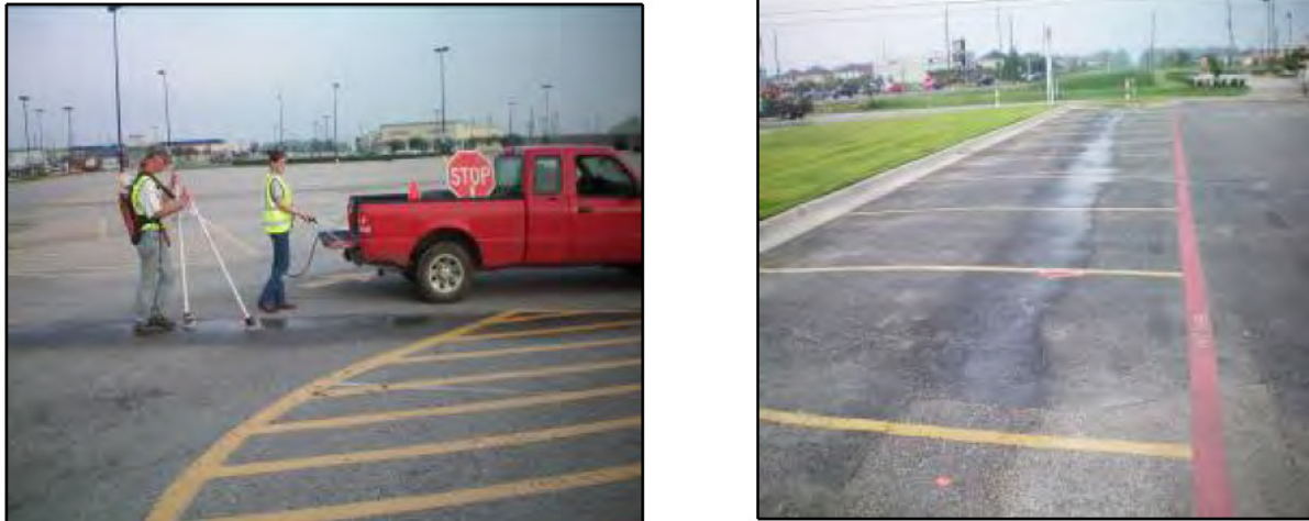
Figure 17: Pre-wetting for pipeline survey #5: Weathered asphalt
