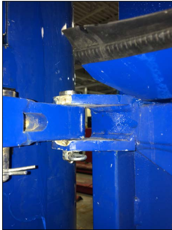
Figure 29. Photo. This hinge was instrumented for the structural integrity assessment.
