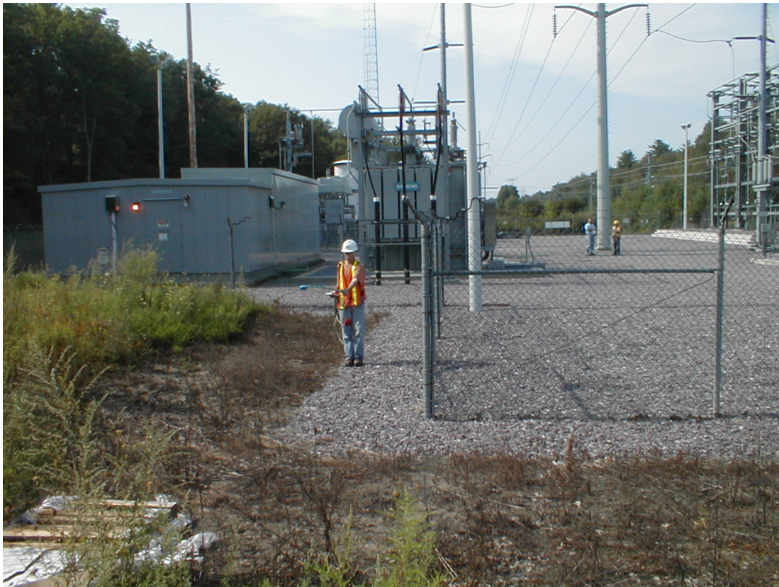
Figure B2. Sharon SS Looking Southwest, Tracks are at Far Right
