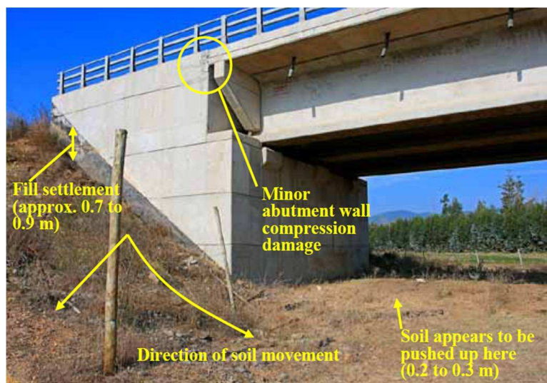
Figure 3.1: Settlement and lateral spreading deformation of northeast approach embankment to Mataquito River Bridge (FHWA, 2011).
