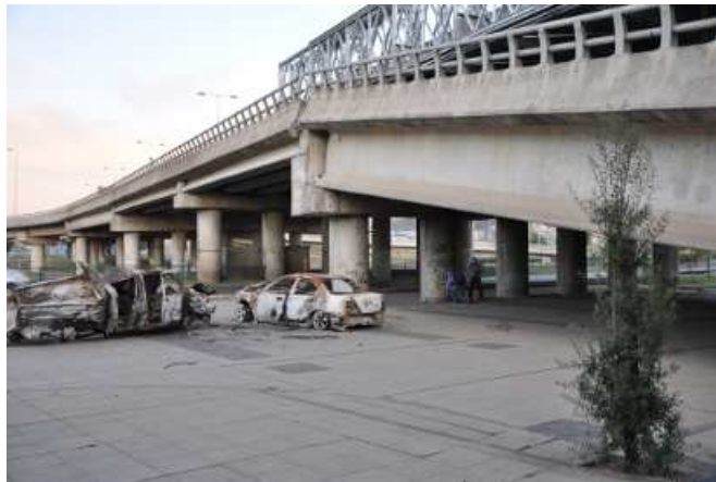
Figure 3.16: Lateral spreading and span collapse of northeast approach embankment to Llacolén Bridge (FHWA, 2011).
