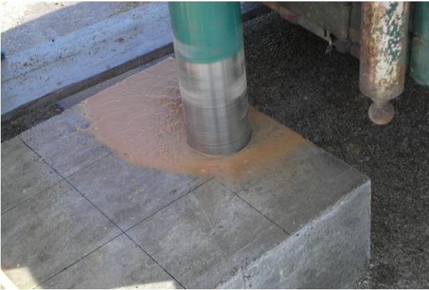
Figure 28. Coring of a large core block.
