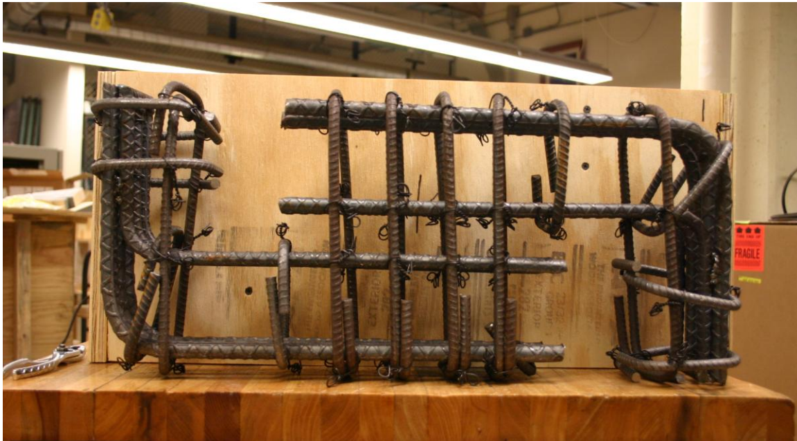
Figure 36. Completed rebar cage.
