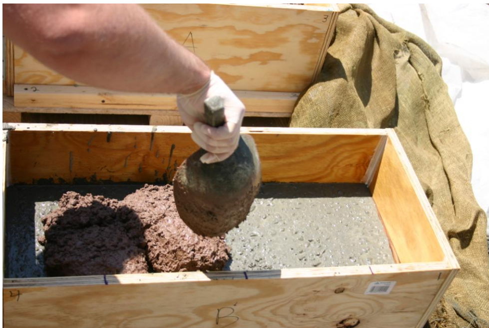
Figure 30. Concrete placement for small core block.
