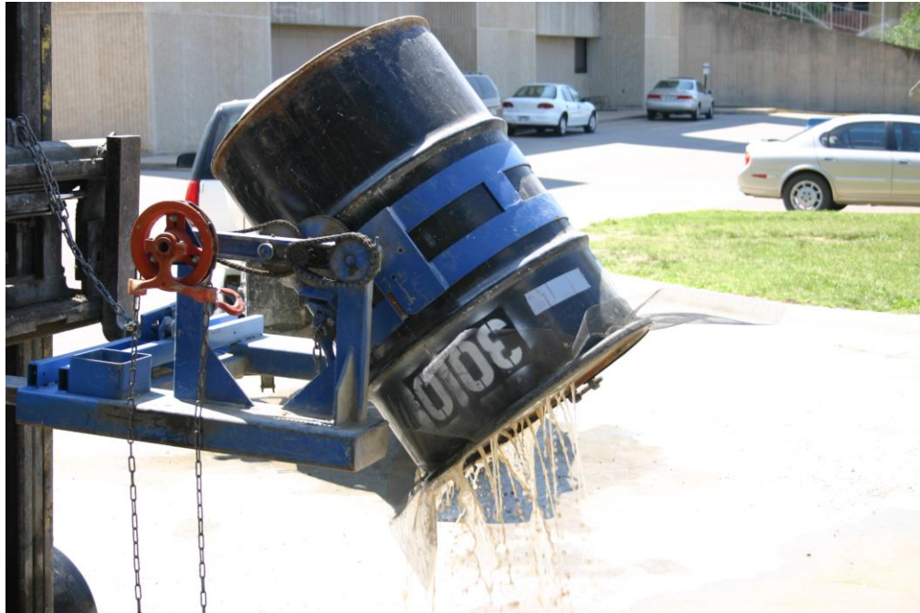
Figure 11. Water being drained for large concrete batch.
