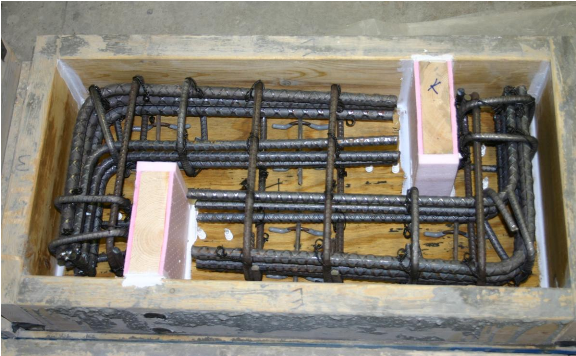
Figure 37. Monolithic specimen prior to casting.
