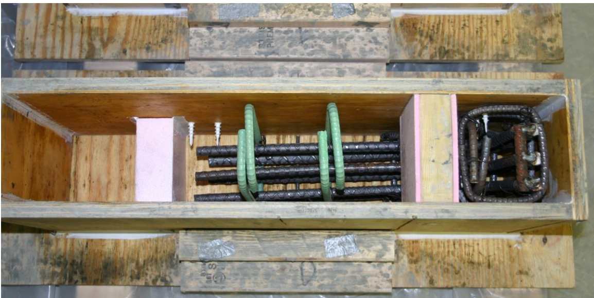
Figure 38. Cold-joint specimen prior to casting.
