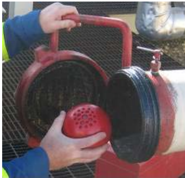
Figure 2. Insertion of SmartBall Tool in Standard Pig Launcher
