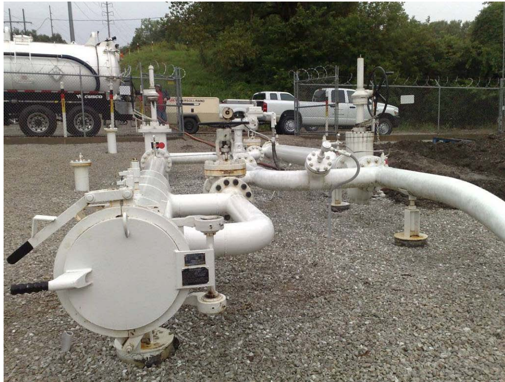
Typical Pig Trap Layout
