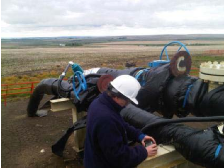
Figure 26. Measuring Gas Leak Flow Rate
