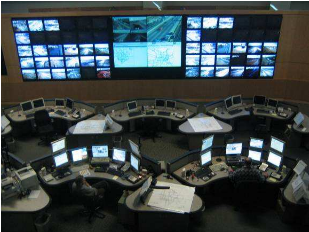
Figure 4. View of the Mn/DOT Regional Traffic Management Center
