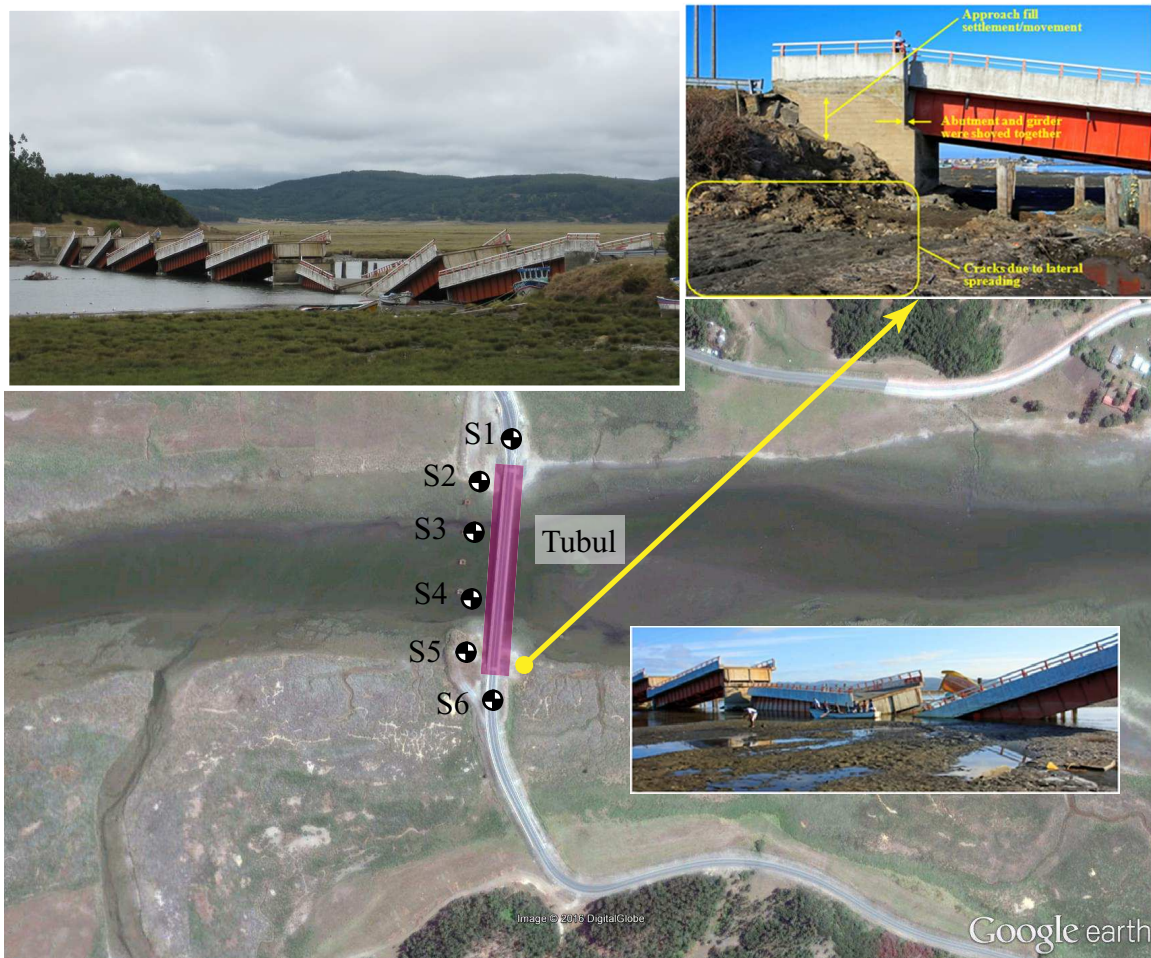
Figure 4.6: Location of the Puente Tubul.
