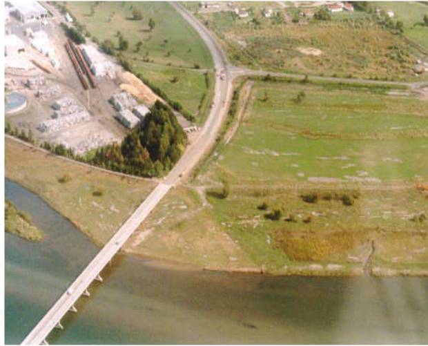
Figure 1.2: Northern approach to Landing Road Bridge two days after the Edgcumbe event. Ejected sand is visible on the ground surface (Berrill and Yasuda, 2002).
