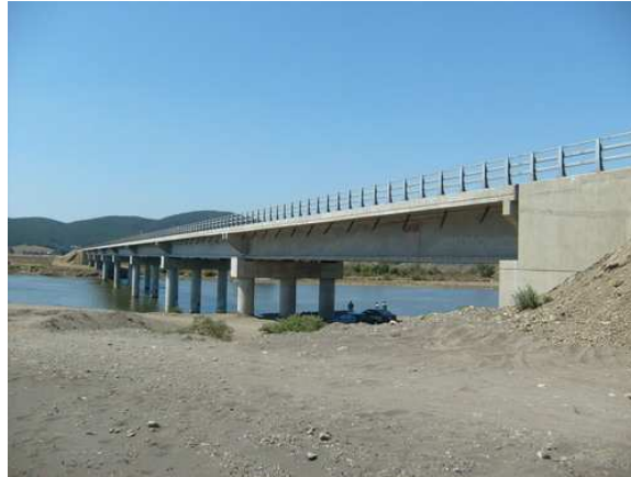
Figure 4.9: Puente Mataquito looking northeast from the southwest approach. Photo retrieved January 14 2013, www.panoramio.com/photo/8172577 .
