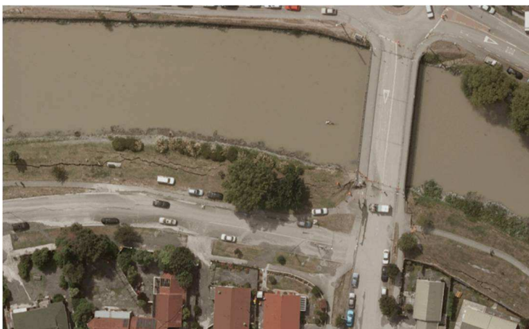
Figure 1.8: Avondale Road Bridge after the Christchurch event. Lateral spreading cracks are visible near the southern approach and along the river bank (LINZ, 2011).
