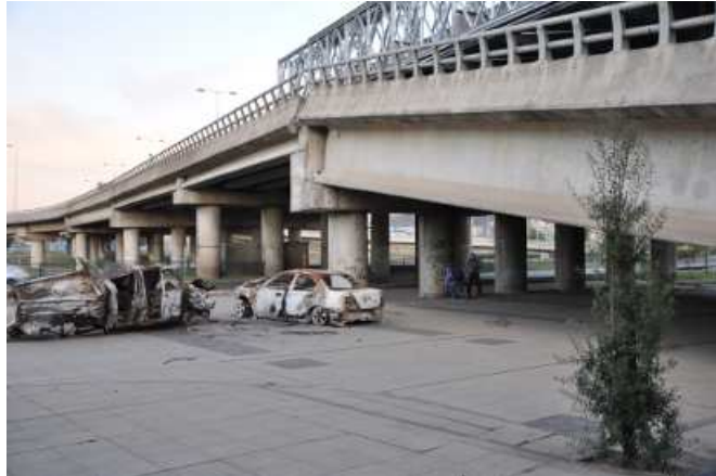
Figure 1.5: Lateral spreading and span collapse of northeast approach embankment to Llacolén Bridge (FHWA, 2011).
