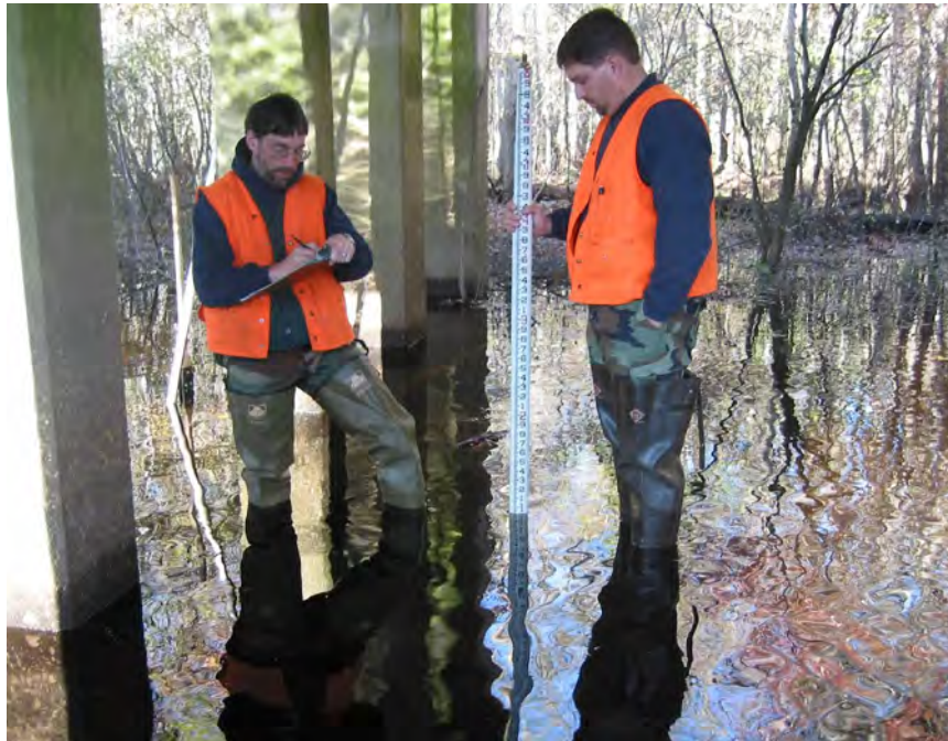
Figure 8. Probing in standing water to determine clear-water scour depth at structure 342050111100 on U.S. Route 501, crossing the Little Pee Dee River floodplain in Marion County, South Carolina. (Photograph by U.S. Geological Survey, South Carolina Water Science Center, December 3, 2002)
