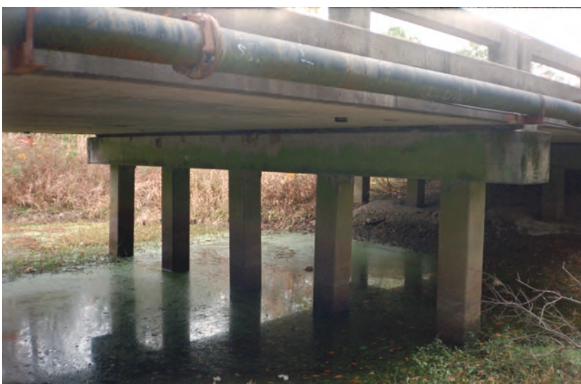
Figure 13. Concrete pile bent with common pile dimension at structure 182007800200 on U.S. Route 78, crossing Polk Swamp in Dorchester County, South Carolina. (Photograph by the U.S. Geological Survey, South Carolina Water Science Center, November 26, 1996)
