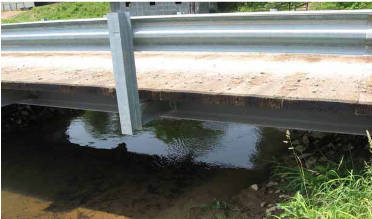
Figure 3.10: Guardrail Condition on Peel Tree Bridge
