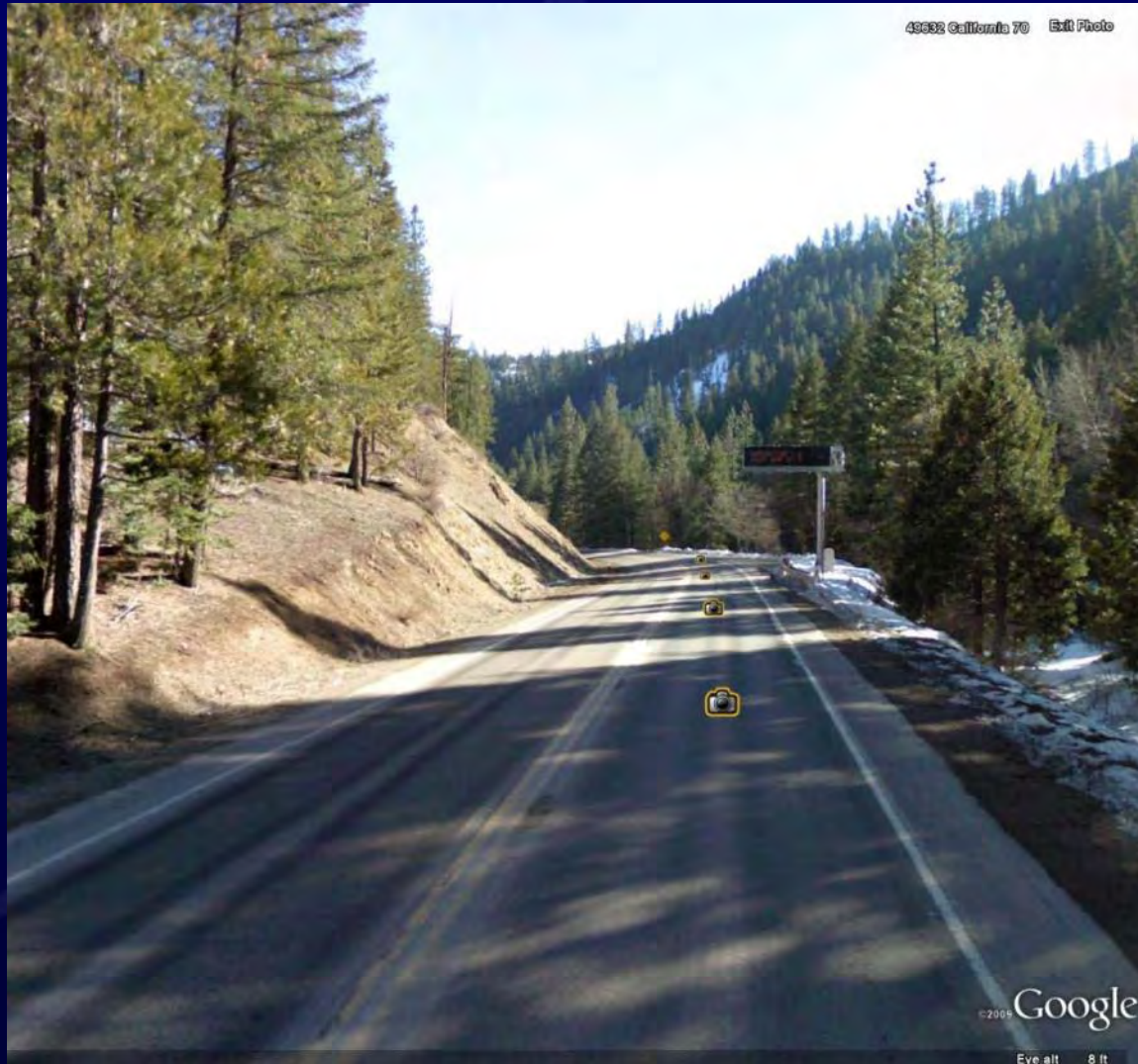
Photo from Google Street View
