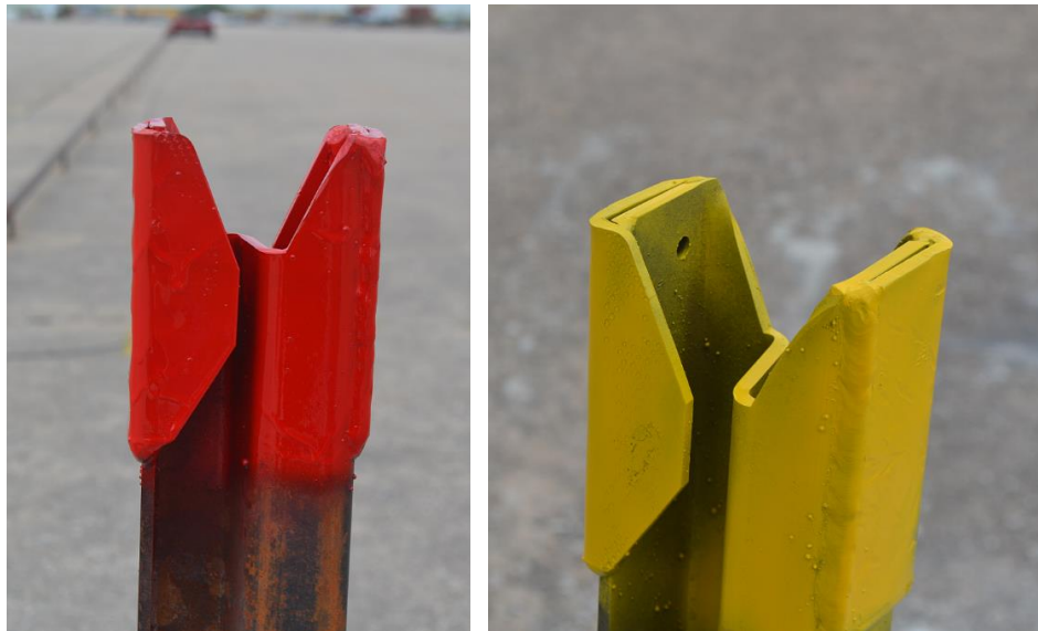
Figure 57. MWPs with Steel Plate Edge Protectors
