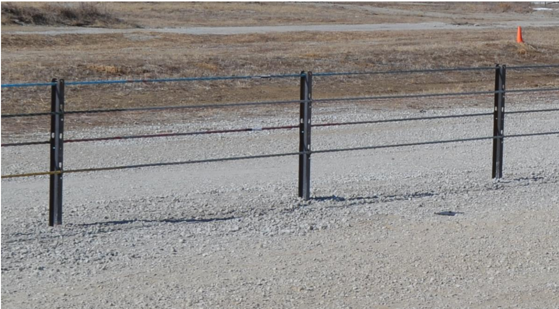
Figure 1. Current Cable Median Barrier Prototype
