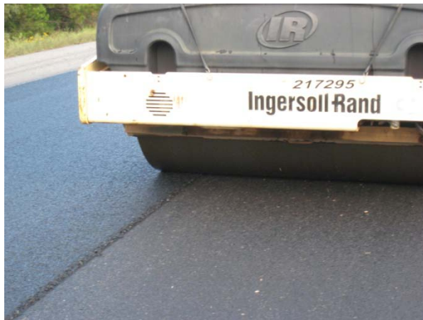
FIGURE 32 Cold Roll Rolling Pattern.
