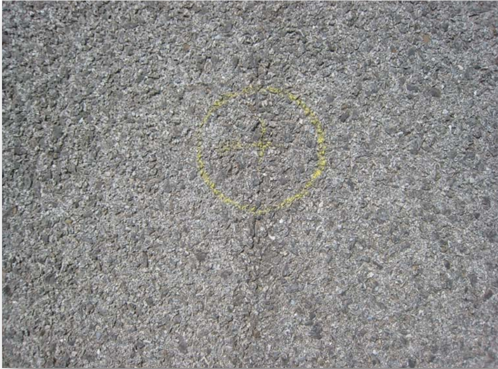
FIGURE 3 Site #1 – Good Condition.
