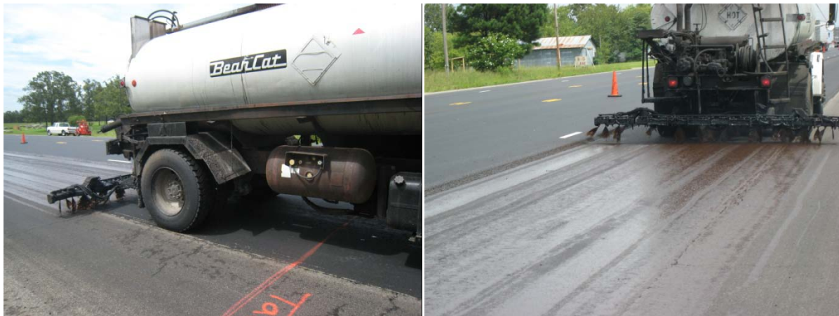
FIGURE 29 Tack Coat (SS-1) Applied by Contractor.
