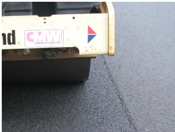
FIGURE 31 Hot Pinch Rolling Pattern.
