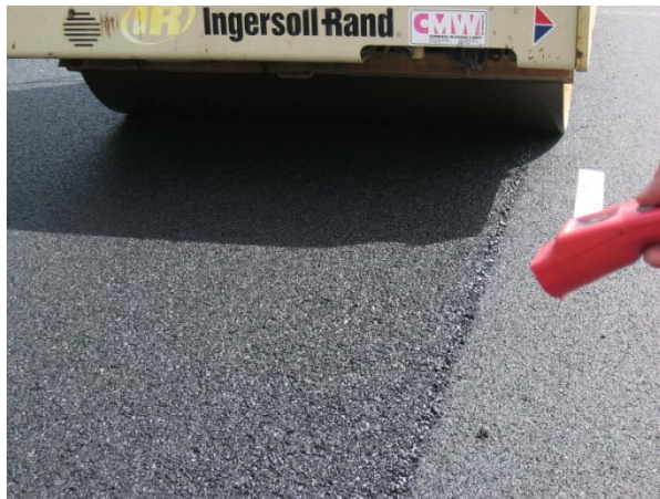
FIGURE 30 Hot Overlap Rolling Pattern.
