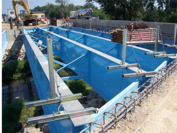
Figure 2. Multi-girder steel bridge with concrete deck to be applied.
