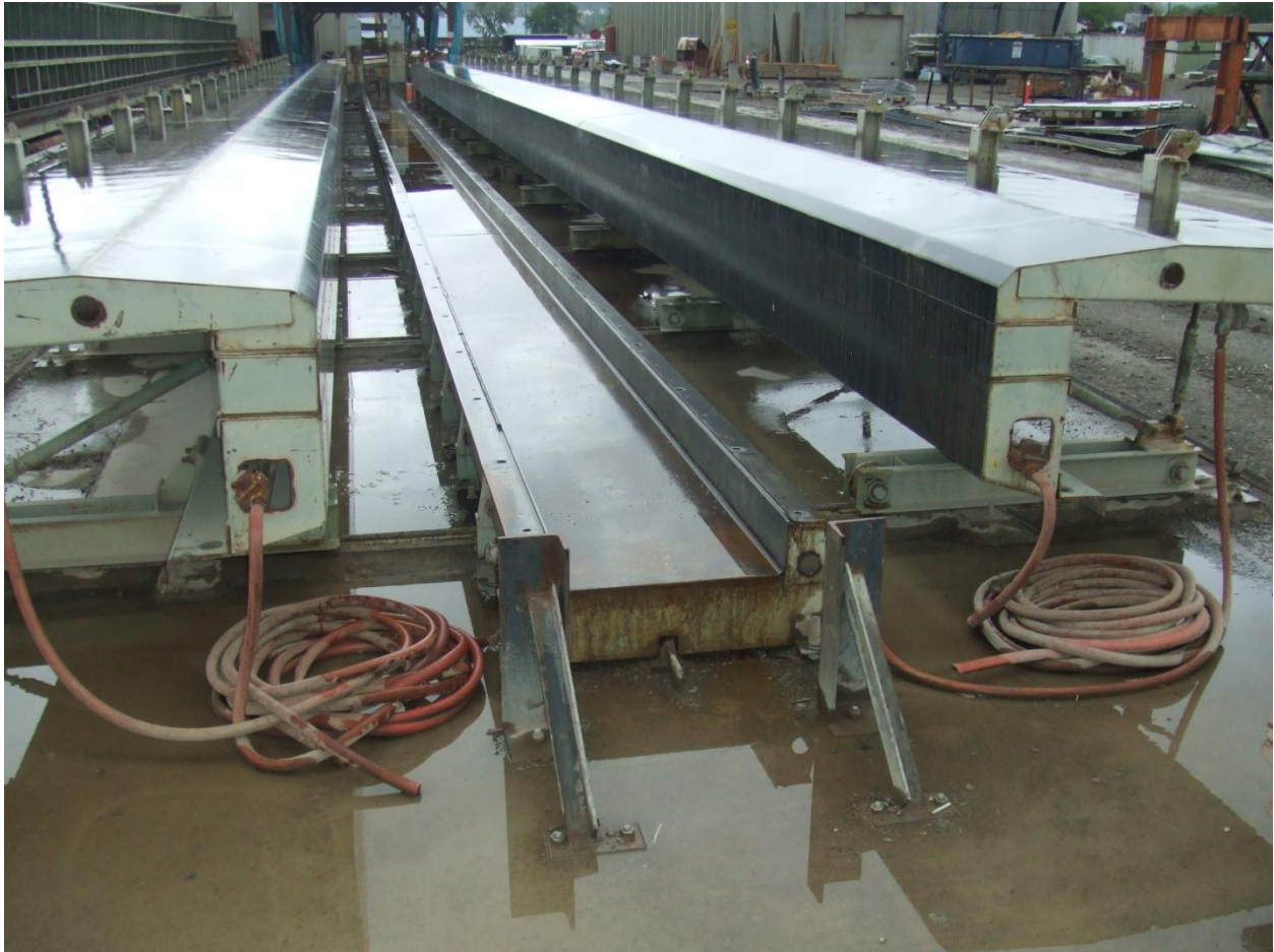
Figure 56. Photo. The form pictured uses steam heat pumped through the red tubing to control the cure temperature. Woodworth 2008
