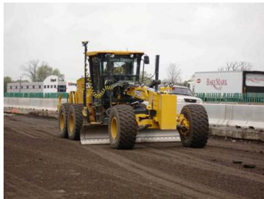
Figure 15. A Motor Grader Using TOPCON CORS-Based GPS Machine Guidance on I-94 Illinois Tollway Reconstruction (Corrections are being Received by Cellular Connection to a Central Server)
