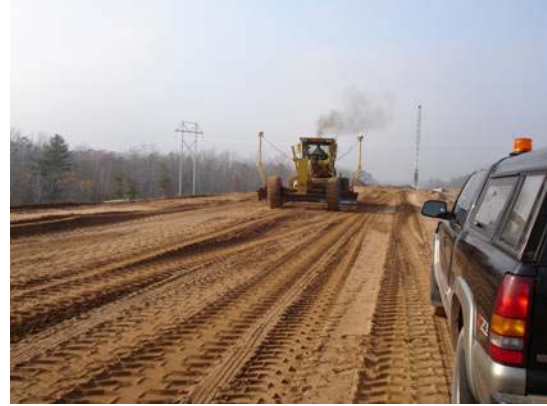
b) Work on Northbound Main Line
