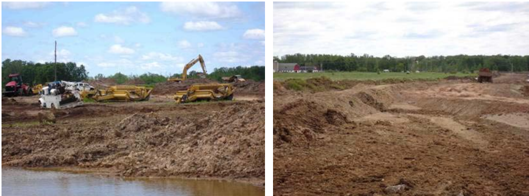
Figure 6. Initial Excavation, Haul, and Fill on Oconto Bypass Project
