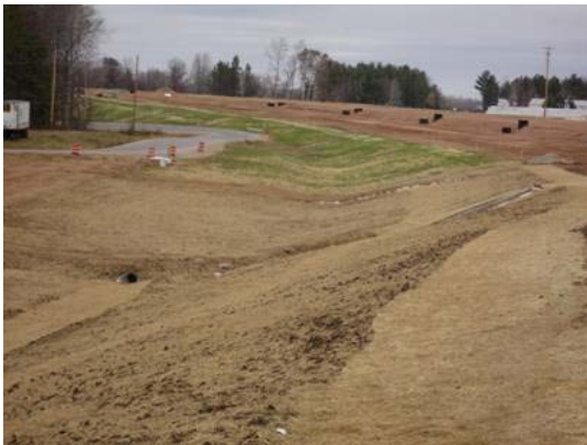
a) Finished Slopes and Ditch
