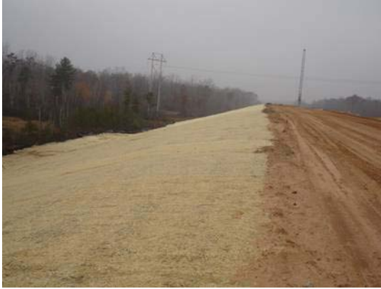
a) Finished Slope and Ditch
