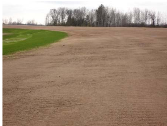
b) Finished Mainline Sub Grade
