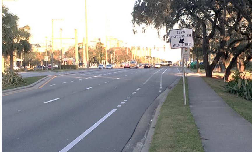
Figure 8-3 Implementation of through bike lane at intersection.
