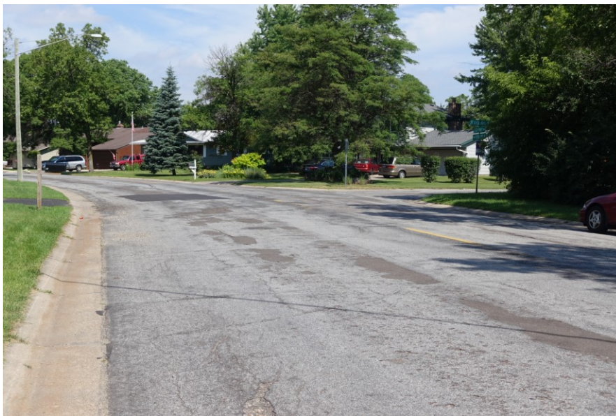
Figure 6. Deteriorating Street Surface in Brooklyn Park
