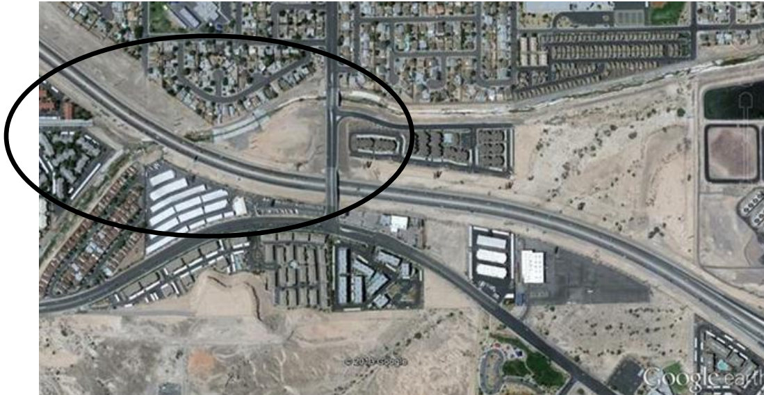
Figure 4.12: Reverse curve located on US 95 and Russell Rd interchange, curve with smaller radius circled
