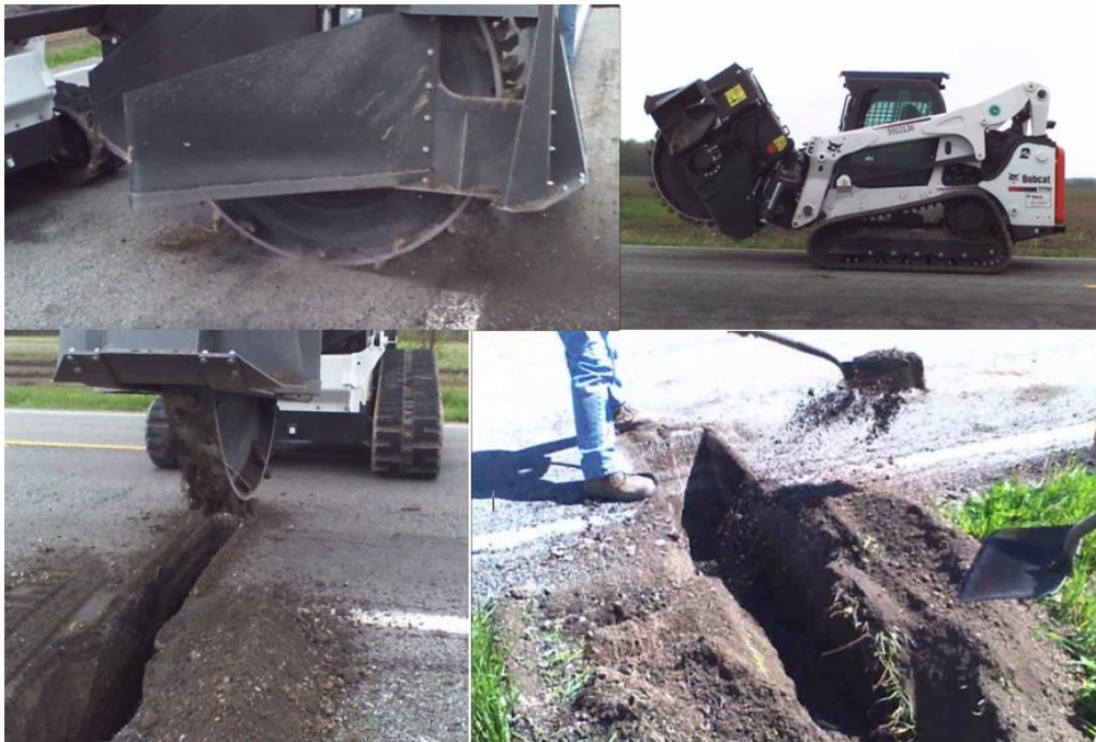
Figure 27. Rock Saw Excavation.
