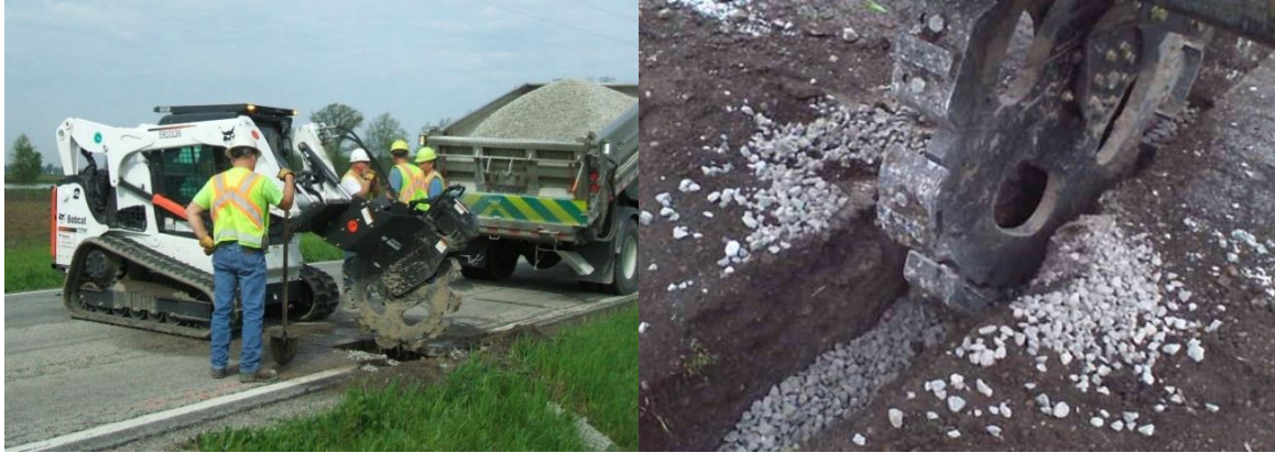
Figure 24. Bobcat with Compactor Attachment.
