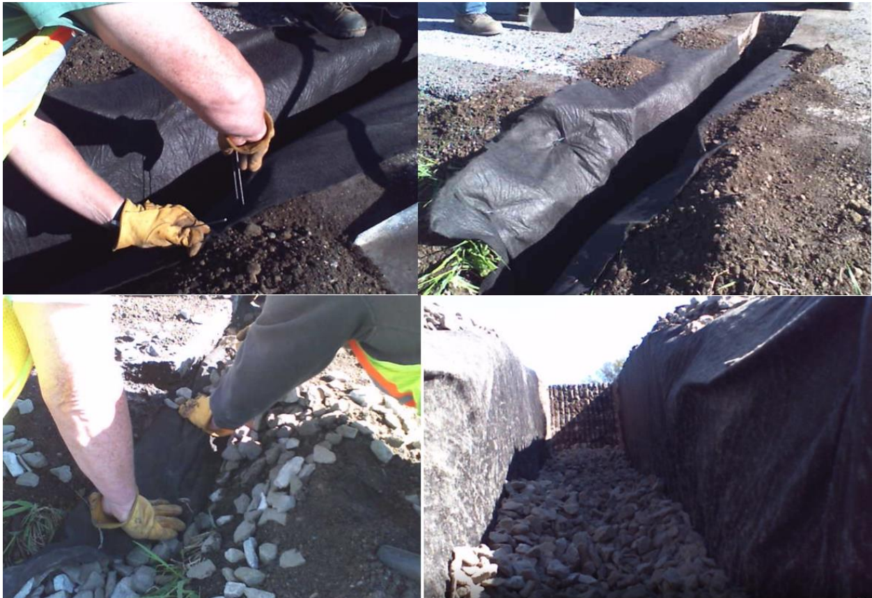
Figure 28. Fabric Installation.
