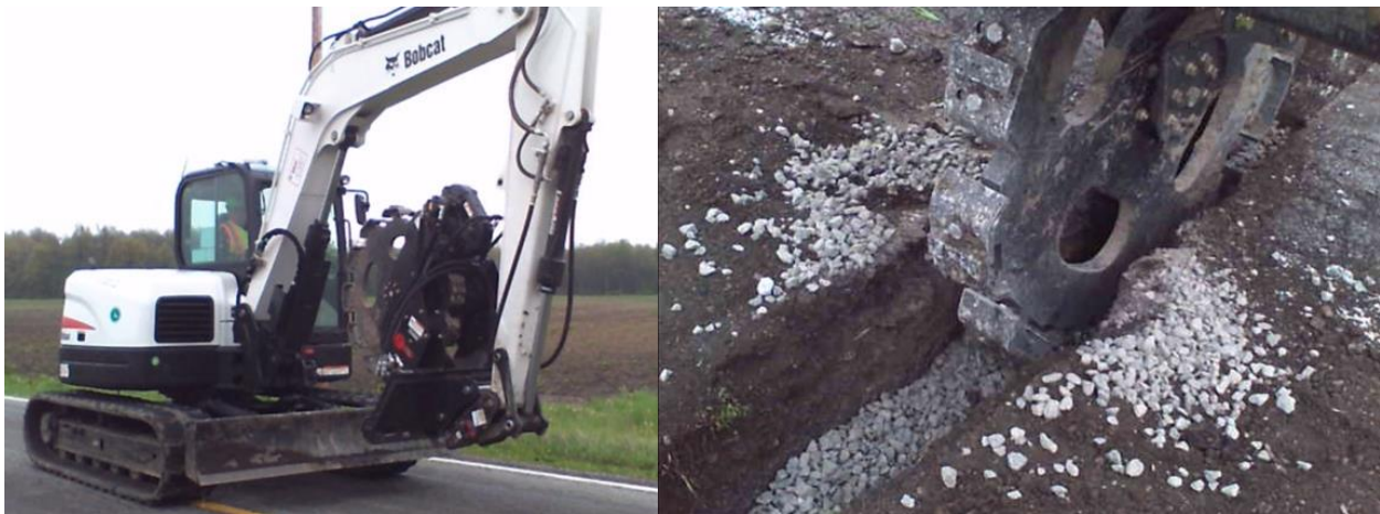
Figure 30. Compaction.
