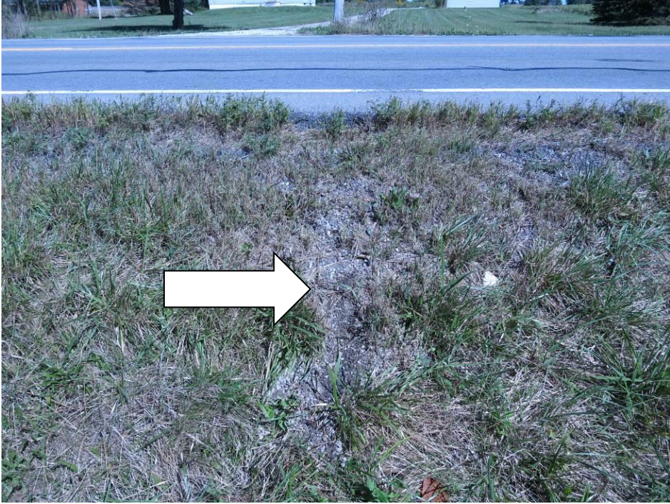
Figure 6. Finished Aggregate Roadside Drain.
