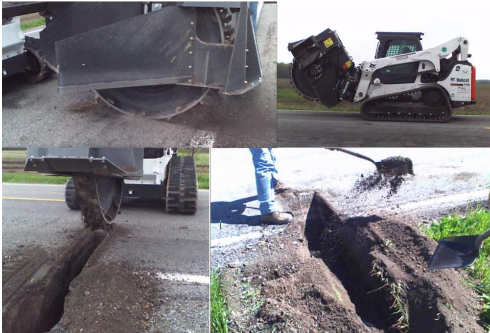
Figure 2. Rock Saw Excavation.
