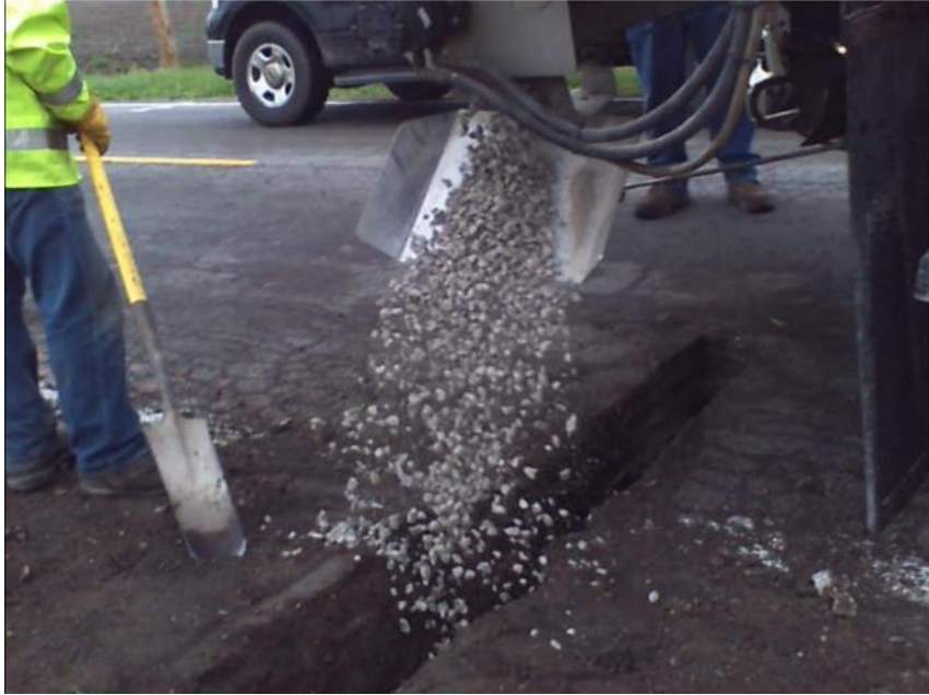
Figure 29. Backfilling.
