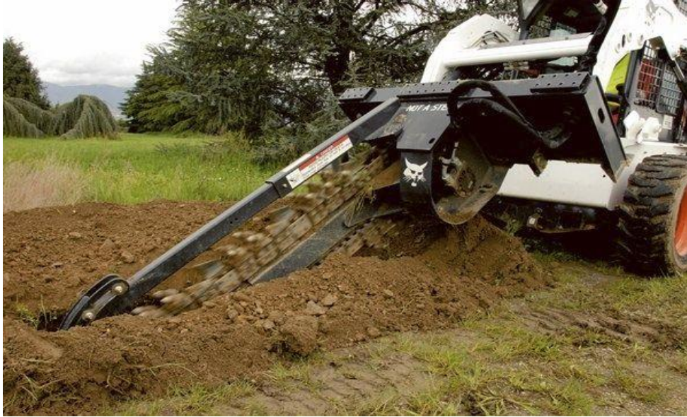
Figure 9. A Bobcat Track Loader with Trencher Attachment in use. [ http://www.directindustry.fr/prod/bobcat/product-31379-1180679.html ]
