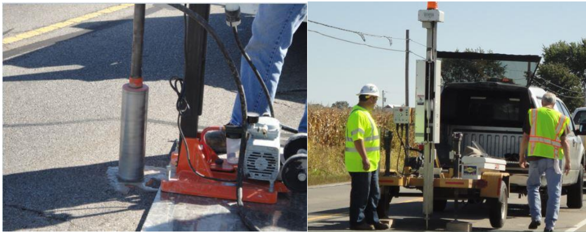
Figure 13. Coring (left) and Dynamic Cone Penetrometer (DCP) Testing (right).
