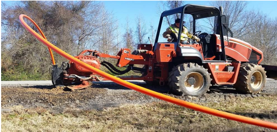
Figure 12. A vibratory Cable Plow. [ http://williscable.com/services/ ]
