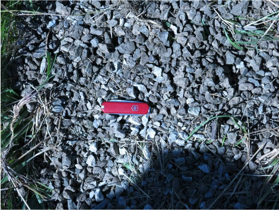
Figure 7. Close-up View of Finished Aggregate Roadside Drain.
