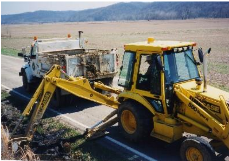
Figure 5. Backhoe with Bucket Excavating for Road Drainage [ http://www.odotonline.org/photoarchive/ ].
