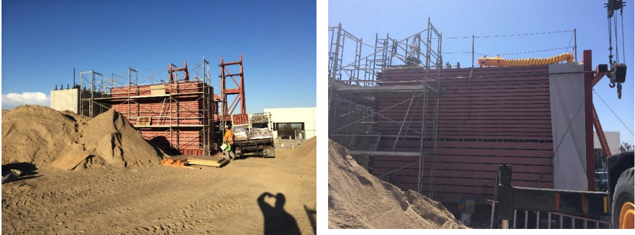
Figure F-6: Photographs of the installation and assembly of laminar container
