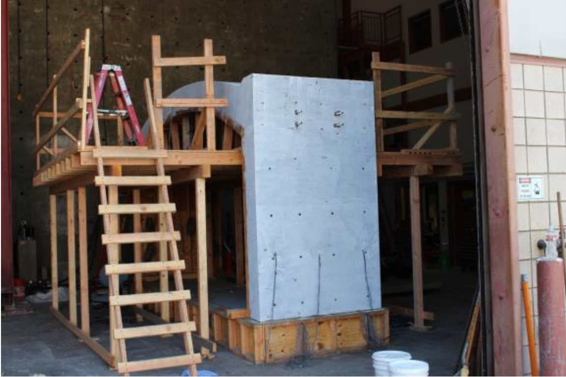
Figure C-12: After removal of the form
