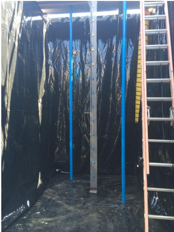
Figure F-5: Photographs of the installation of the liner
