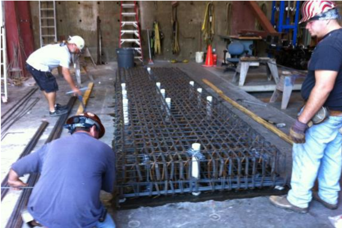
Figure C-2: Formation of reinforcing in the slab
