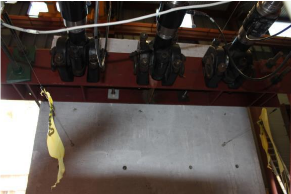
Figure C-13: Installation of the actuators on the South wall
