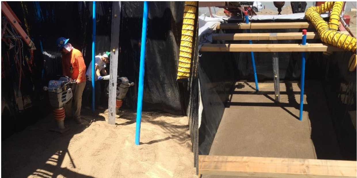
Figure F-7: Photographs of the soil compaction
