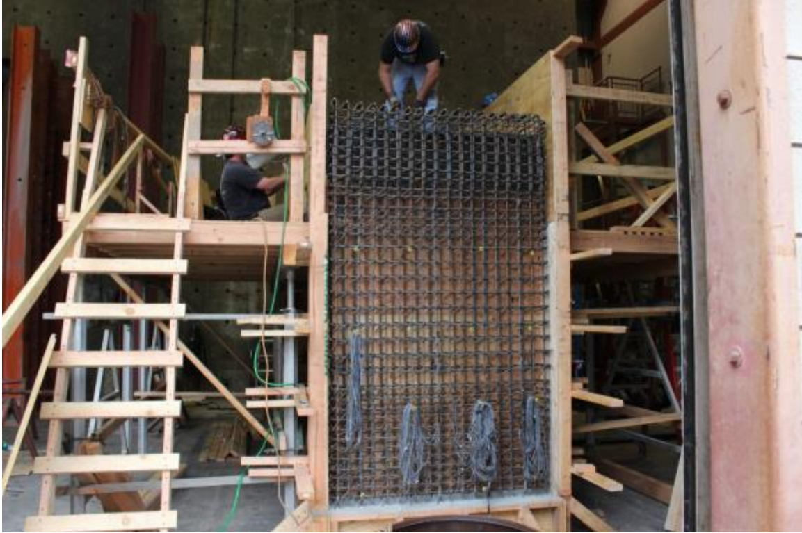
Figure C-6: Reinforcing and form for the wall
