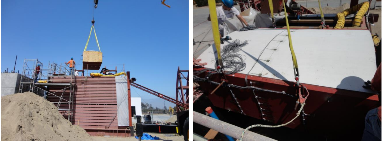
Figure F-7: Photographs of the tunnel replacement
