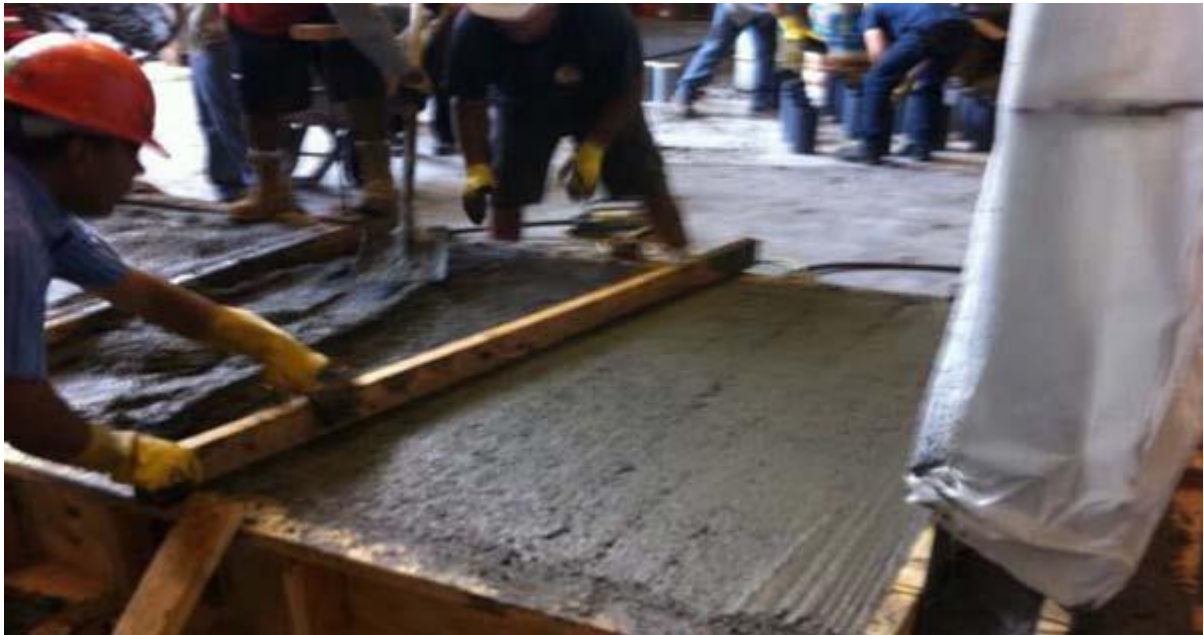
Figure C-5: Smoothing surface on concrete for the slab
