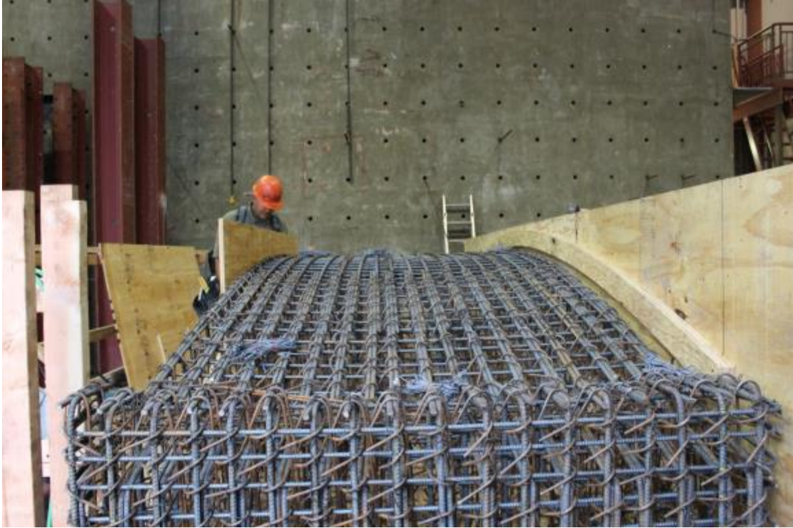
Figure C-8: Reinforcing and form for the roof
