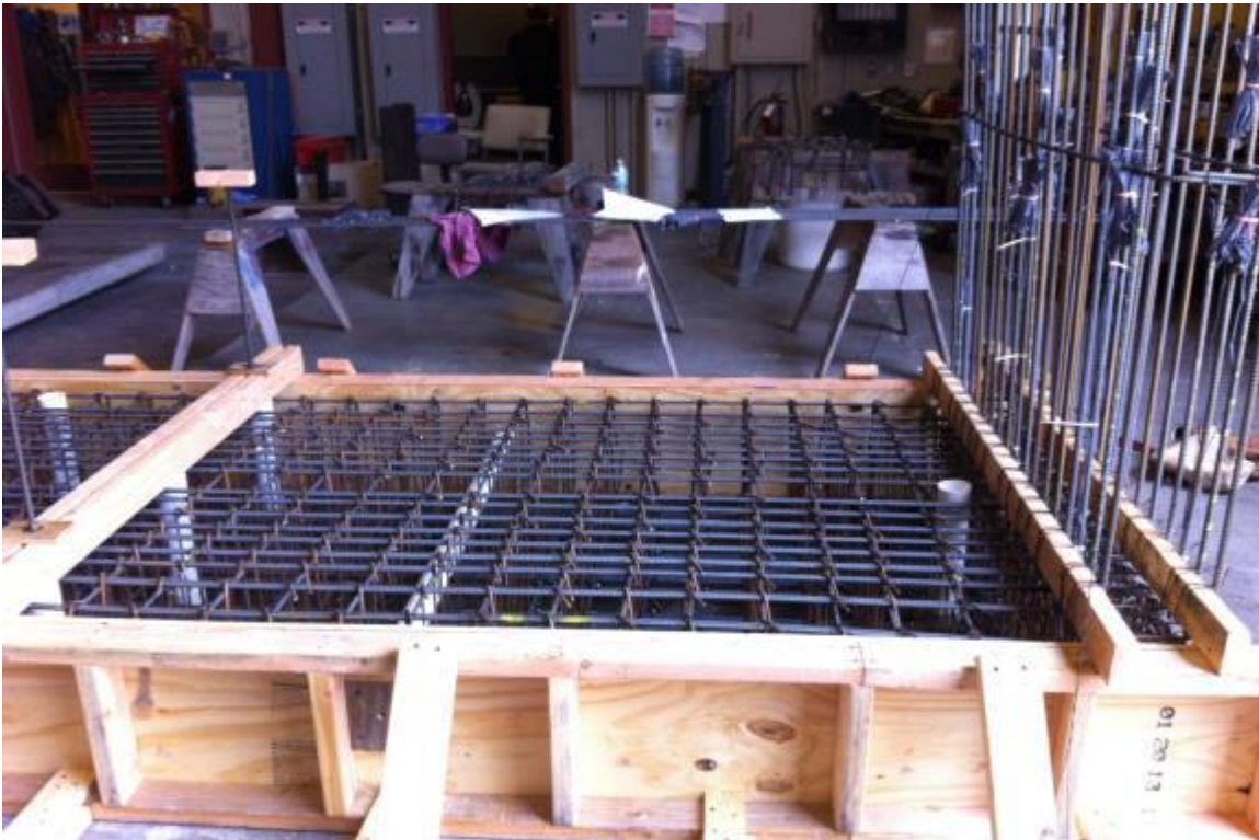
Figure C-3: Form for concrete pour in the slab
