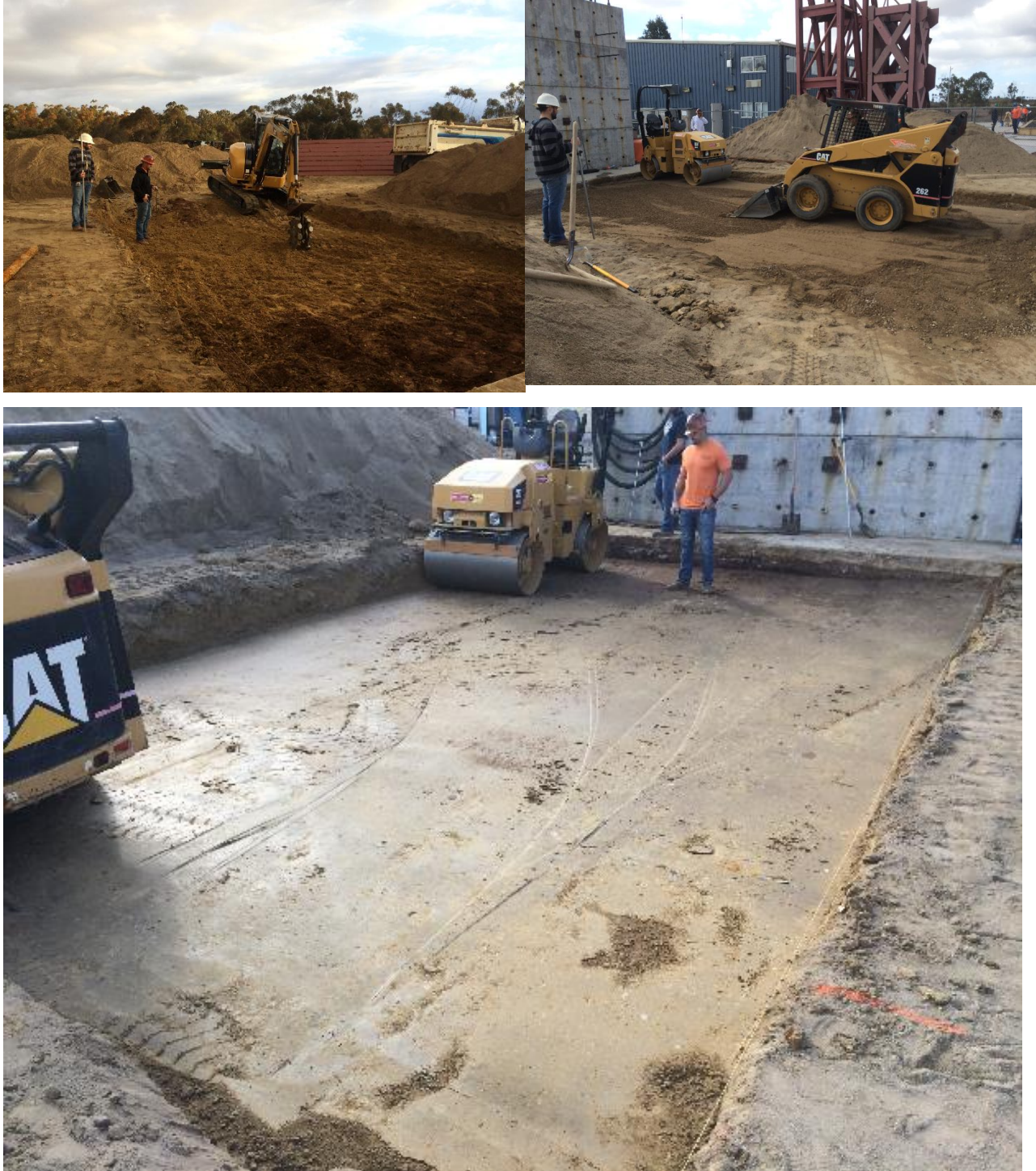
Figure F-3: Photographs of the construction for the foundation
