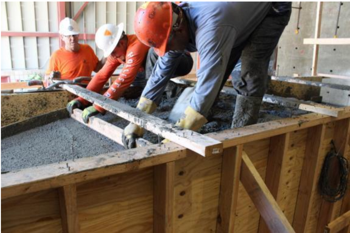
Figure C-11: Smoothing surface on concrete for the roof
