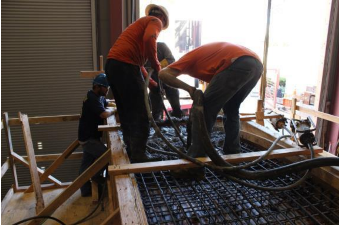
Figure C-10: Concrete pour for the roof
