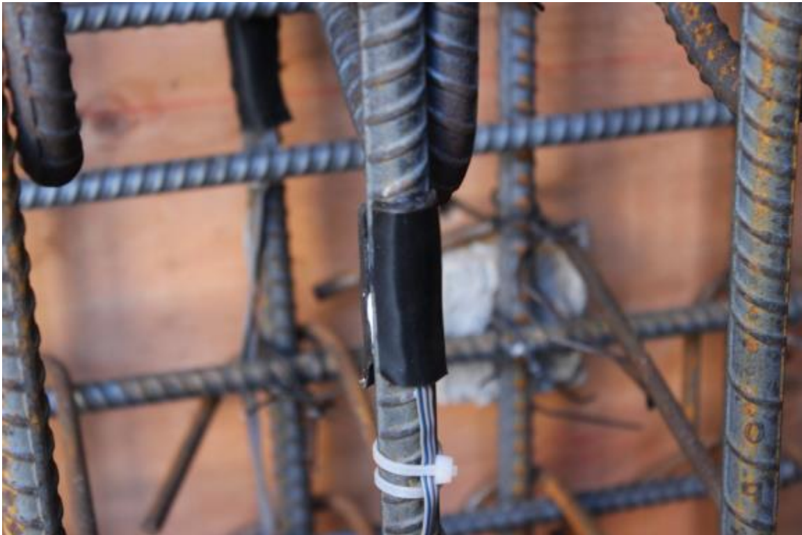
Figure C-7: Installation of strain gauge on the longitudinal reinforcement in the wall
