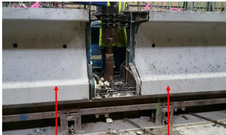
SCC Girder North End
