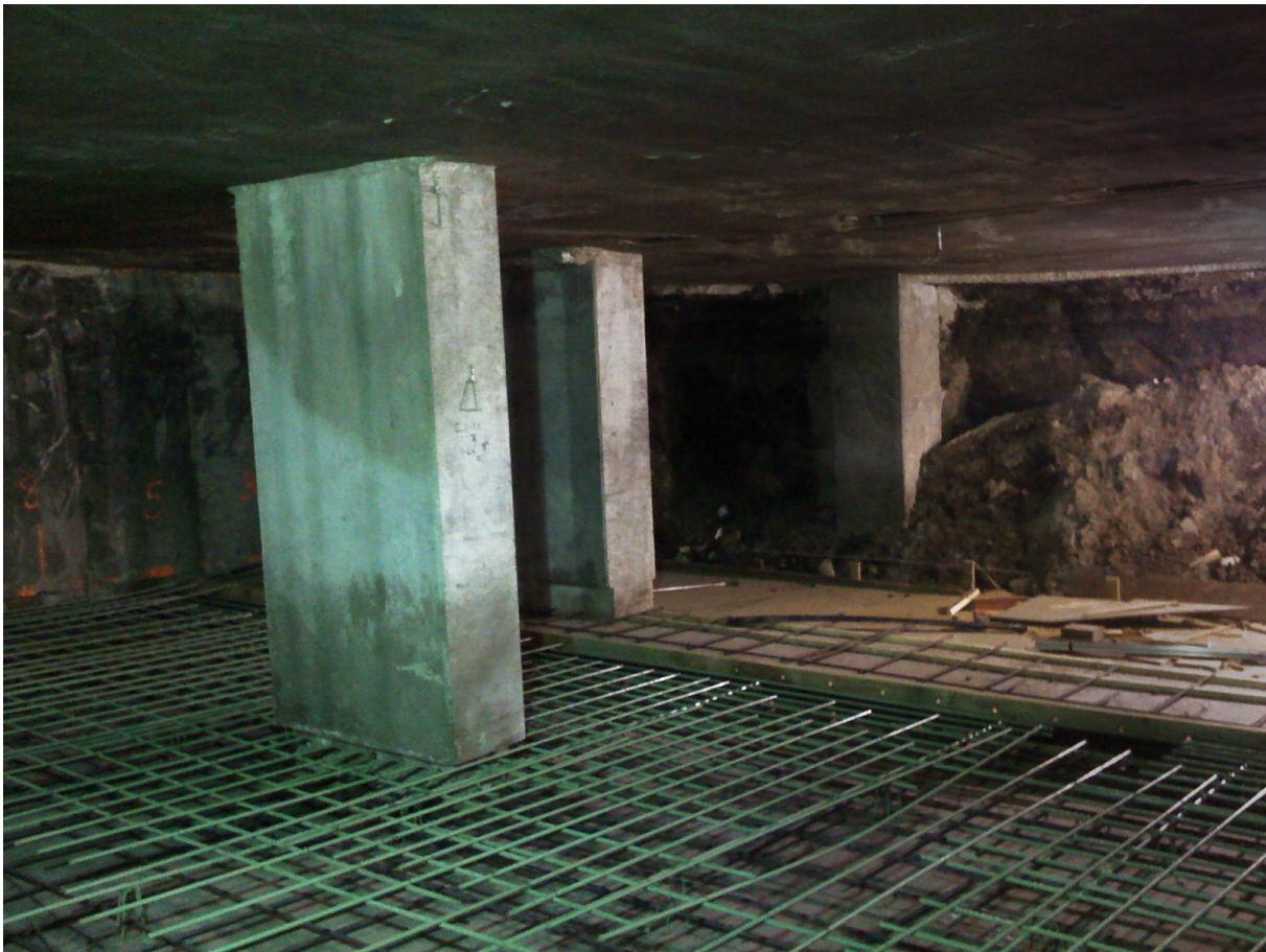
Figure 4.16: Top-down construction
