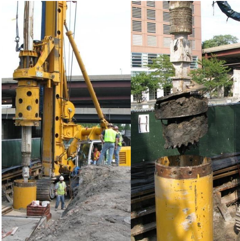
(4.13.1) External casing released (4.13.2) Internal auger
