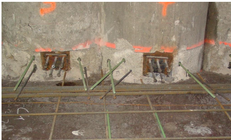
Figure 4.10: Detail of typical slab-wall connection.
