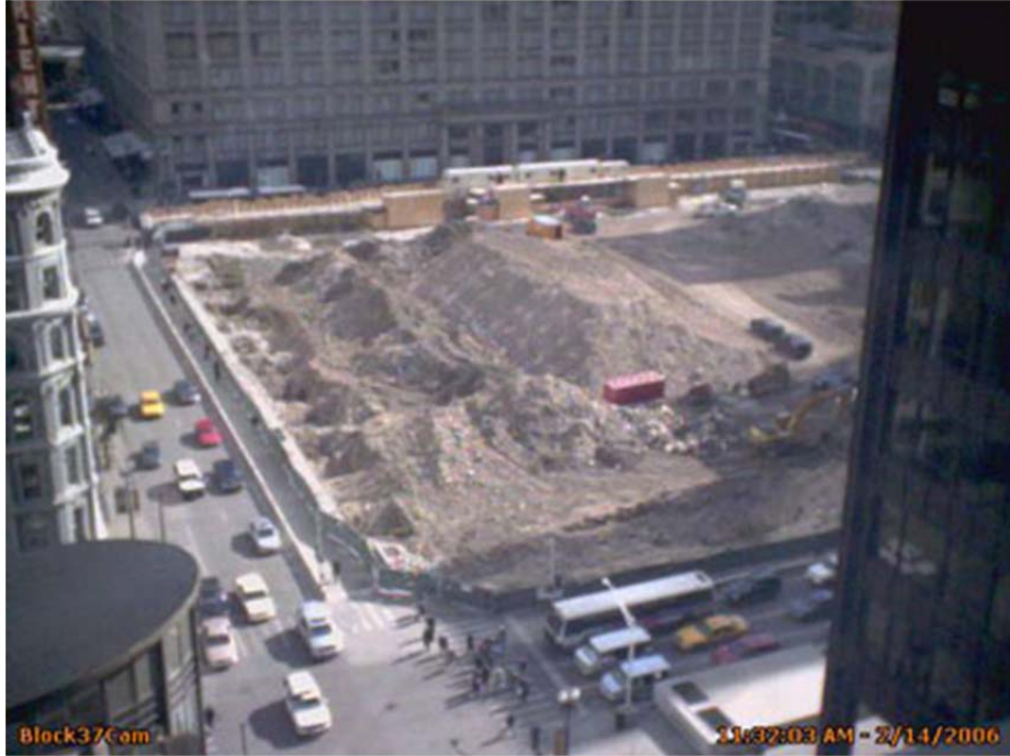
Figure 4-6: Webcam Photo during Potholing (Hill, 2006)
