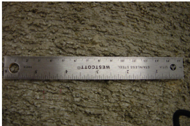
Figure 4.3.6 Astro turf textured concrete surface
