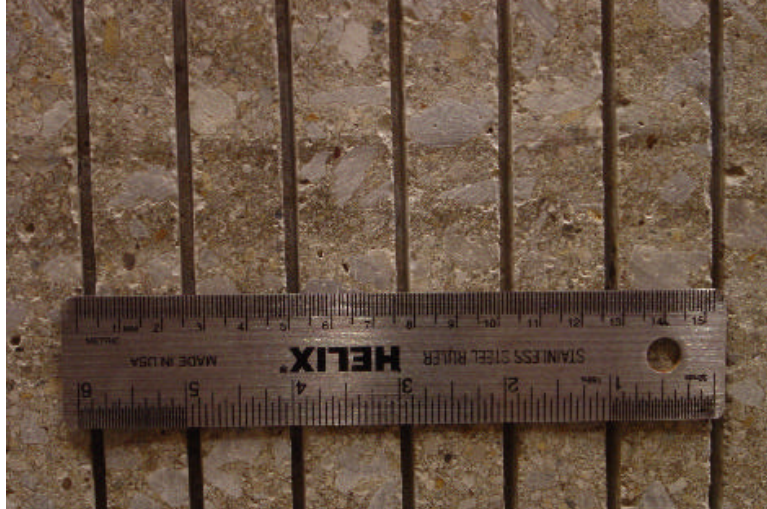
Figure 4.3.9 Ground tines (uniformly spaced at 25 mm)
