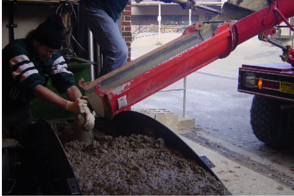
Figure 4.2.5 Casting of the slabs
