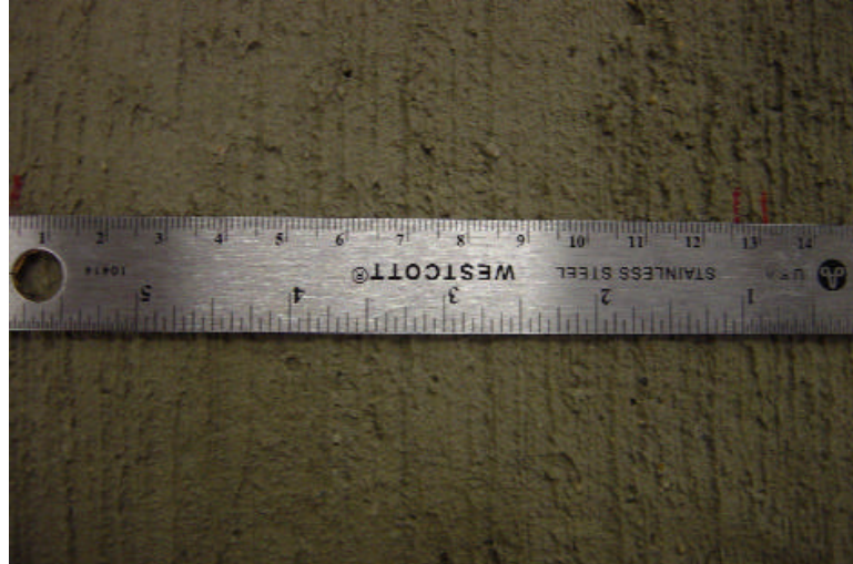
Figure 4.3.5 Broom textured concrete surface
