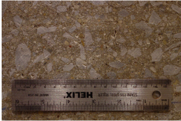
Figure 4.3.3 Grounded concrete surface
