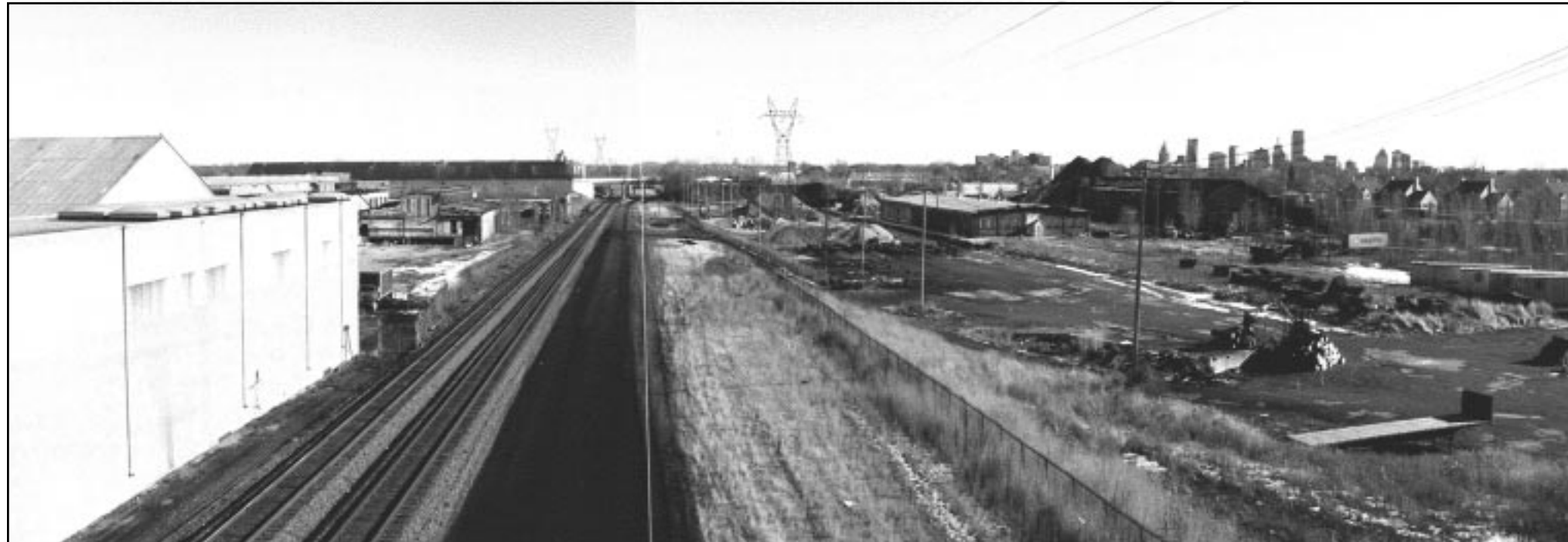
Brownfield site, seen from Dale Street bridge
