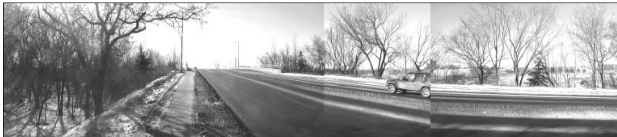
Lexington Avenue crossing, seen from the north
