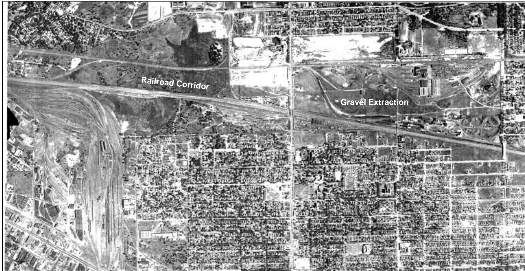
Central Corridor - aerial photo (circa 1940)
