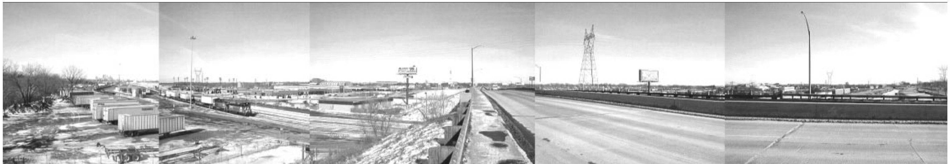
Snelling Avenue crossing, seen from the south
