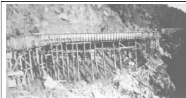
Figure 23. Flume on Colgate system, 1910 (PG&E Archives)
