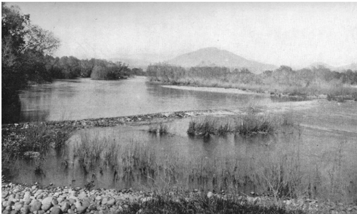
Figure 5. Cobble and brush dam, Fresno Canal, ca. 1898 (Grunsky 1898, Water Supply Paper No. 18:46)
