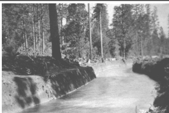
Figure 25. Lower end of Butte Creek Canal in 1908 (PG&E Archives)
