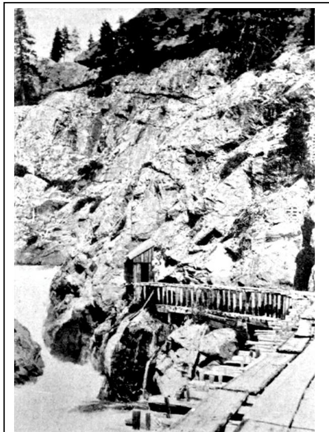
Figure B9. Trestled wood box flume, head of South Yuba Ditch (PG&E Archives)
