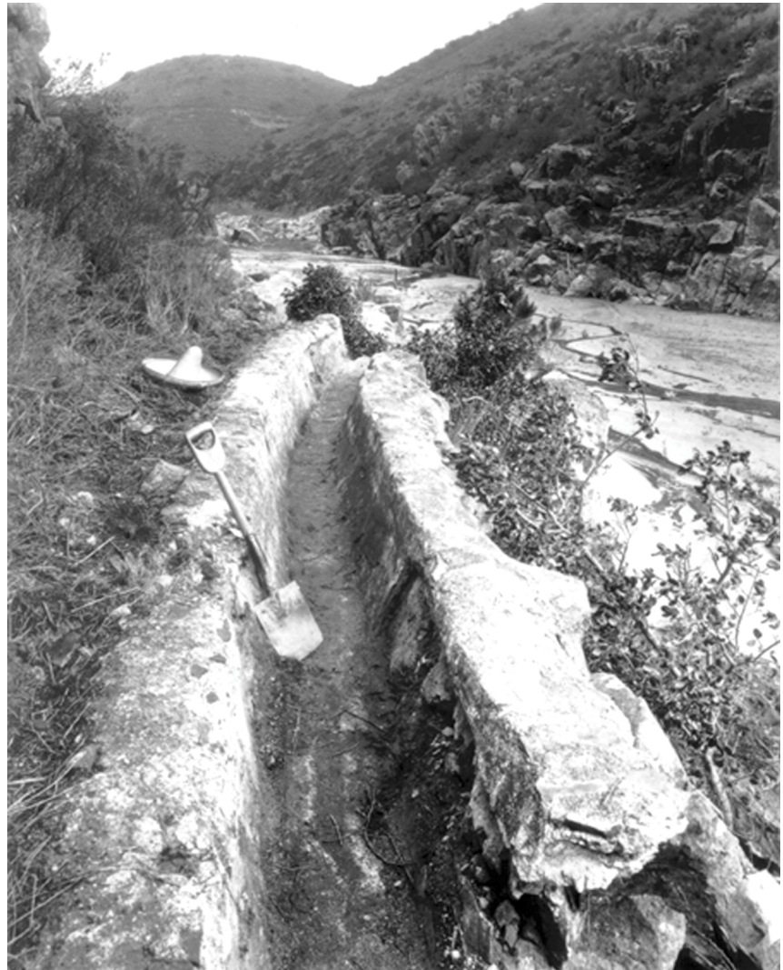
Figure 2. San Diego Mission Aqueduct (California Room, California State Library)
