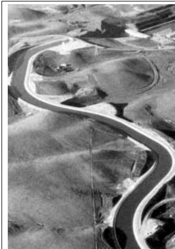
Figure 32. Typical State Water Project canal (DWR, Bulletins 132-193, 1994: cover)
