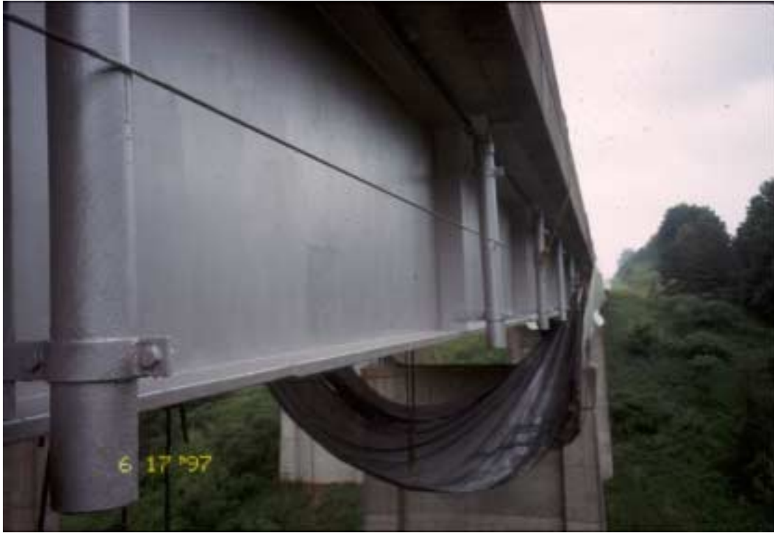
Figure 54. Containment structure during painting operation on I-75.
