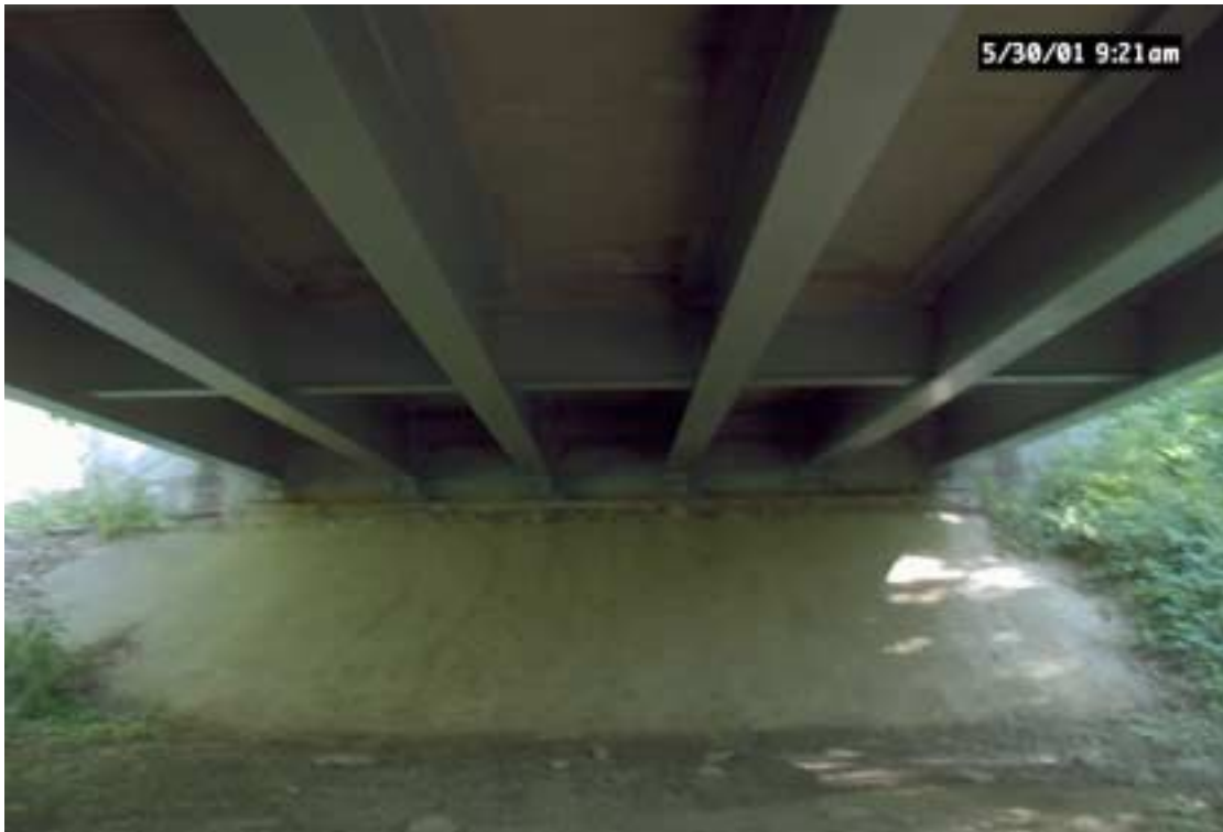
Figure 17. View of abutment and rockers in 2001.
