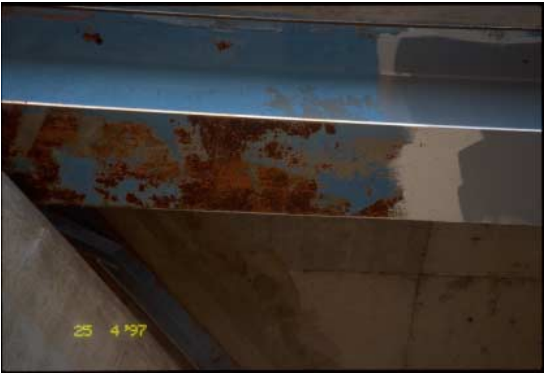
Figure 31. Bridge over I-64 after surface preparation.
