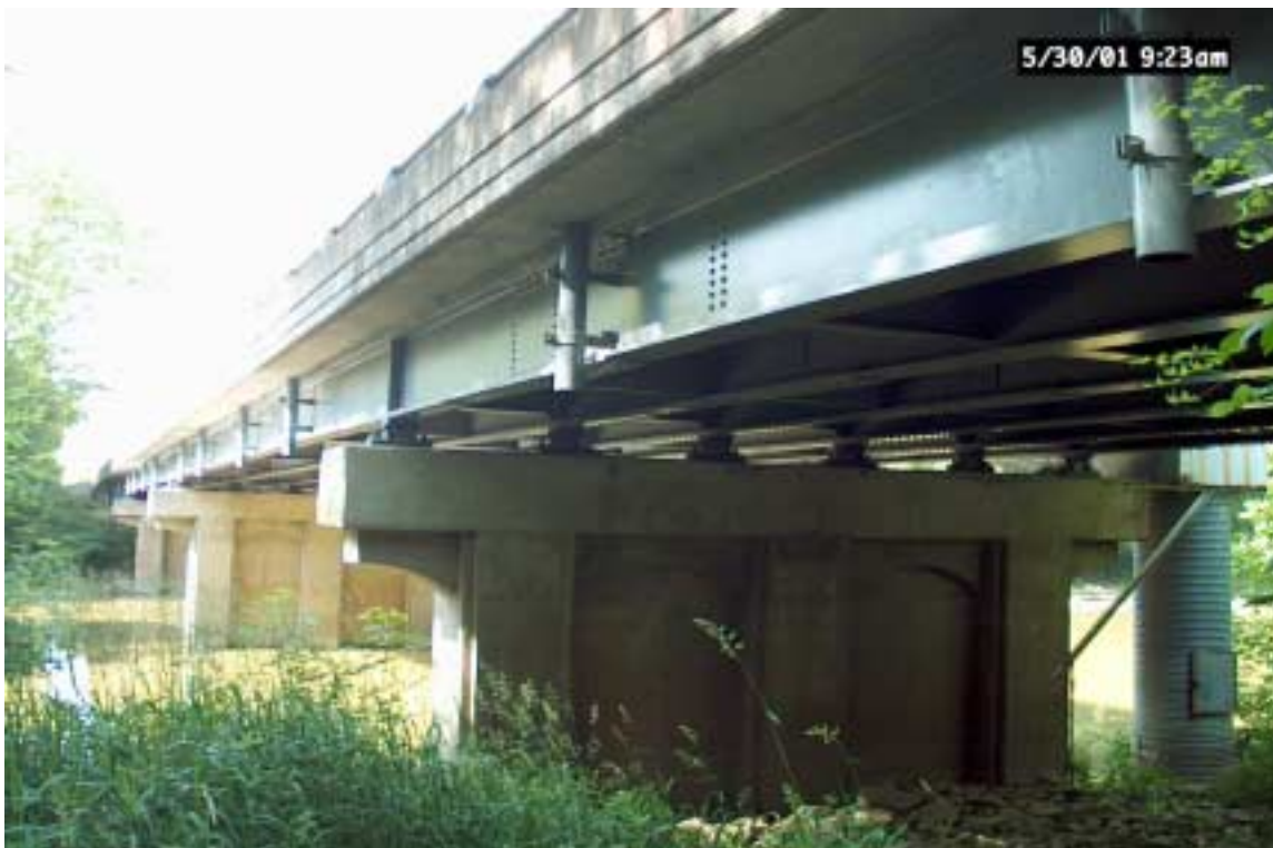
Figure 20. Current condition of the bridge in 2001.
