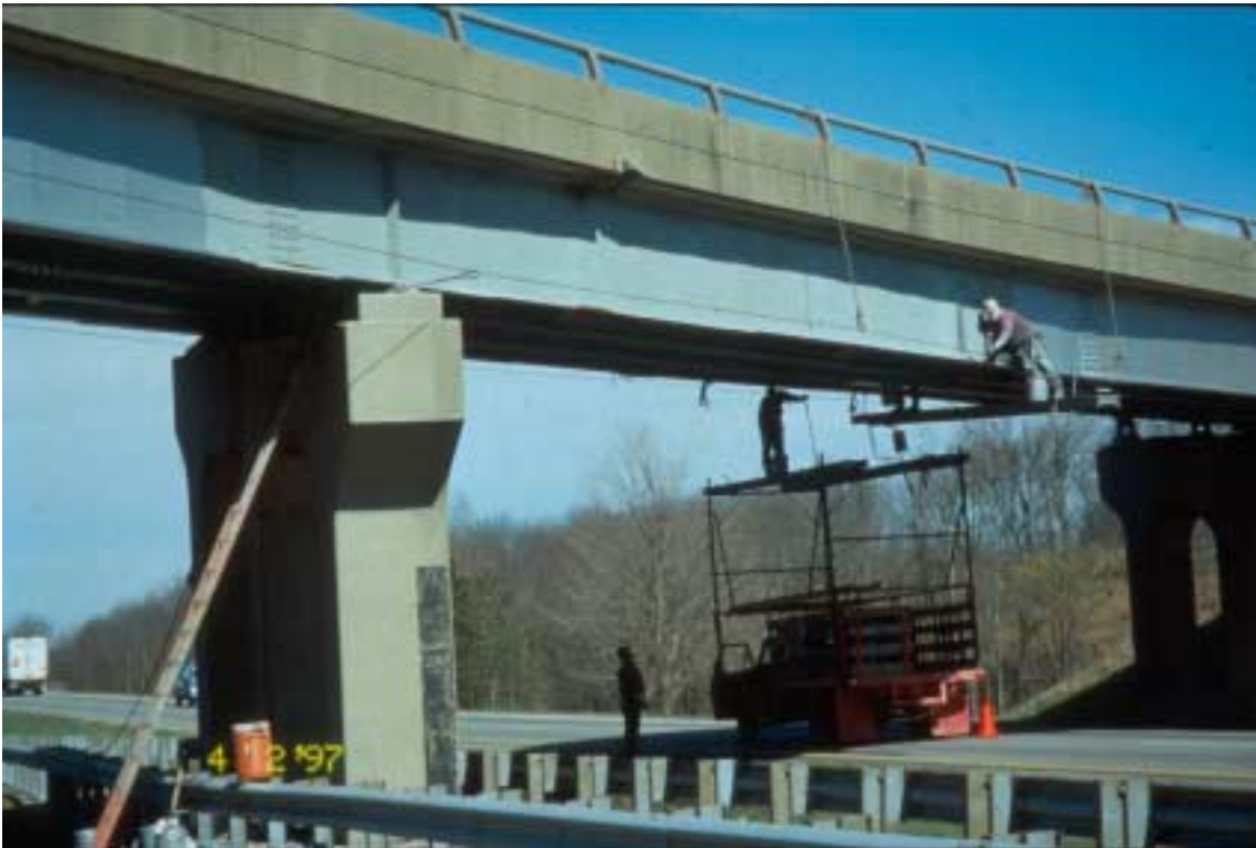
Figure 35. Contractor painting the Mountain Parkway overpass on I-64.
