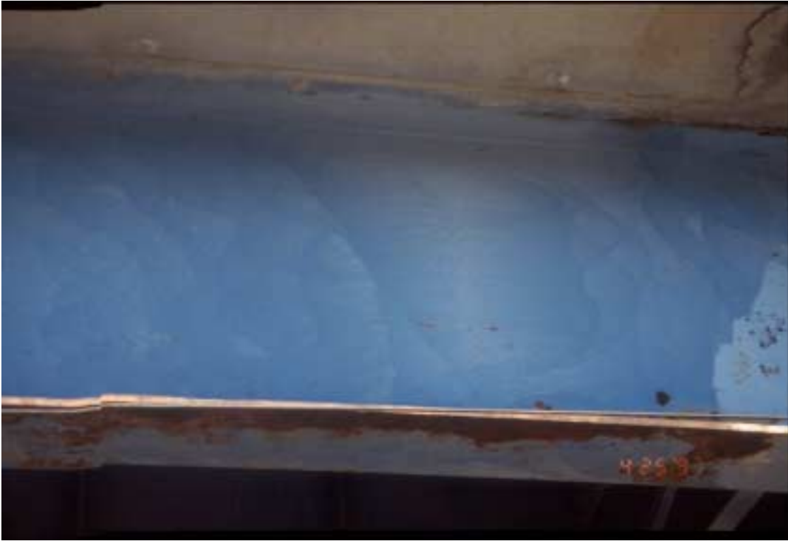
Figure 30. Bridge over I-64 after pressure washing.
