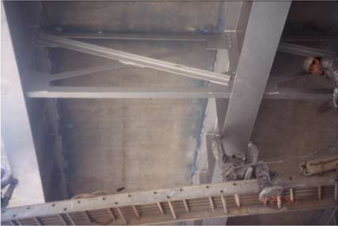
Figure 32. Bridge over I-64 during painting operation.
