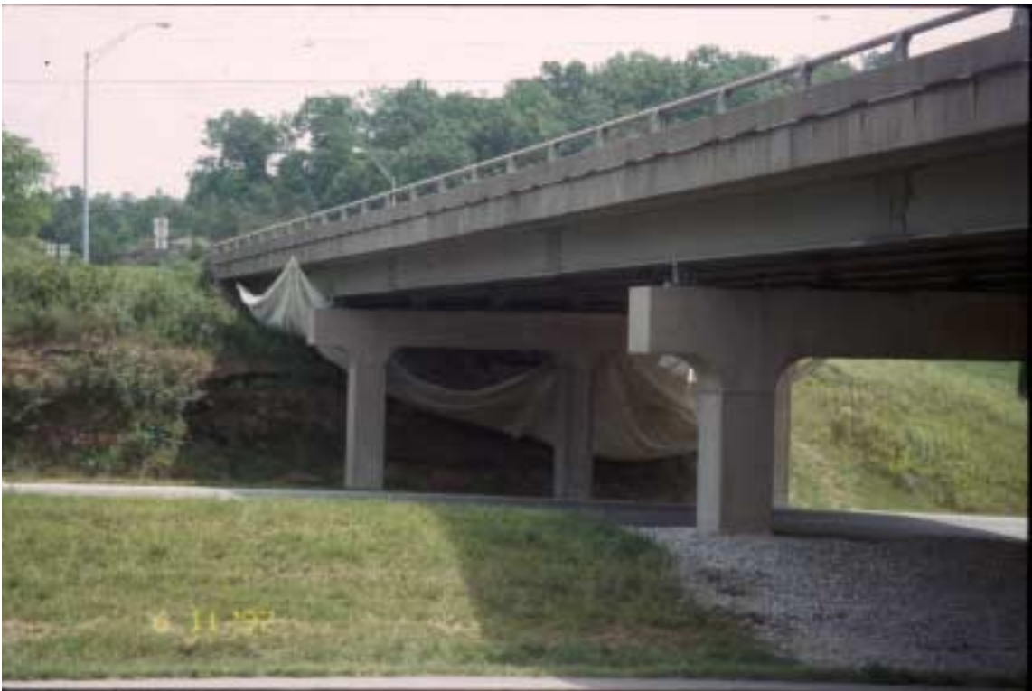
Figure 33. Containment of an overpass bridge on I-64.
