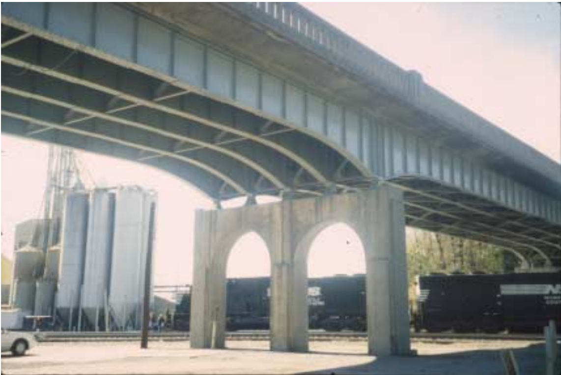
Figure 27. Condition of the bridge after it was painted.
