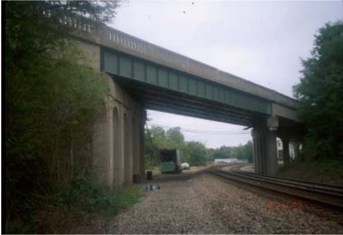
Figure 10. Looking at US 25 bridge over Southern Railroad in Grant County.
