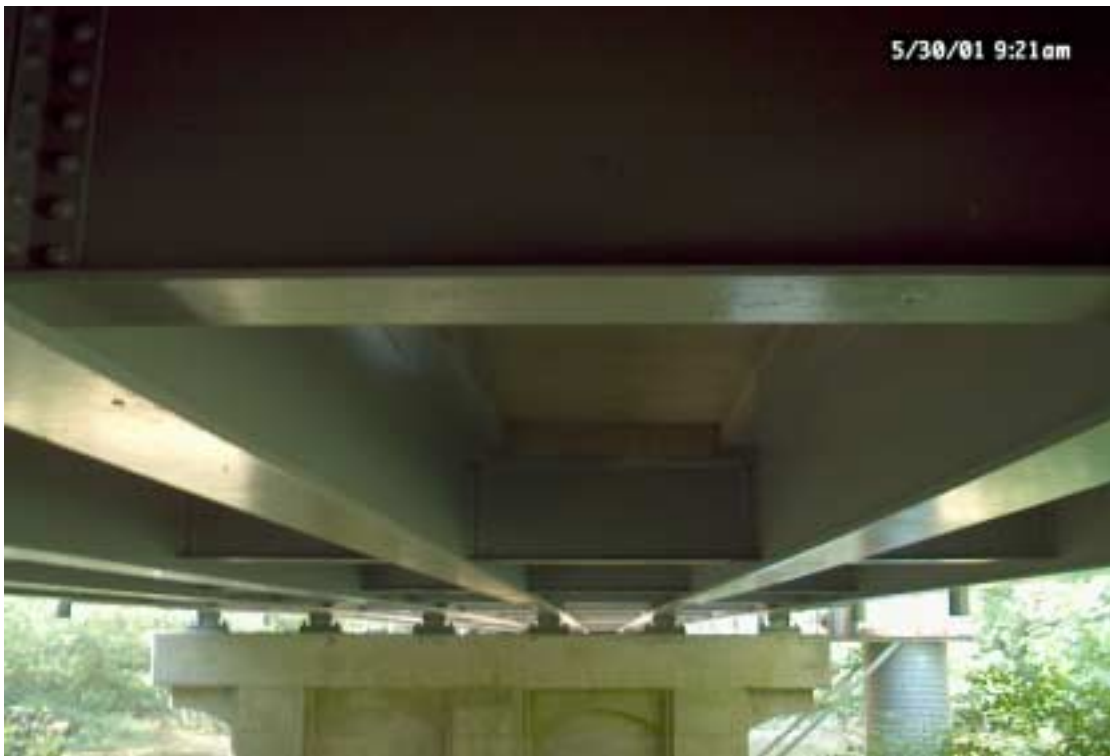
Figure 18. Current condition of the bridge during follow up inspection in 2001.
