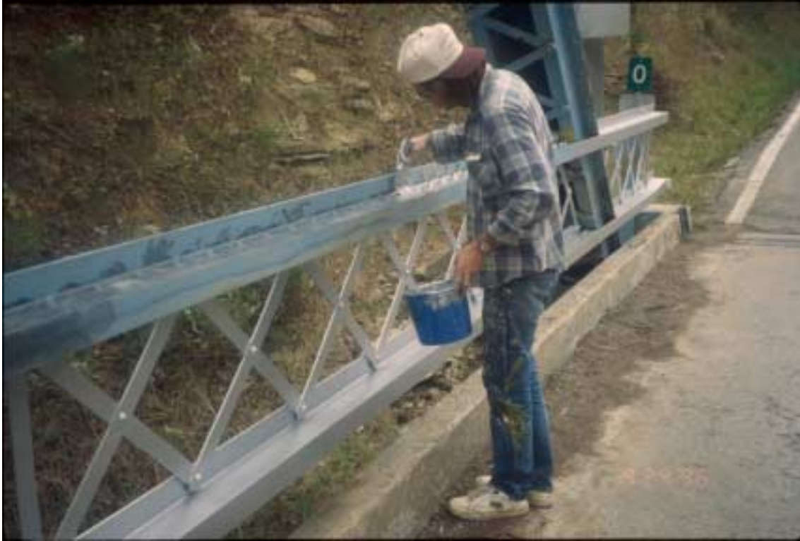
Figure 4. Painting the guard rail steel.
