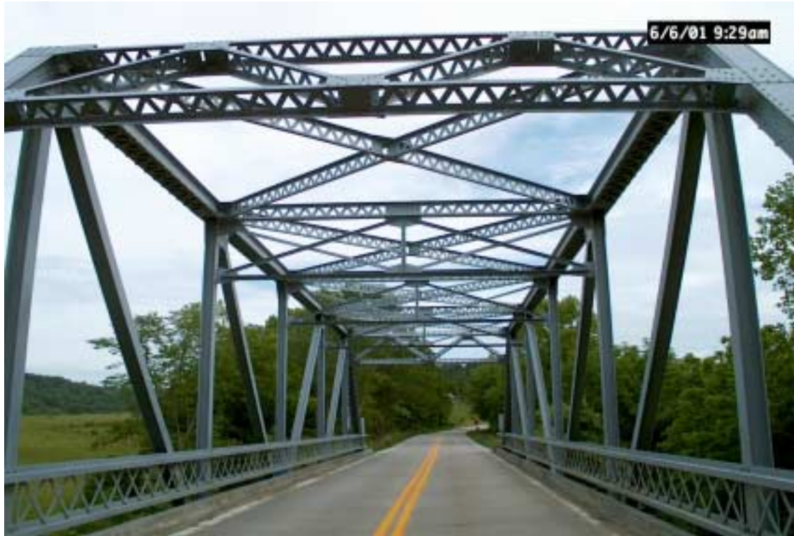
Figure 8. Current condition of truss of the bridge on June 6, 2001.
