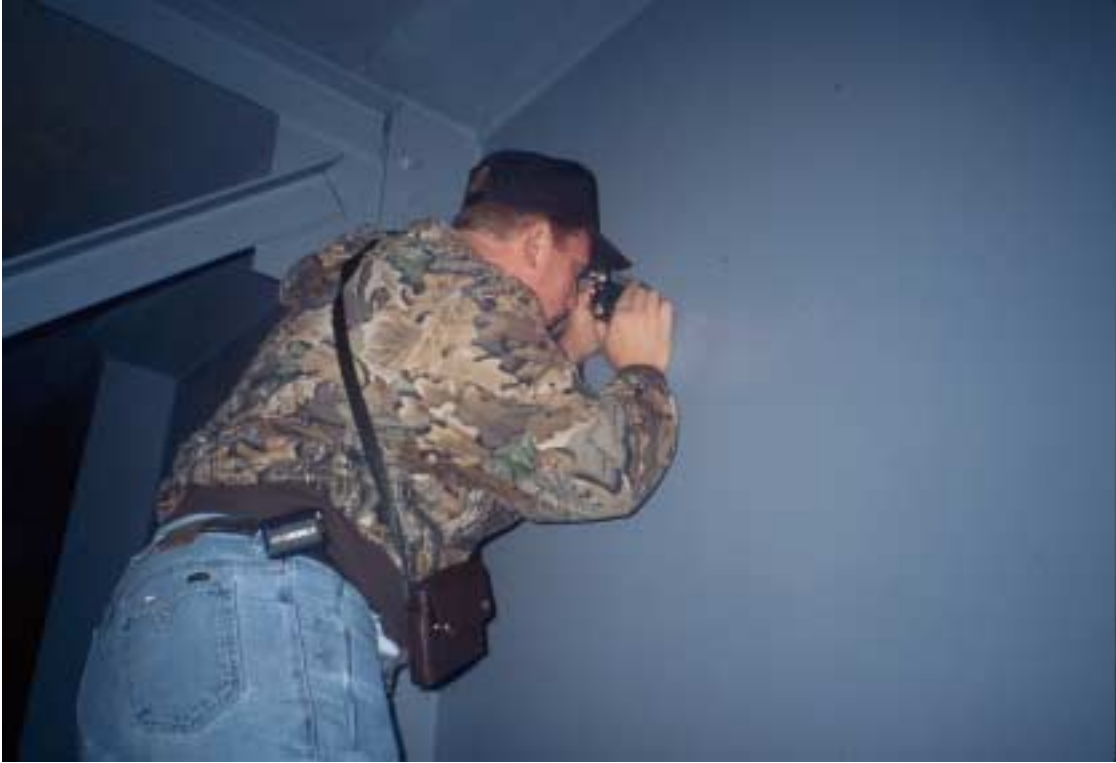
Figure 48. Coating thickness measurement using a tooke gauge.
