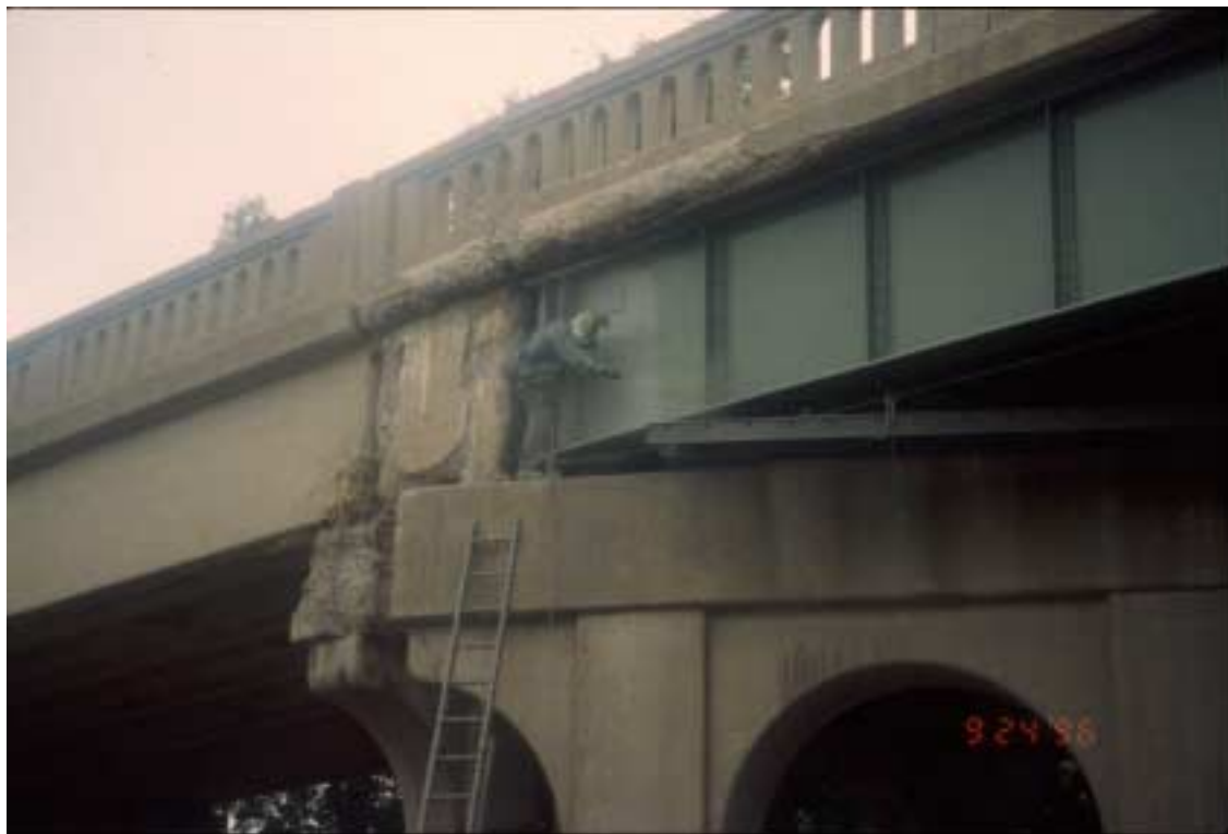
Figure 13. Side view of the bridge being painted in 1996.
