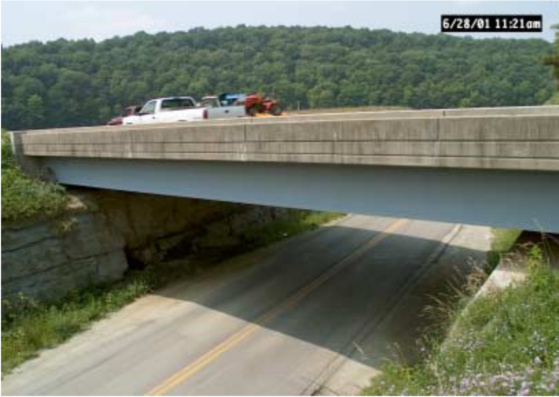
Figure 58. I-75 over Green Hill Road in Rockcastle County.
