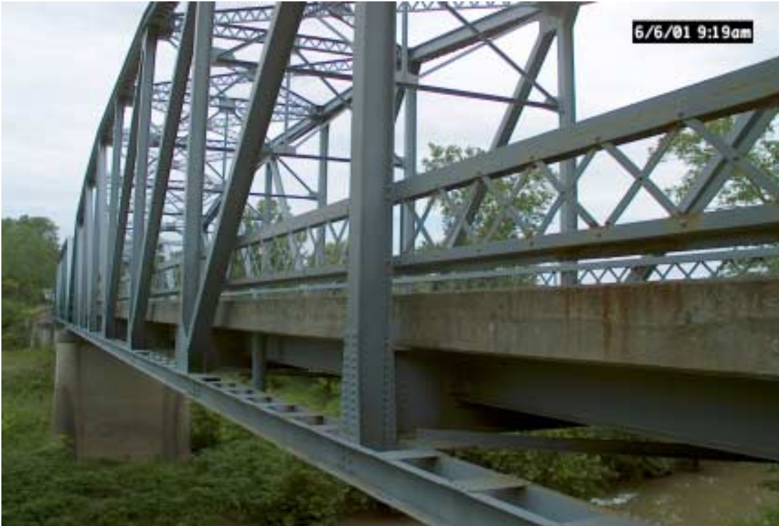
Figure 7. Current status of the Clark County Bridge during follow-up inspection in 2001.
