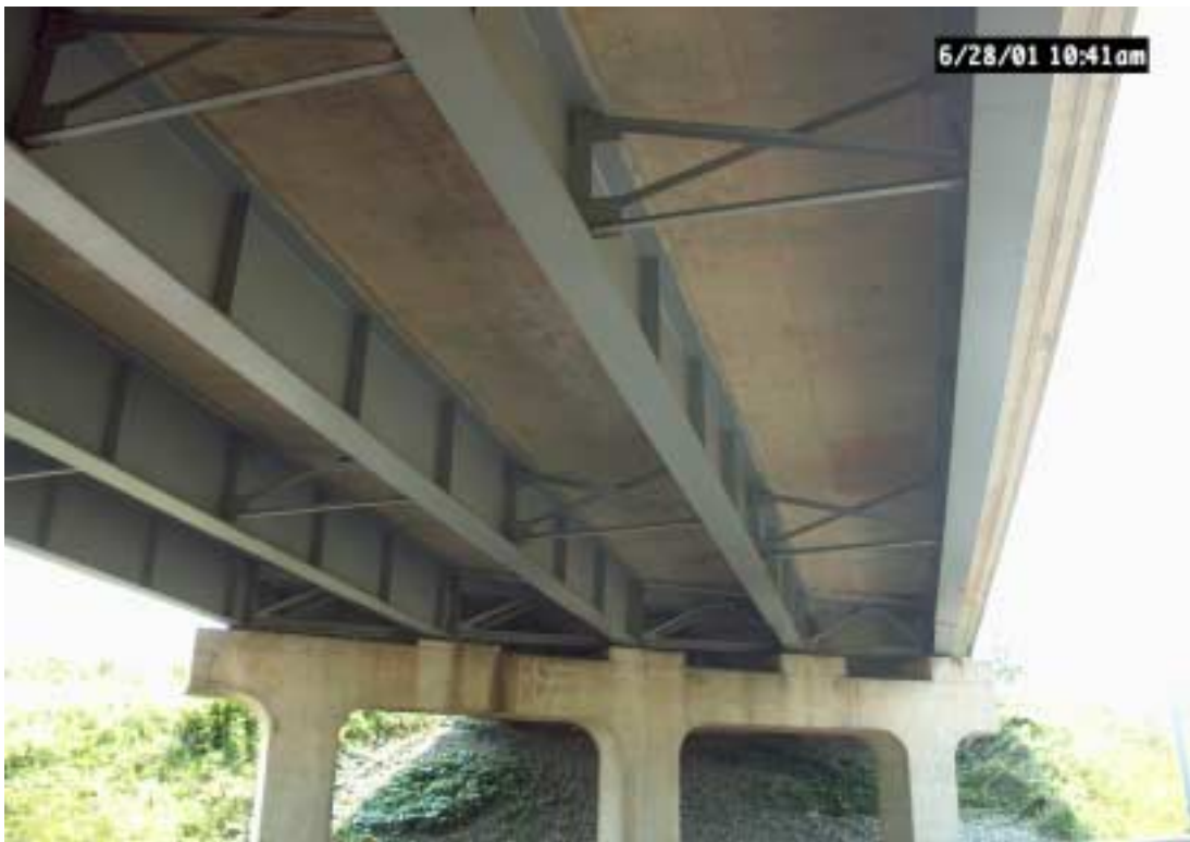
Figure 57. I-75 over US 25 in Rockcastle County.
