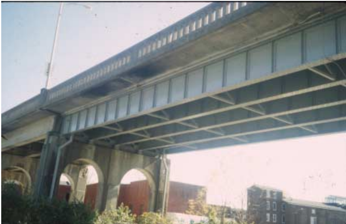
Figure 25. Condition of Bridge prior to painting.
