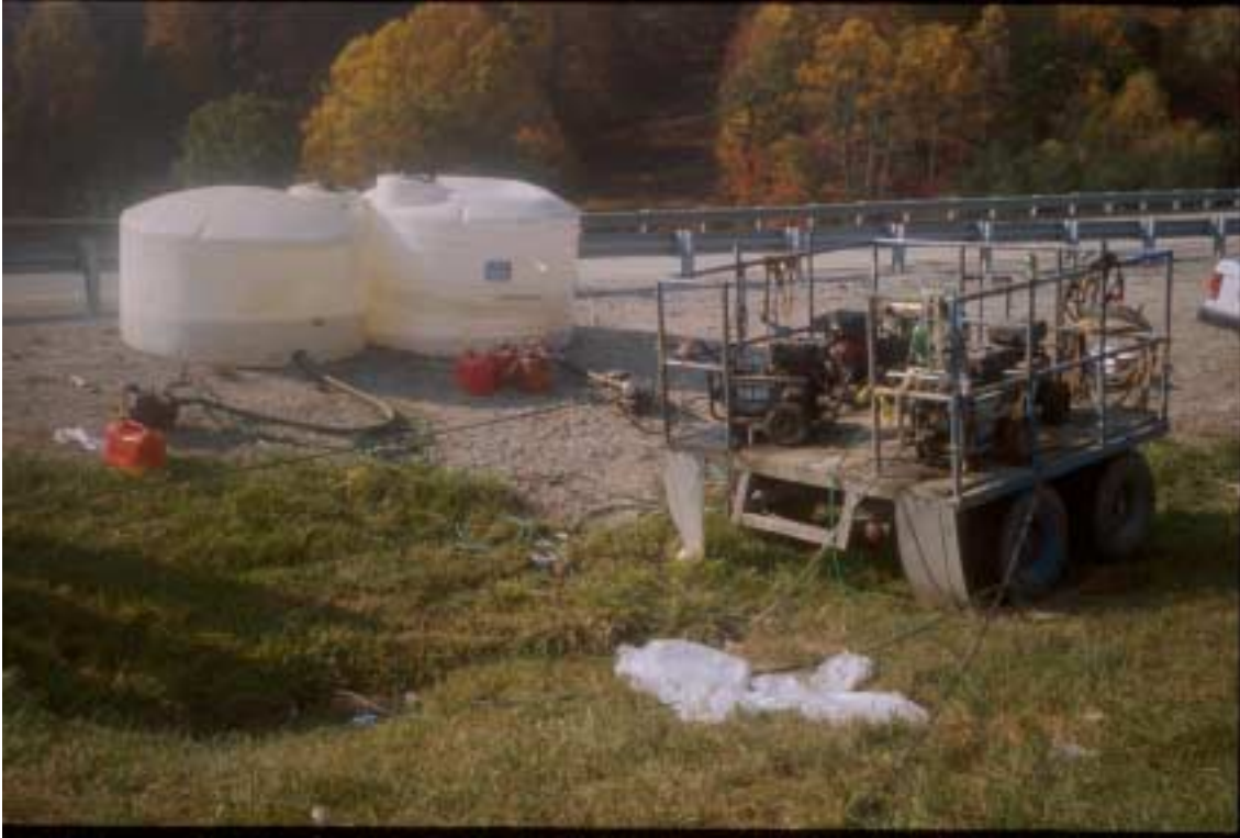
Figure 44. Water tanks and pressure washers used in painting an I-64 bridge.
