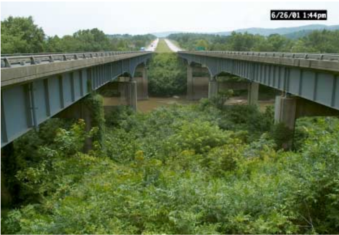
Figure 52. I-75 over Cumberland River and Croley Road in Whitley County.
