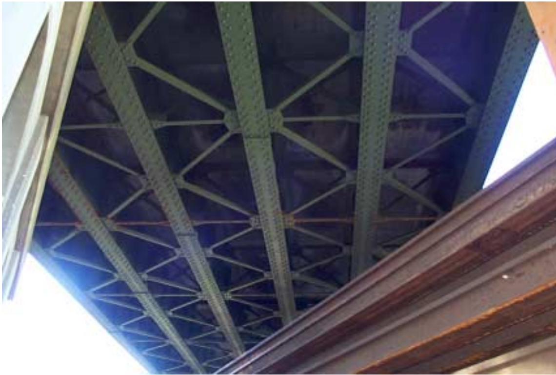
Figure 14. Follow up inspection of the bridge in 2001.
