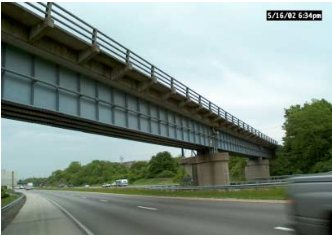
Figure 47. CSX Railroad bridge over I-64.
