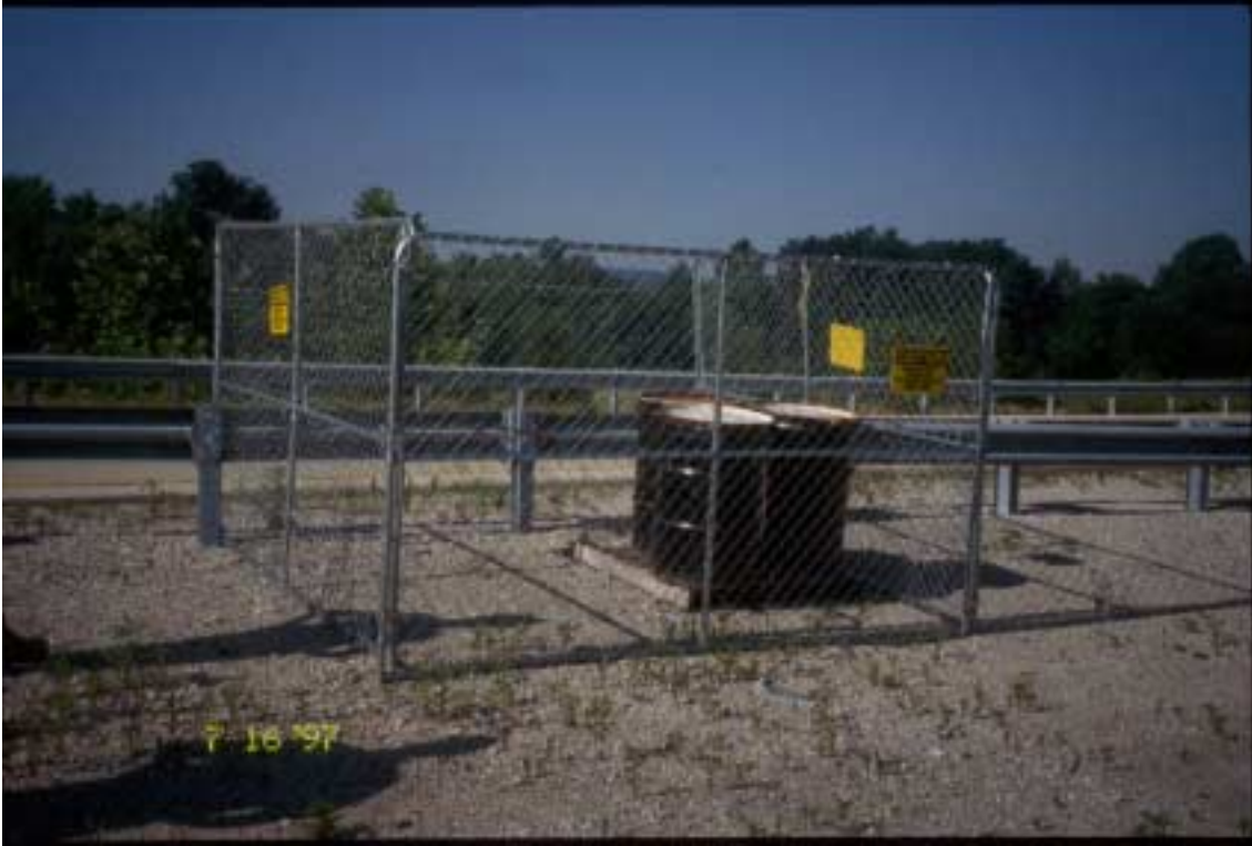
Figure 34. Improper storage of hazardous waste (Using guard rail).
