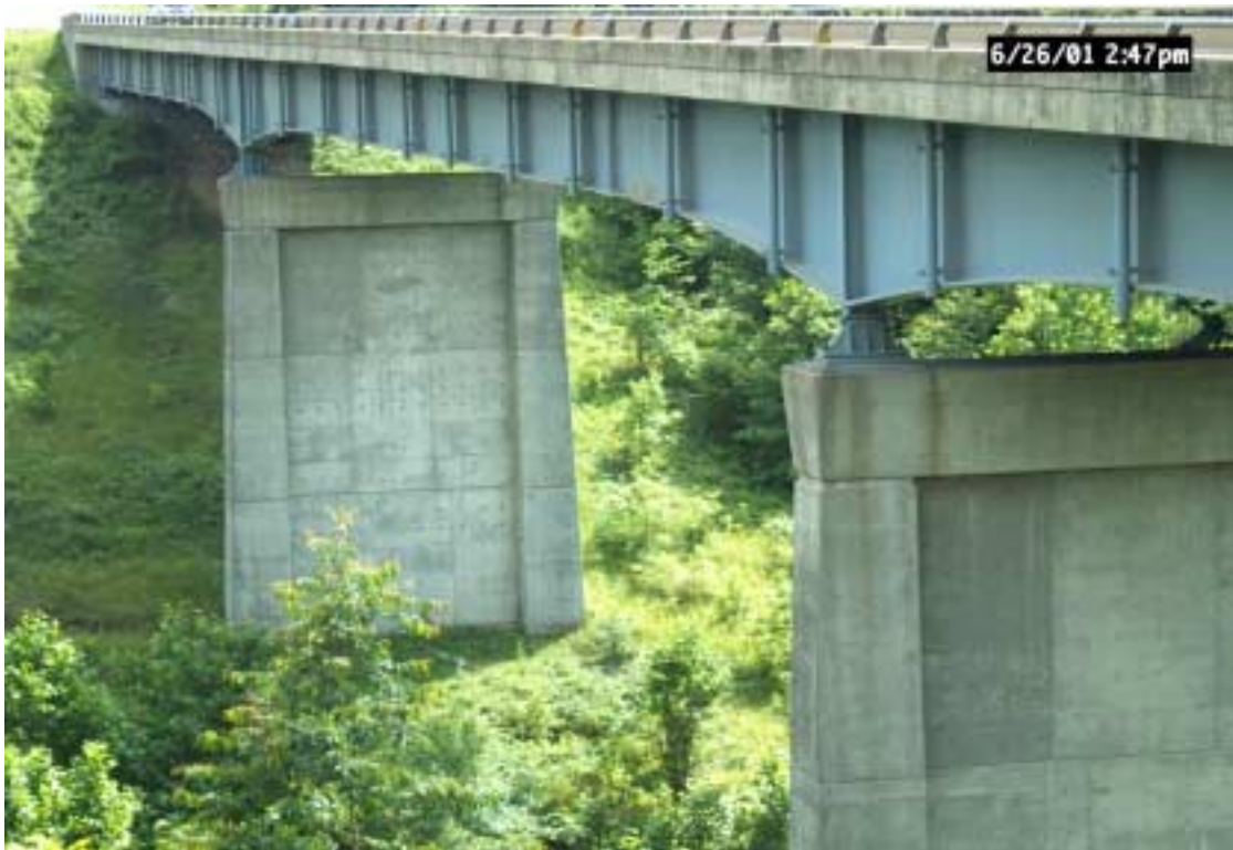
Figure 55. I-75 over Laurel River in Laurel County.
