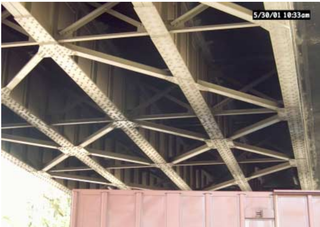
Figure 29. Condition of bridge in 2001.
