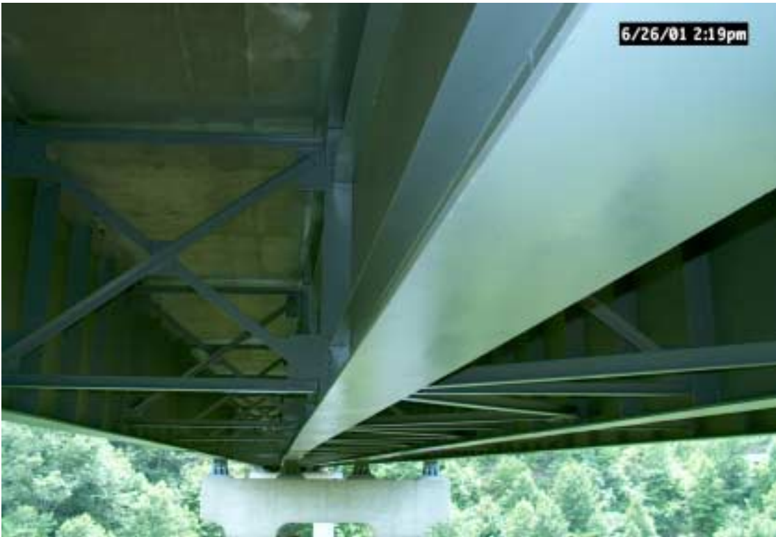
Figure 53. I-75 over Lynn Camp Creek on Laurel-Whitley County.
