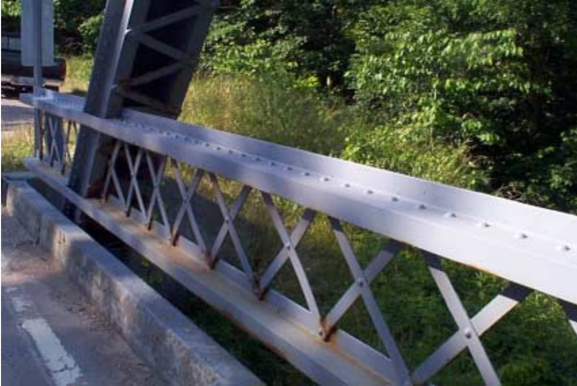
Figure 6. Side view of the cross bracing.
