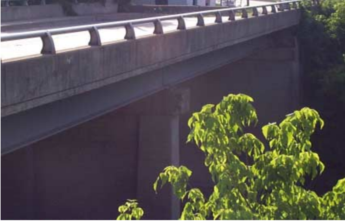
Figure 23. Condition of the bridge in 2001.
