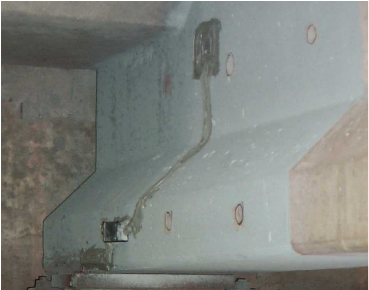
Photo 6. Plate and wire covered with epoxy.
