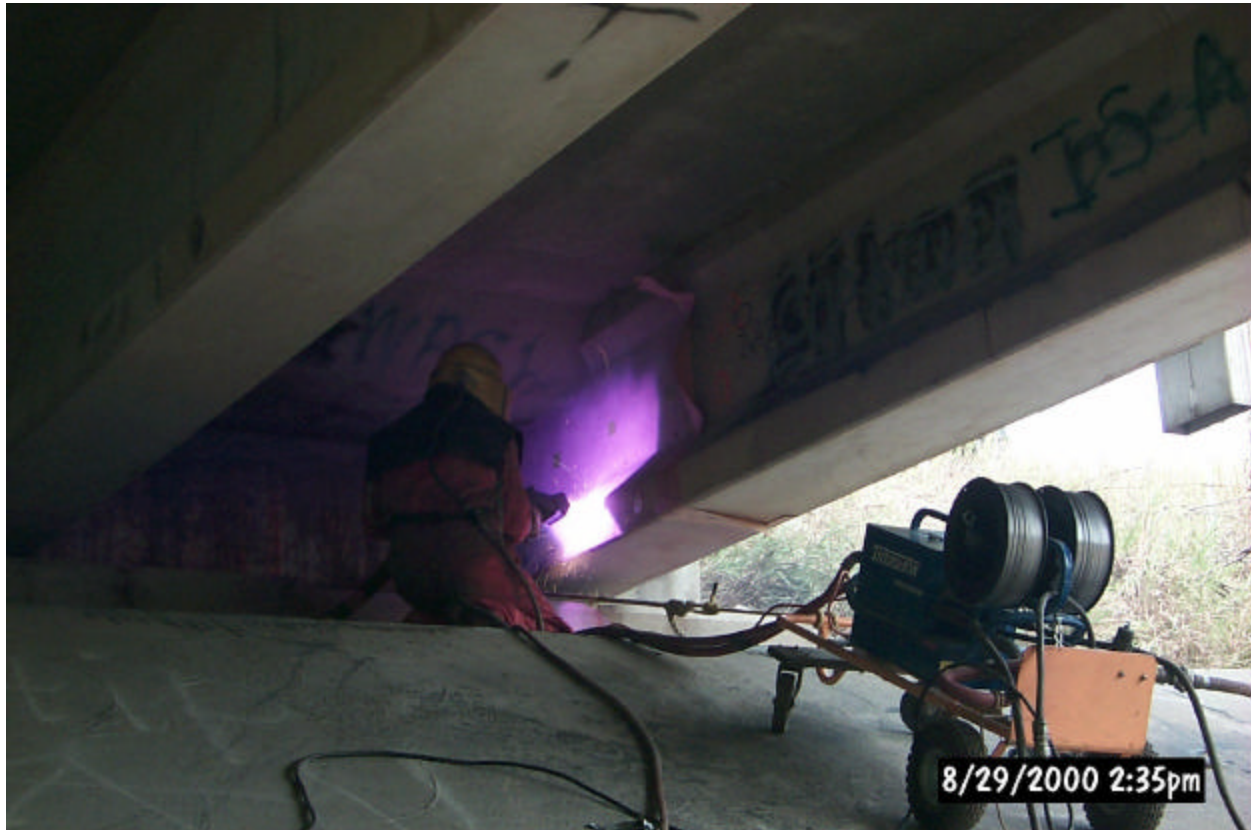
Photo 4. Metallizing beam #6 with Zn/Al/In anode.
