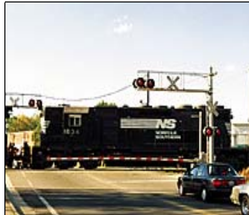
Figure 6. Long Arm Gate at Orr Road, Phase I
