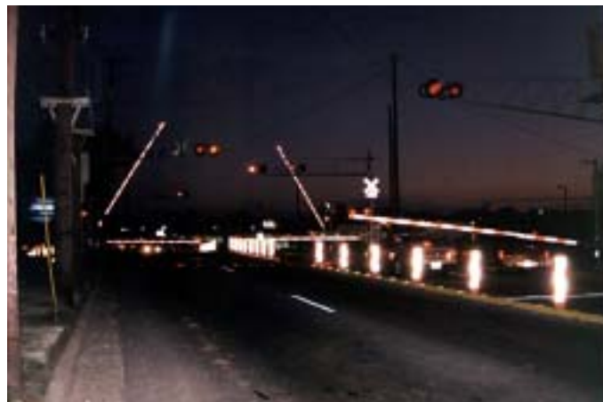
Figure 9. Sugar Creek Crossing with 4 Quad Gates and Traffic Channelization Devices at Night
