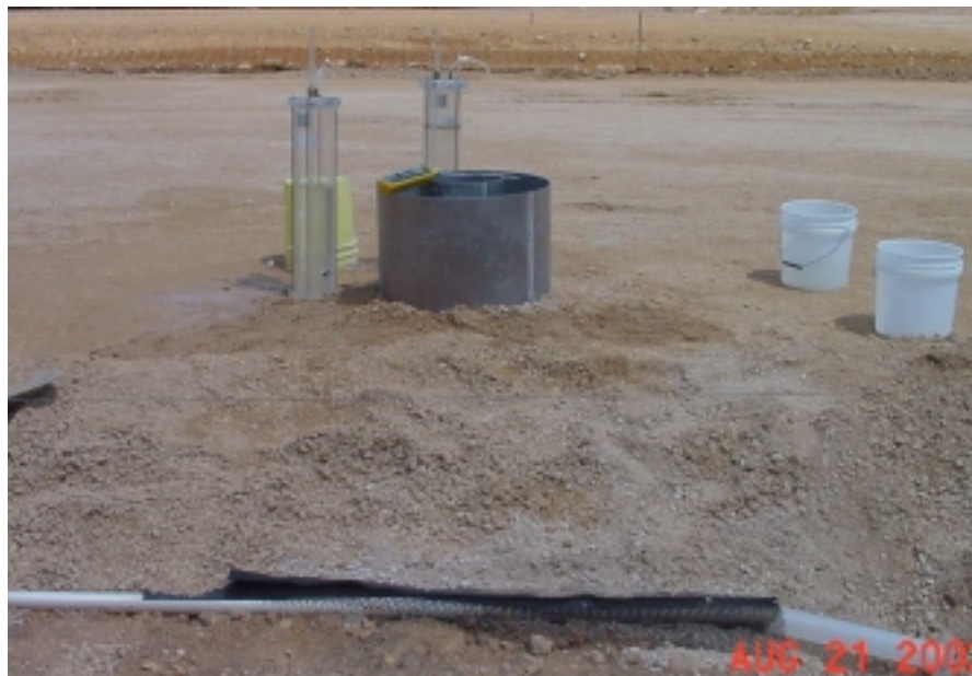
Figure 13 Field setup of underdrain lysimeter and double ring infiltrometer.
