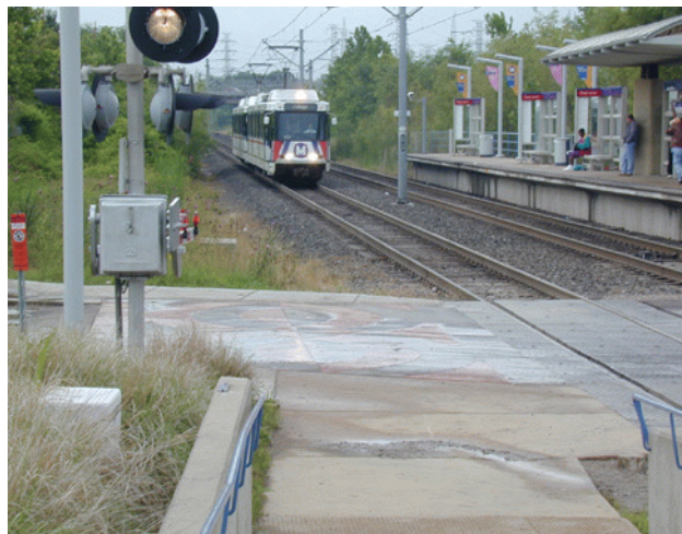
The rail platform is elevated, but accessible to all by ramp.
