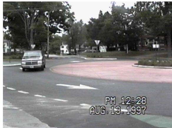
Figure 4 The Gorham, Maine, roundabout constructed in 1997
