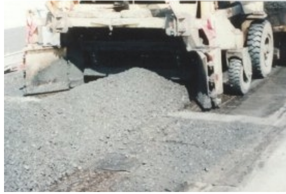
Figure 11 The pickup machines were kept raised to prevent damage to the fabric.
