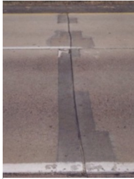
Figure 4 Joint 685 after minimum rehabilitation and prior to the asphalt overlay.
