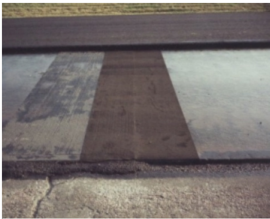
Figure 12 Linq Tac-711N with passing lane overlaid with asphalt.
