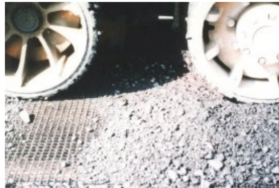
Figure 9 A thin layer of spread used to avoid pulling and stretching from the tires.
