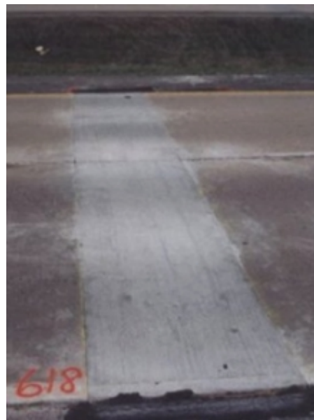
Figure 2 Joint 618 after maximum rehabilitation and prior to the asphalt overlay.
