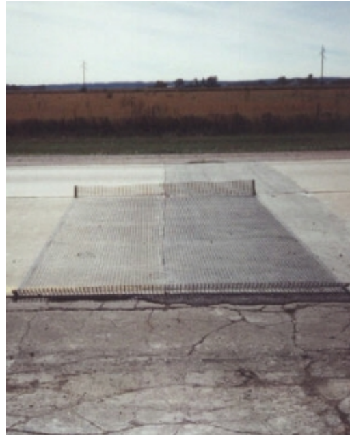
Figure 7 Strata Grid-200 installed and ready for the asphalt overlay.
