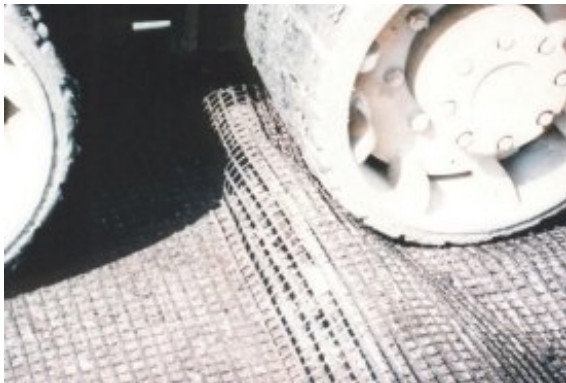
Figure 8 Strata Grid-200 bubbling under the tires of a truck.
