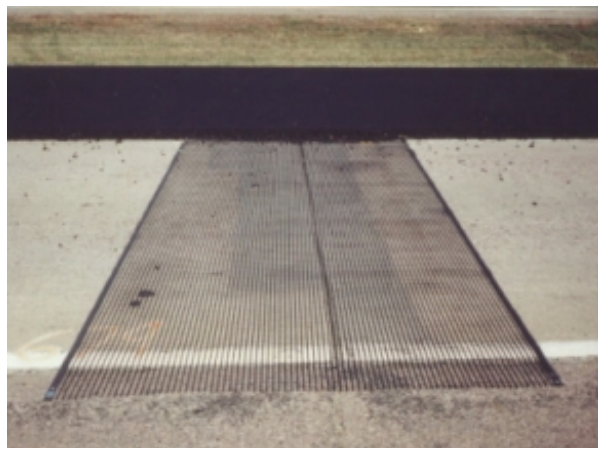
Figure 13 Strata Grid-200 with passing lane overlaid with asphalt.
