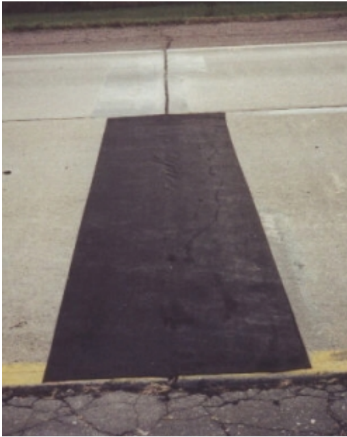
Figure 6 Linq Tac-711N installed and ready for the asphalt overlay.
