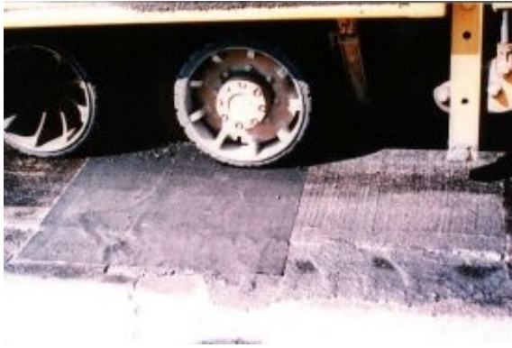
Figure 10 Linq Tac-711N under construction with no pulling or shoving.
