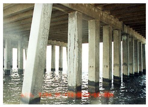
Figure 2.11 - Face Splitting of a Bridge Column in Corpus Christi
