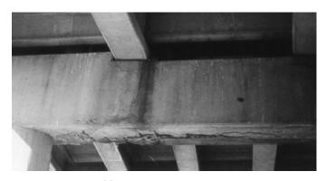
(c) Bent Cap Corrosion
