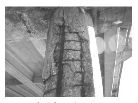
(b) Column Corrosion
