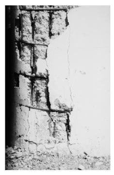
Figure 5.4 - Column Corrosion Resulting from Splashing Adjacent to Roadway
