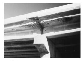
(a) Corrosion at Leaking Deck Joint
