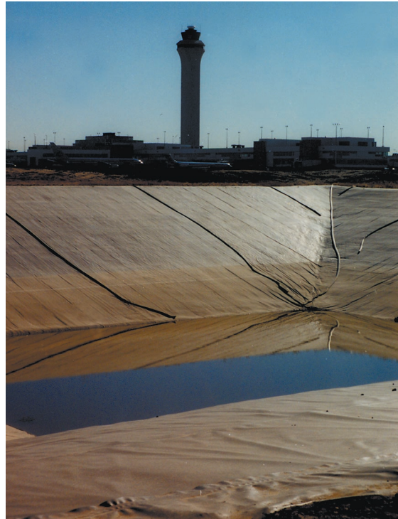
Figure 17: Two Deicing/Anti-Icing Runoff Capture Basins at Denver International Airport
