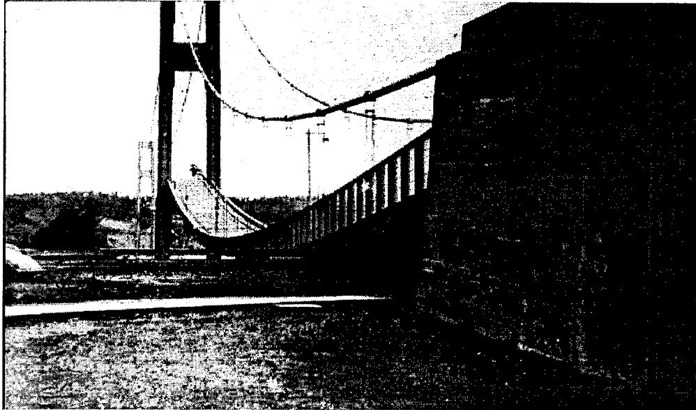
Figure 2.12: This photograph shows the sag in the east span after the failure. With the center span gone there was nothing to counter balance the weight of the side spans. The sag was 45 feet (13.7m). Also the immense size of the anchorage is illustrated.
