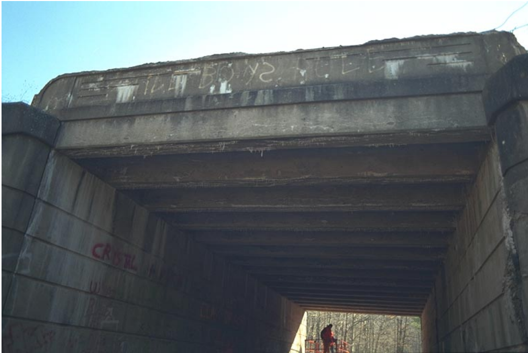
b. Exterior face of north parapet of Bridge 101A.
