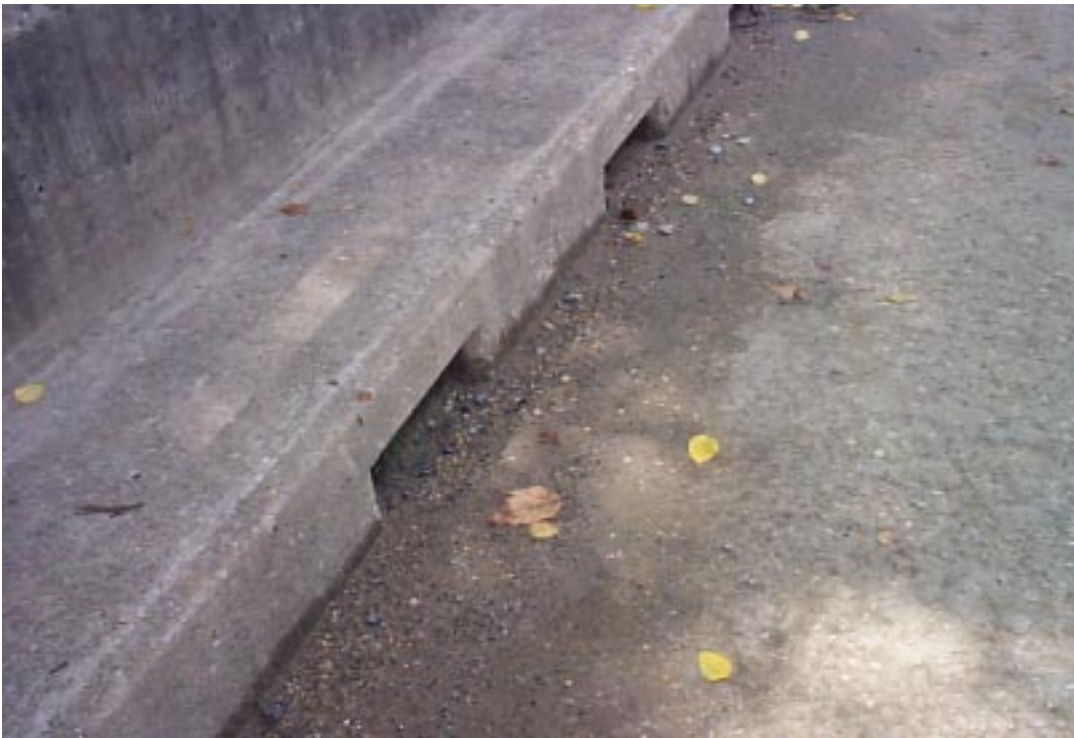
Figure 174. Curb close-up example photograph.
