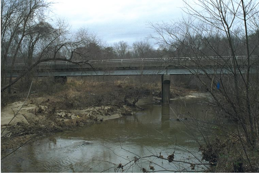
Figure 17. Van Buren Road Bridge.
