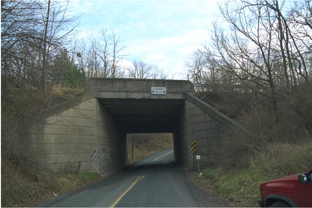
a. Elevation view of Bridge B111A.
