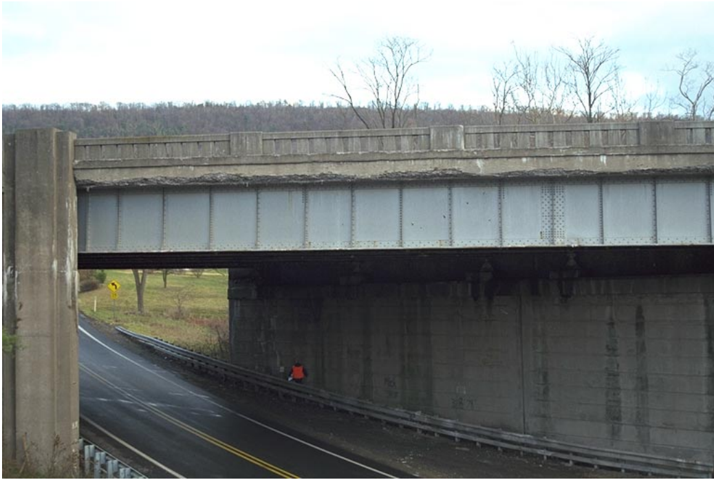
a. Elevation view of Bridge B544.
