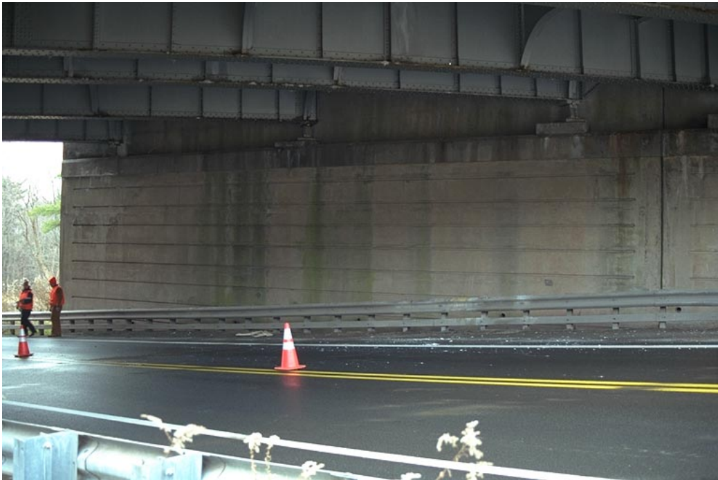
b. Bridge B544 superstructure.
