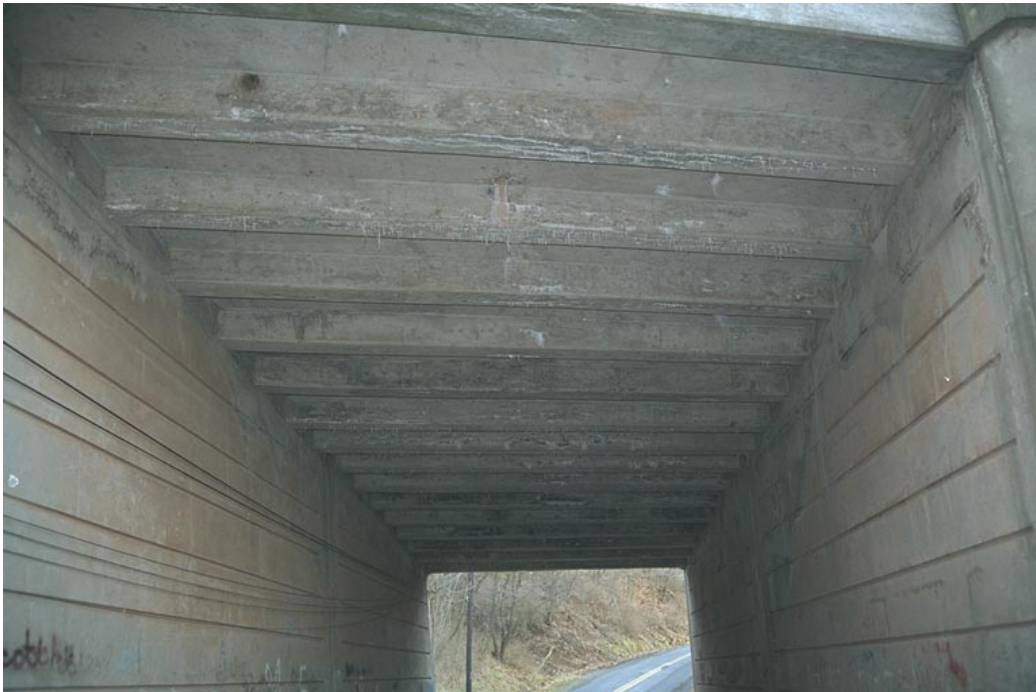
b. Bridge B111A superstructure.
