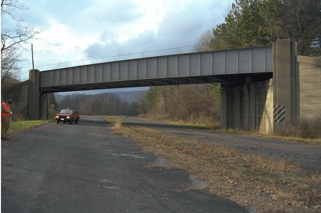
a. Elevation view of Bridge B521.
