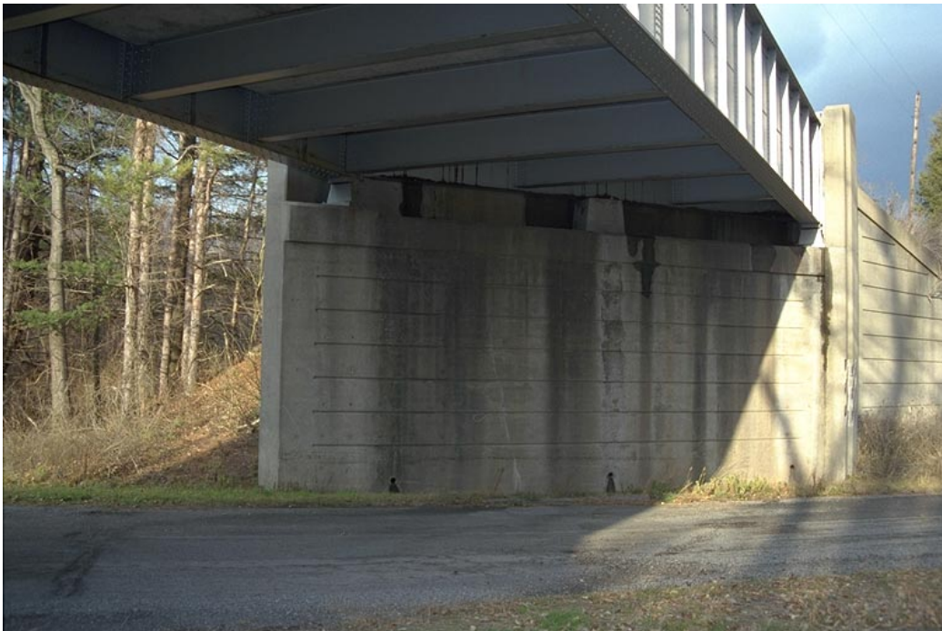
b. Bridge B521 superstructure and abutment.
