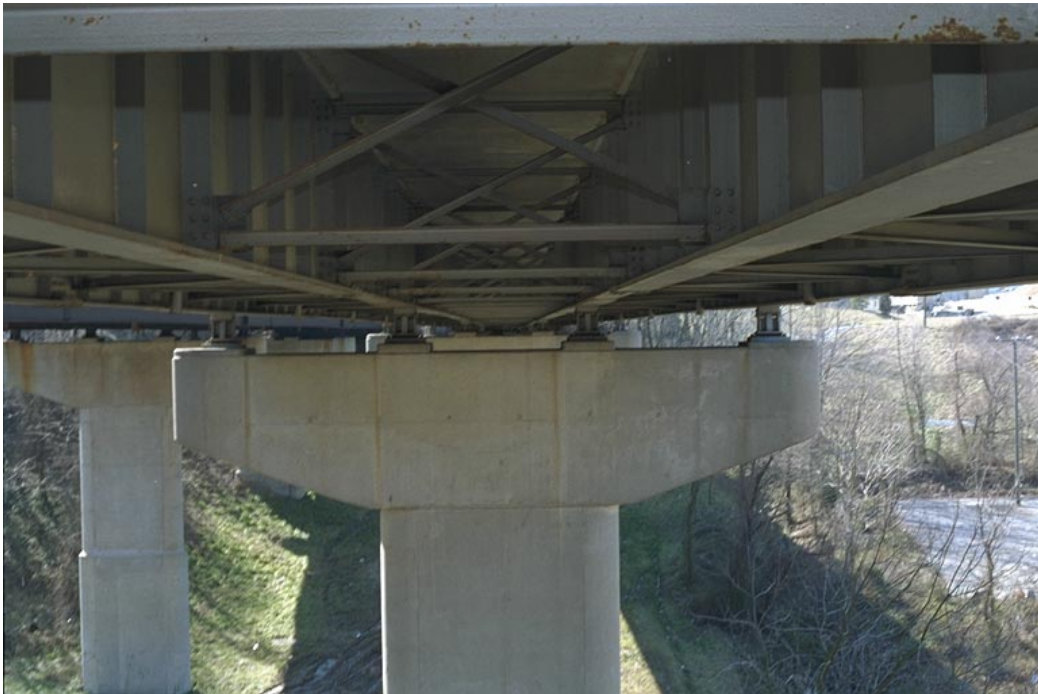
b. View of superstructure.
