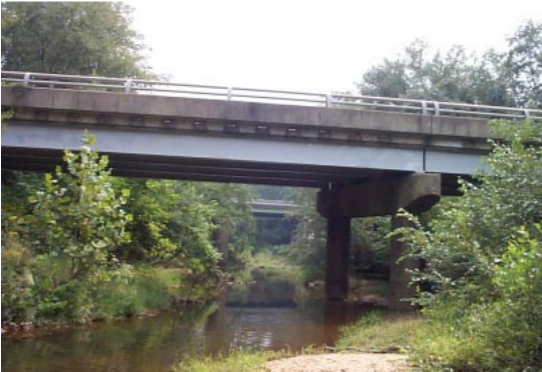
Figure 168. Overall elevation example photograph.
