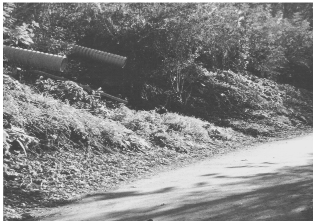
Figure 19 Center Avenue Bridge Drain
